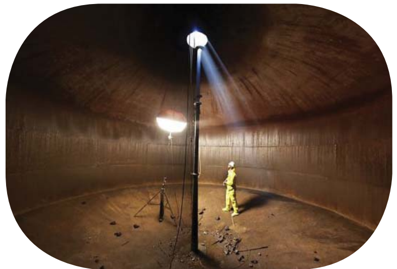
The interior of a cistern. © SFPUC; Robin Scheswohl
