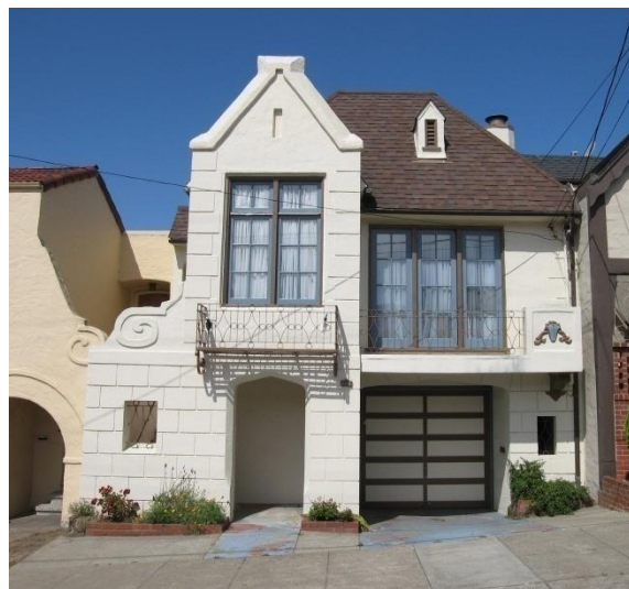
2191 32 nd Avenue, Golden Gate Investment Co., 1933. This house features unusual Period Revival roof forms and detailing not commonly found in the Sunset District.
