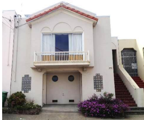
This eclectic house on 21st Avenue displays Art Deco ziggurats (filled with glass block) and porthole garage windows, with Spanish clay tile and arches inspired by Mediterranean Revival design.
