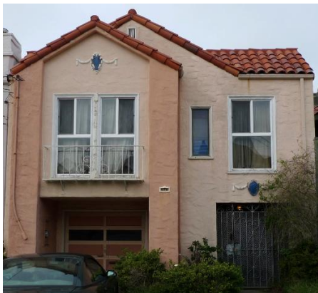
Left: Chris McKeon's temporary personal residence, 2163 29 th Avenue, within the District.
