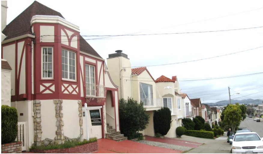
View looking northwest on 31 st Avenue. Source: SF Planning
