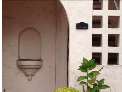
Niche located with an entry alcove.
