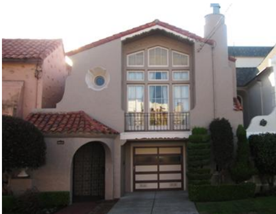
The "Surprise House," 1548 35 th Avenue.
