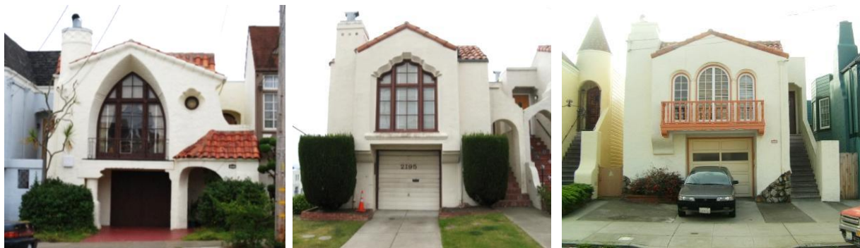
Left: Doelger's 33 rd Avenue tract / 1530 33 rd Avenue Center: Bay Cities Building Company's tract / 2195 30 th Avenue Right: Doelger's 31 st Avenue tract / 1617 31 st Avenue
