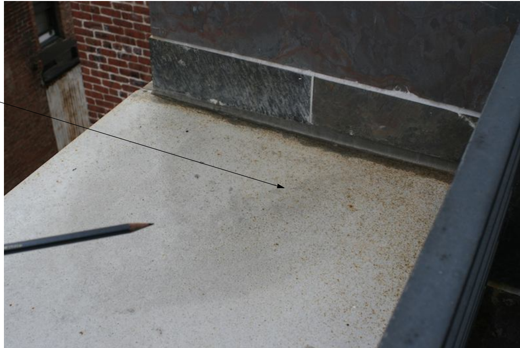
1 - SHEET METAL COPING AT DECK
