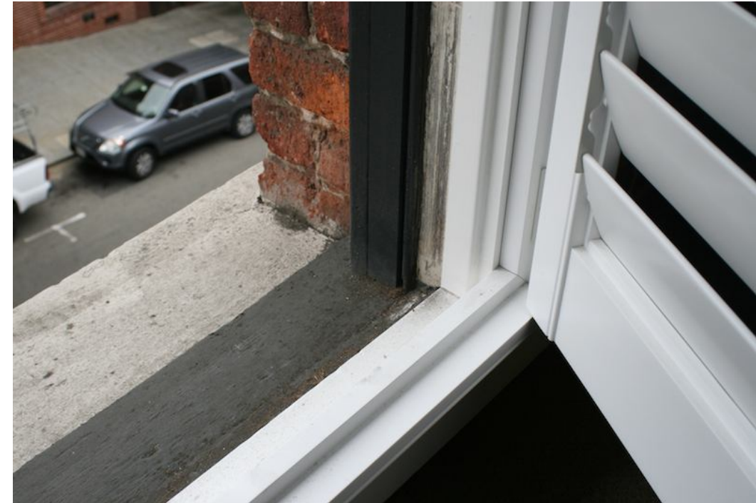
3 - WINDOW ALONG MONTGOMERY ST.
