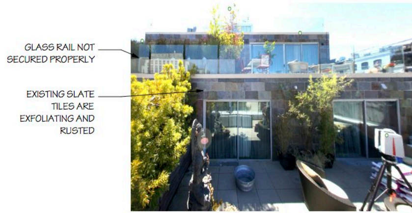
1 - THIRD FLOOR TERRACE VIEW
