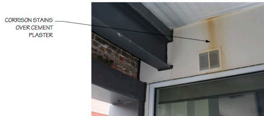
2 - UNDERSIDE OF UNIT DECK
