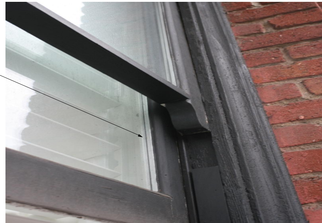
4 - WINDOW ALONG MONTGOMERY ST.
