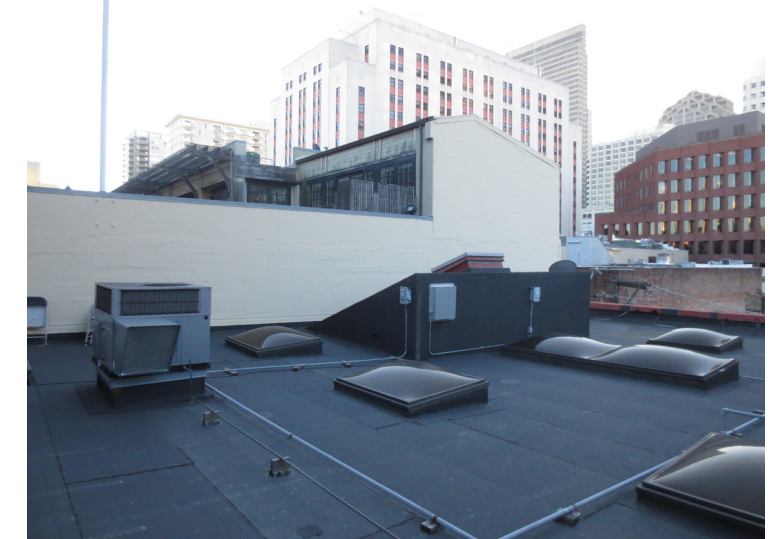
view looking southeast towards 40 Gold (Black Board) existing roof terrace on adjacent building
