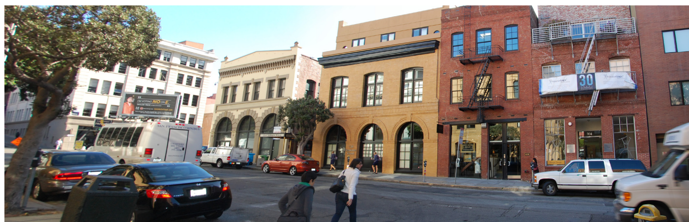
Sansome Street - Looking East previous vertical additions
