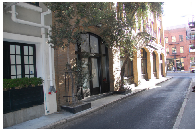
40 Gold Street & 727 Sansome Street general character, rowlock brick, punched openings
