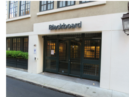
5 View of Context - East
