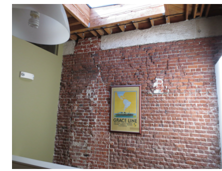
10 View of Existing Interior - Second Floor Office
