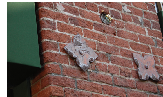
Decorative wall ties and abandoned electrical
