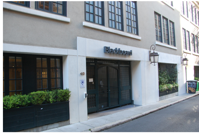
40 Gold adjacent building, punched openings
