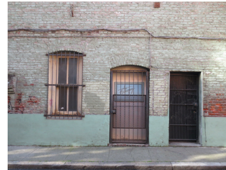
4 View of Context - Across Gold St.
