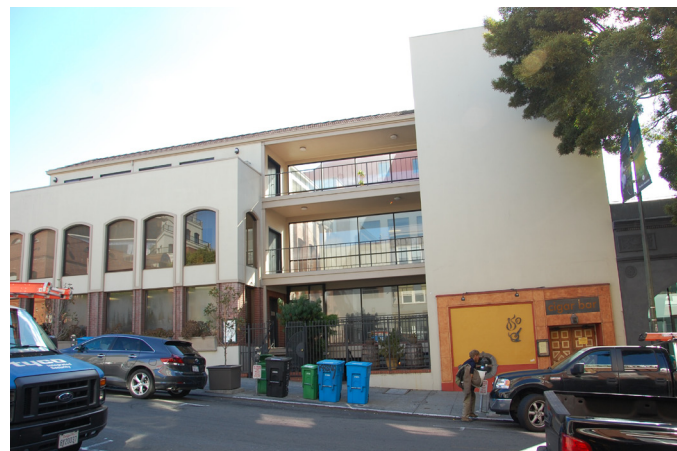
850 Montgomery mix of contemporary buildings in the district
