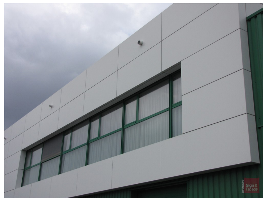
Proposed metal panel system. Example photo of deeply recessed windows, corners and joint module
