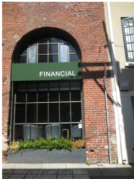
6 View of Existing Window Bay
