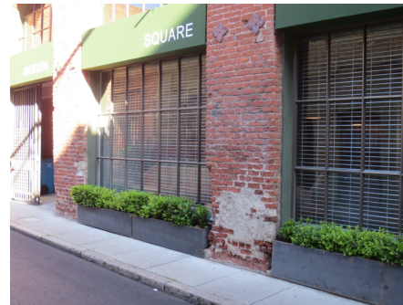
3 View of Existing Brick
