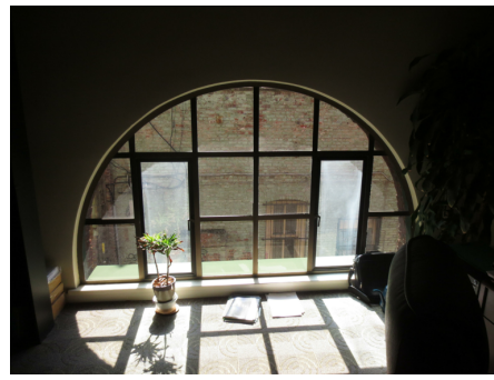
9 View of Existing Interior - Second Floor Office
