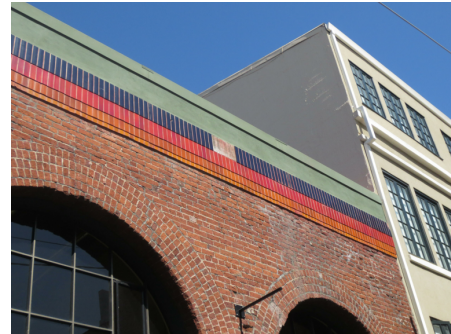
2 View of Existing Parapet
