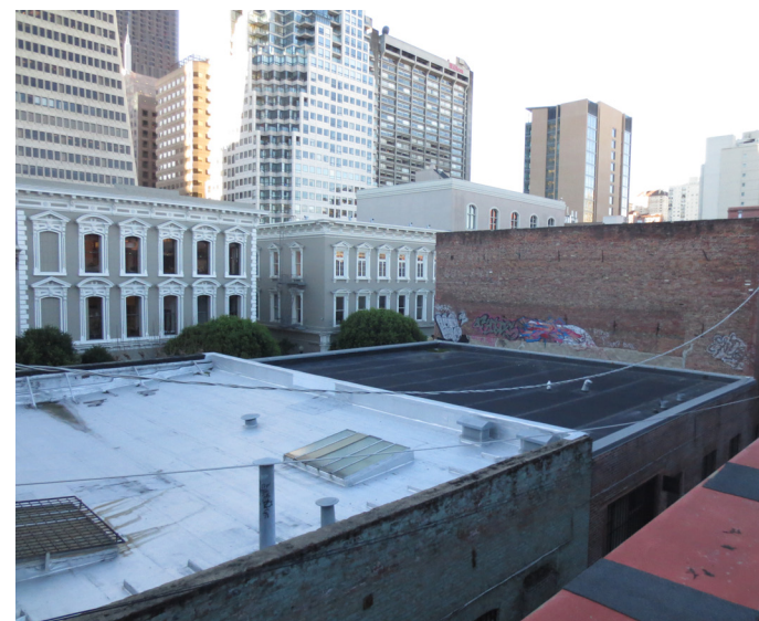
view looking southwest towards Gold, 48 Gold parapet in foreground
