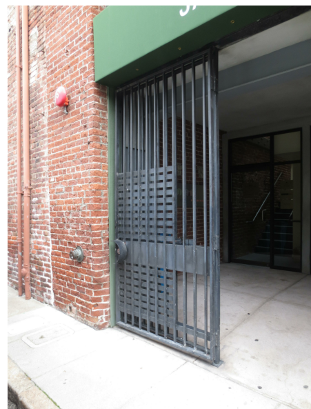
7 View of Existing Entry Gate
