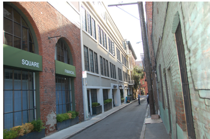
Looking East on Gold Street toward Sansome Street 40&48 Gold St are designed to front onto Gold
