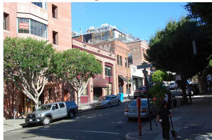
View Looking North on Montgomery new living units above historic structure visible from street
