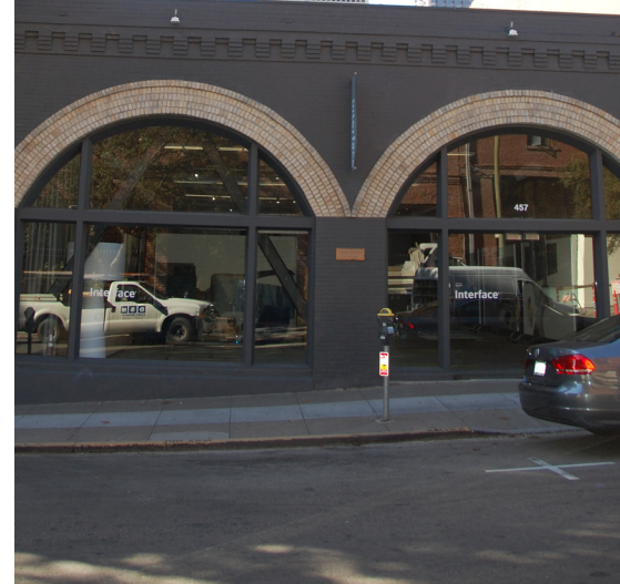
457 Pacific row-lock brick at arch, brick parapet
