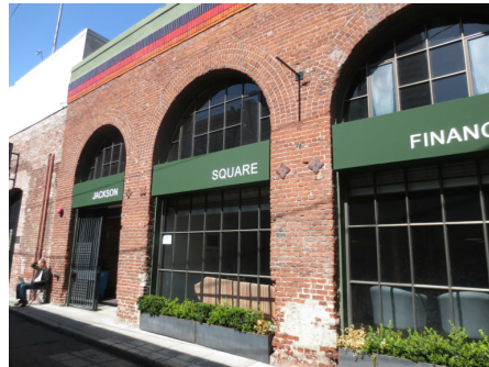
1 View of Existing Facade
