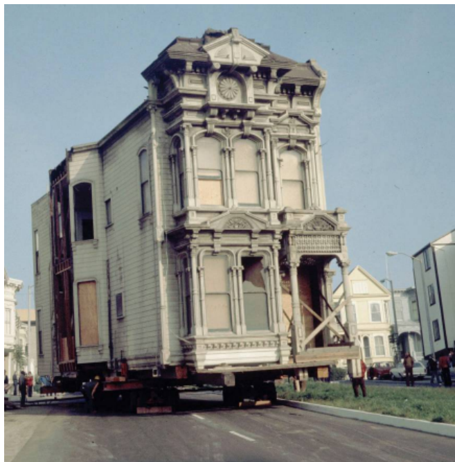
Relocating a 19 th century house in the Western Addition.
