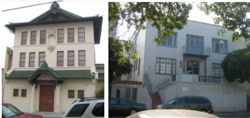
Left to right: The Morning Star School at 1715 Octavia Street and Kinmon Gakkuen / Nihonmachi Little Friends building at 2031 Bush Street. (Page & Turnbull.)
