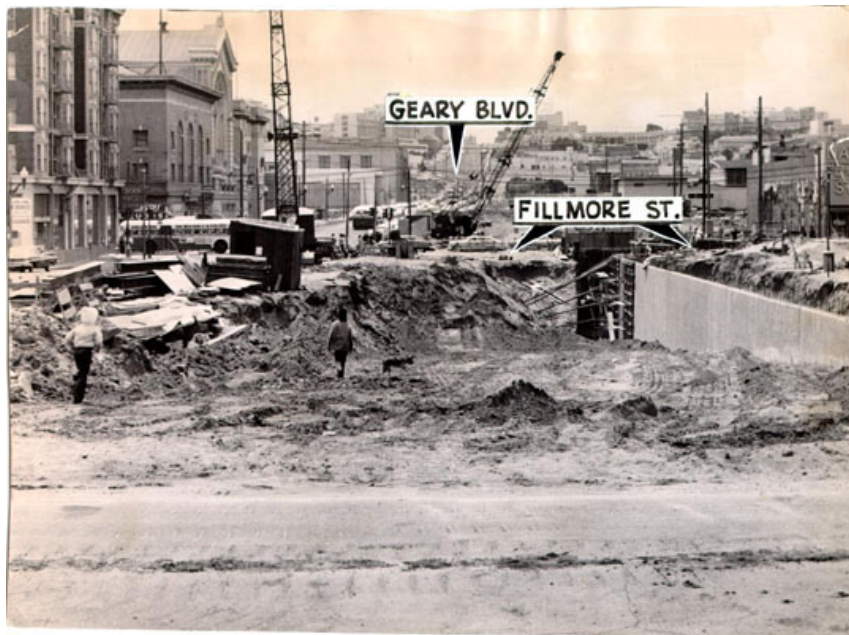
Demolition for the Geary Expressway, 1960. (Collection of San Francisco Public Library)
