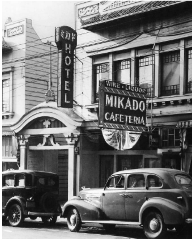
Mikado Hotel and Cafeteria on Post Street, 1930s. (Reproduced in Generations )
