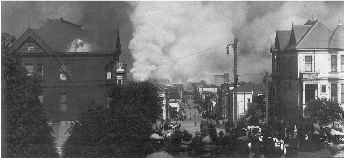
Image 24. At left, 940 Grove Street from Alamo Square during the 1906 Earthquake and Fire of San Francisco. The original upper roof was hipped with a widow's walk. The whitish mass seen at the roof appears to be a chimney on the west side of the main gable roof. The chimney was likely damaged during the earthquake and fell to the ground stripping a gutter below along the way.
