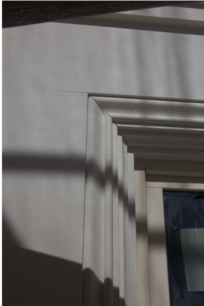
REPAIR OF WINDOW TRIM (TYP.) WORK IN PROGRESS
