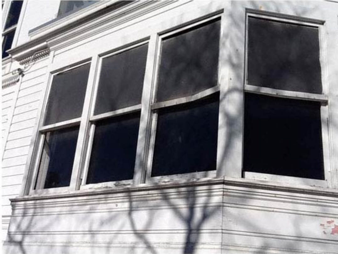
CLOSE-UP SOUTH FACADE
