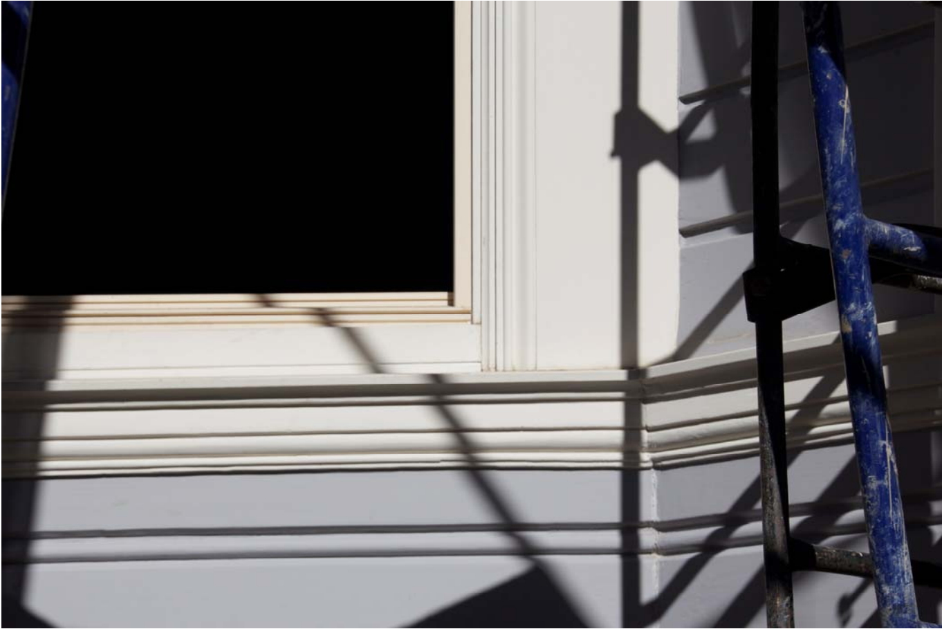
REPAIRED TRIMS AND SIDING SOUTH FACADE
