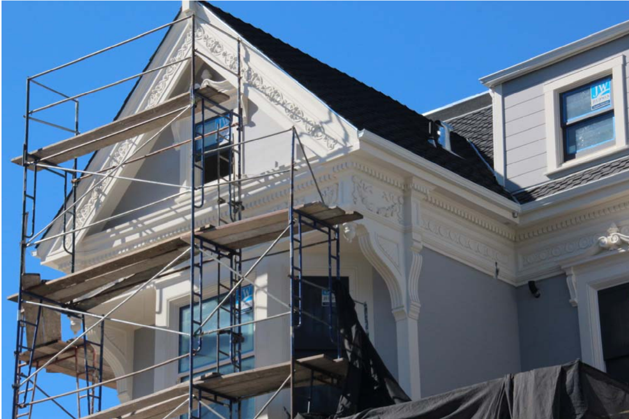
REPAIRED SOUTH FAÇADE WORK IN PROGRESS
