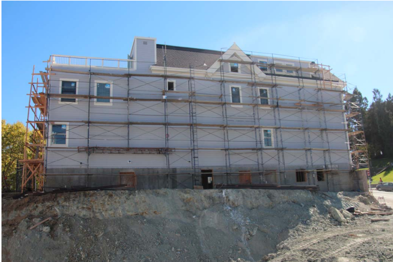
NORTH FAÇADE WORK IN PROGRESS
