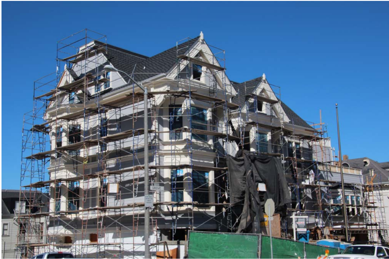
SOUTH & WEST FACADES WORK IN PROGRESS
