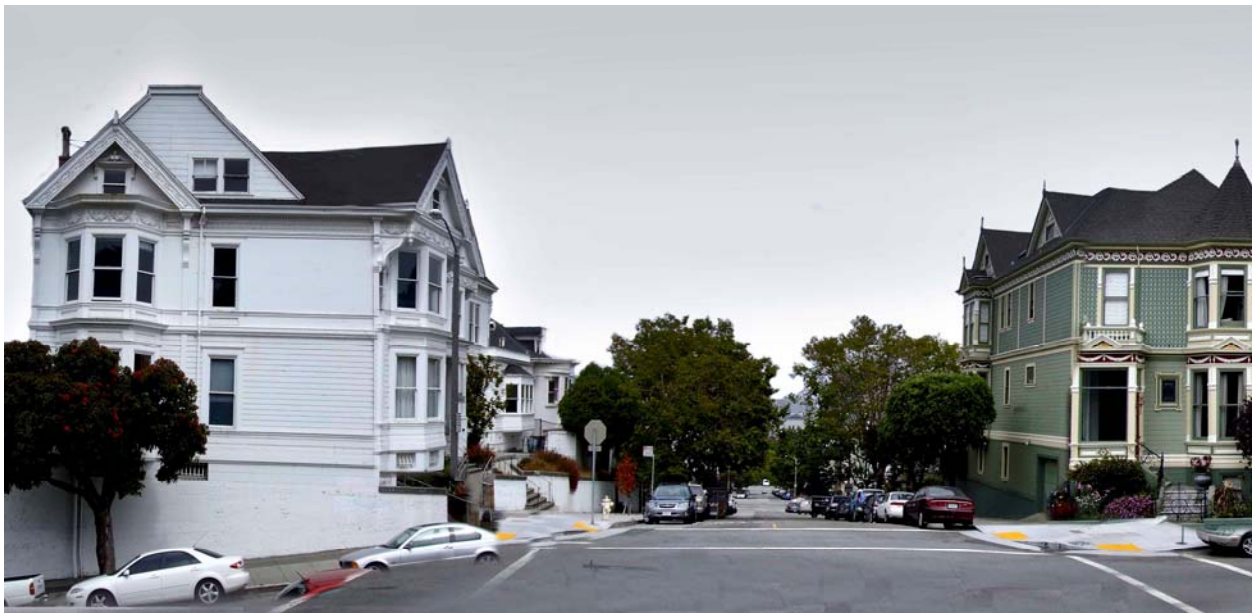
Image 25. The current view along Steiner Street of 940 Grove Street at left from Alamo Square showing how the attic addition adjacent to the west gable changed the original roof massing. Knapp Architects, digital photograph, 2009.
