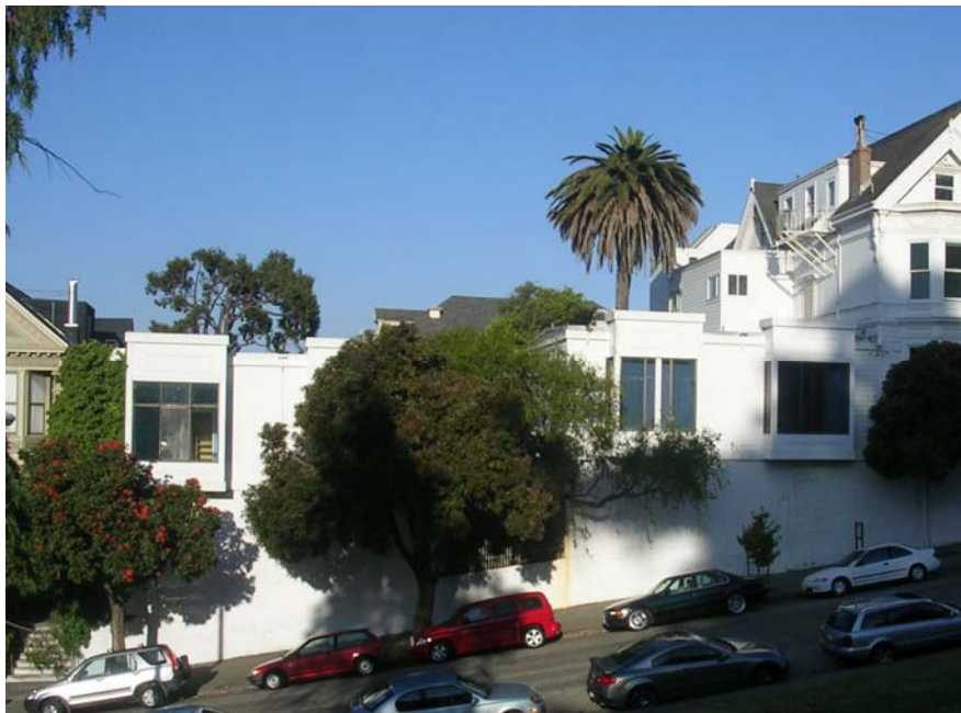
Image 7. North addition at left along the Steiner Street (west) elevation. The top portion of the north façade is visible at the right. Knapp Architects, digital photograph, 2009.
