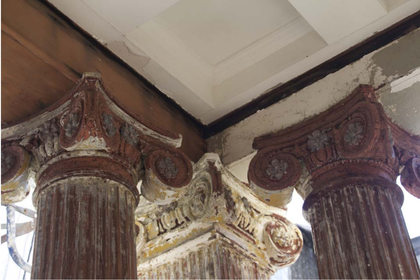
TRIM AND COLUMN REPAIR
