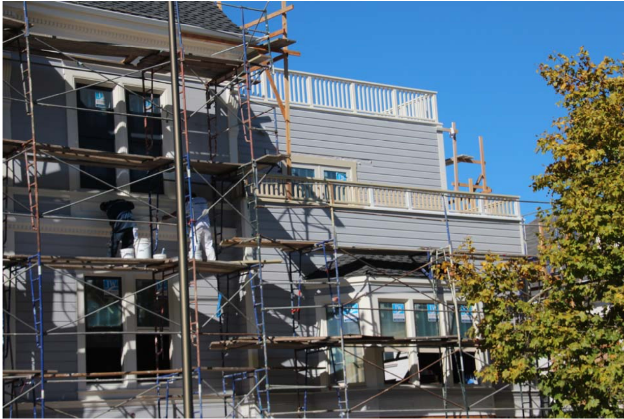
SOUTH FAÇADE – EASTERN PORTION REPAIR WORK IN PROGRESS
