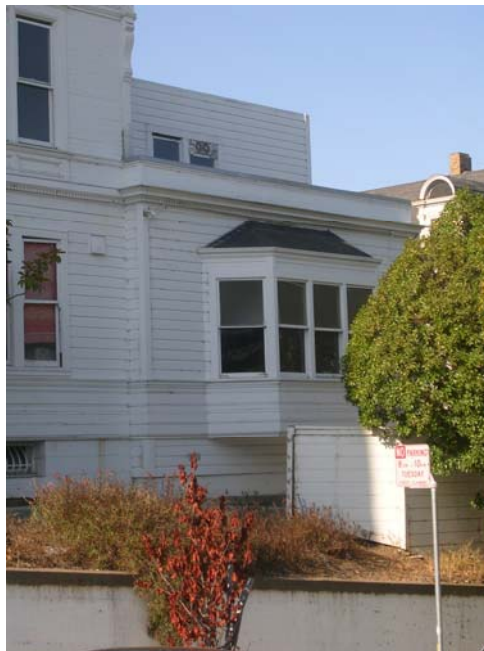
Image 4. East addition along the Grove Street (south) elevation. Knapp Architects, digital photograph, 2009.
