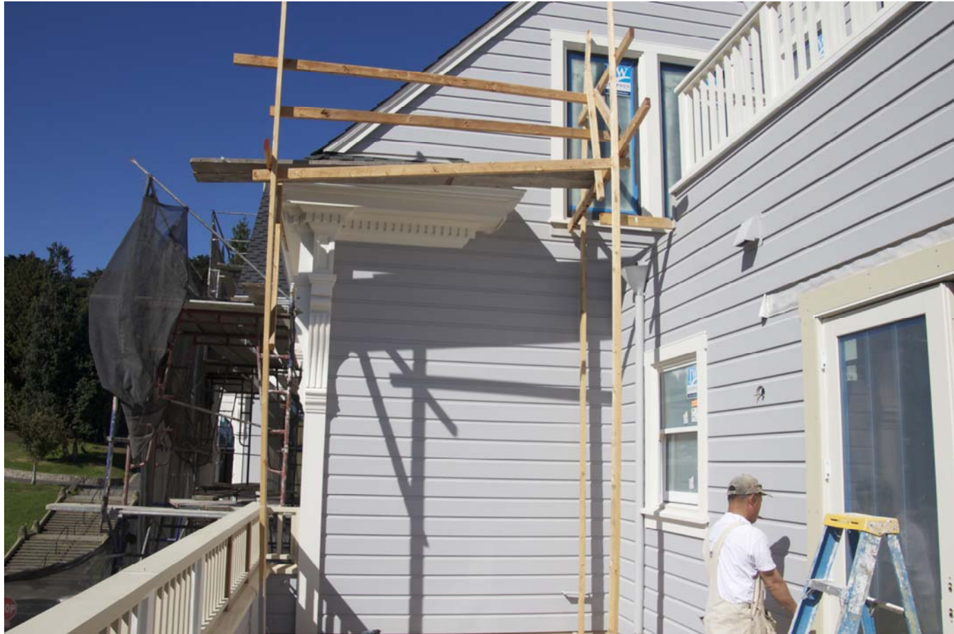
REPAIR AND RENOVATION OF EASTERN SIDE AND FAÇADE WORK IN PROGRESS
