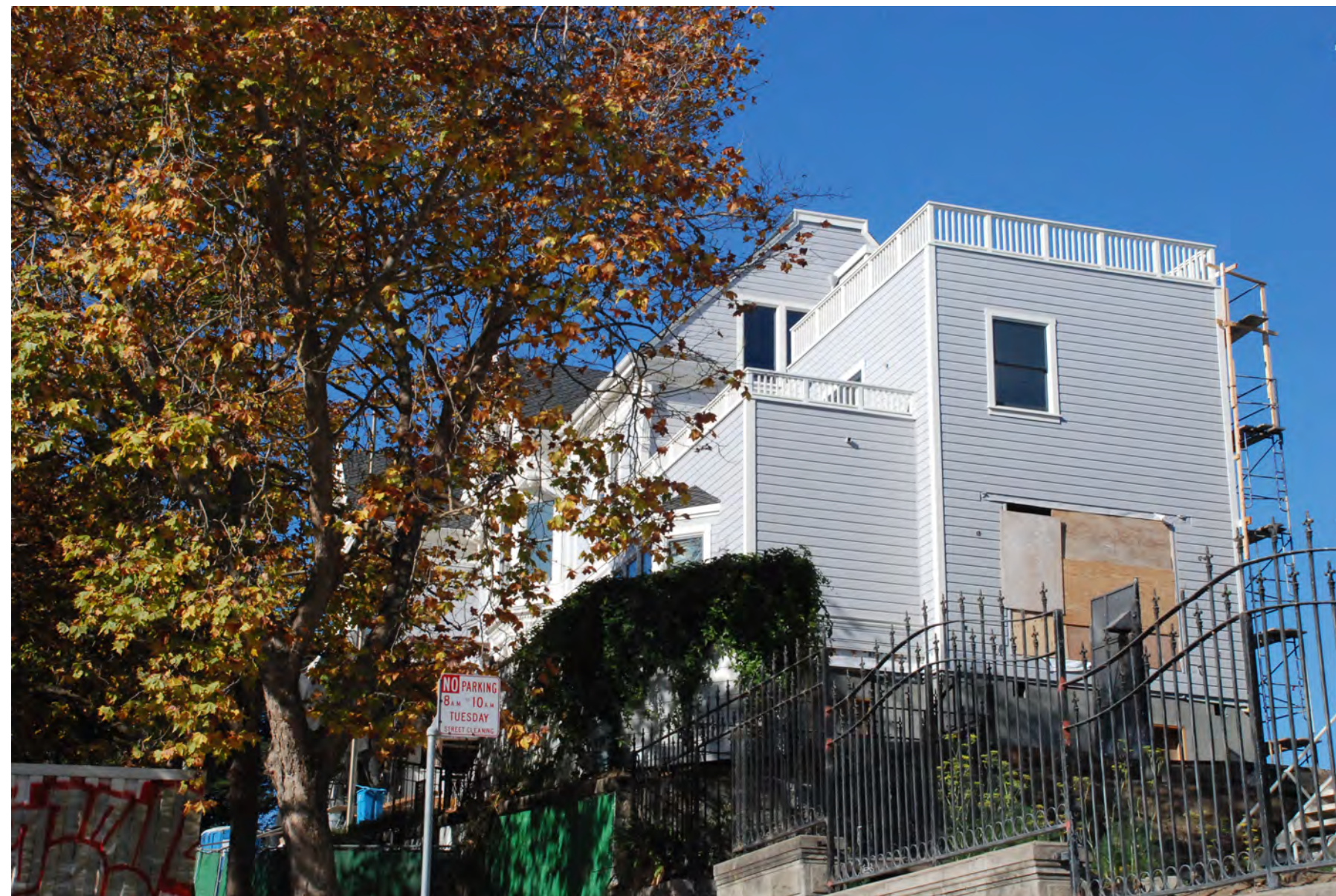
6 PHOTO: EAST FACADE
