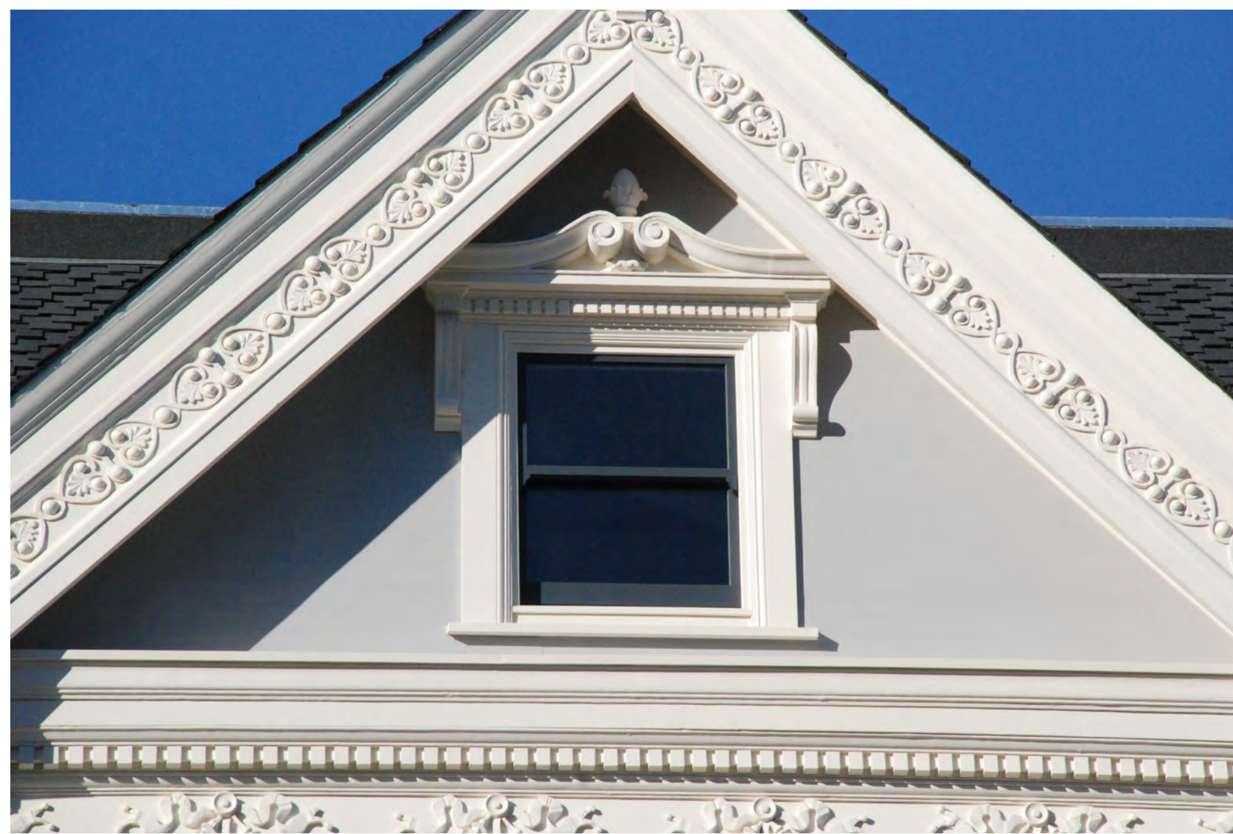
5 PHOTO: GABLE DETAIL
