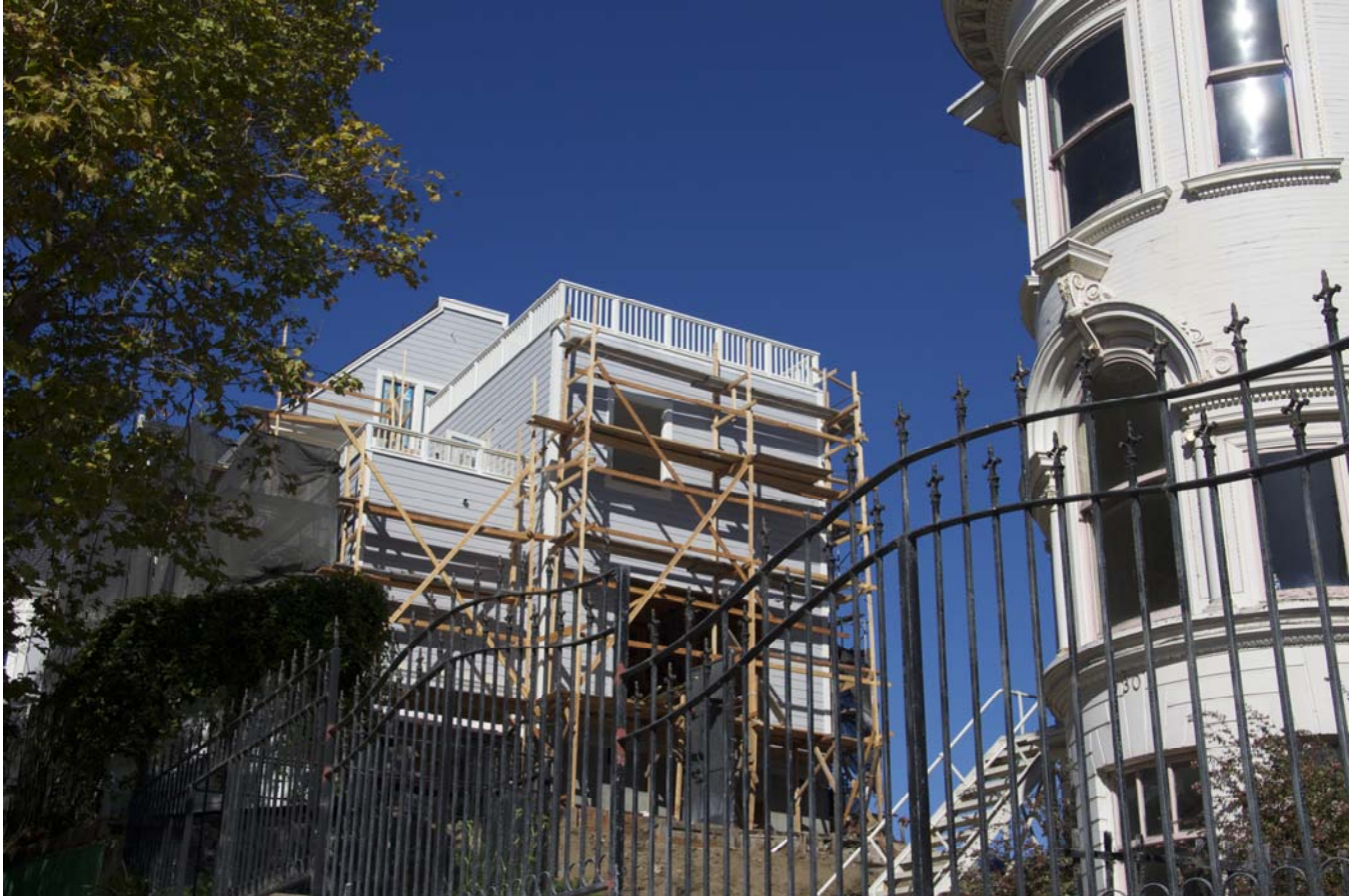
EAST FAÇADE RENOVATION WORK IN PROGRESS
