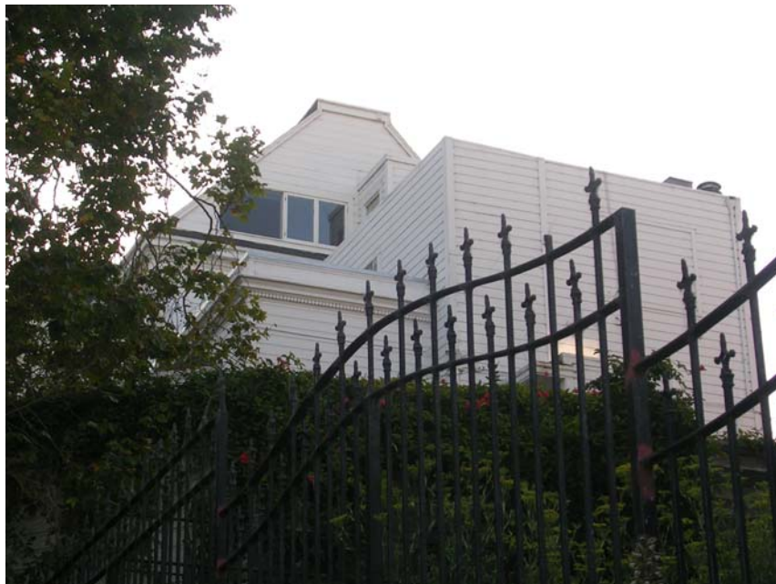
Image 12. Enlarged view of east elevation, the truncated gable addition is seen over the east addition. Knapp Architects, digital photograph, 2009.
