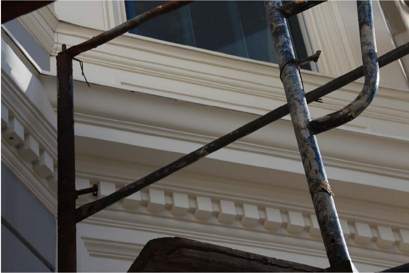
REPAIRED TRIMS AND SIDING SOUTH FACADE
