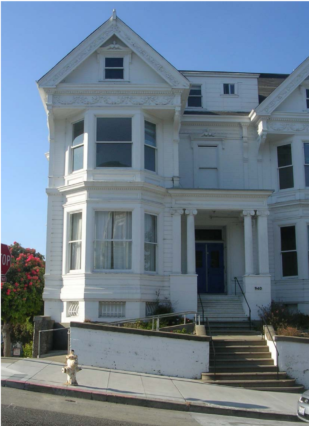
Image 21. Character-defining projecting bay with decorative gable over two-story bay window and basement window at coursed concrete base. Knapp Architects, digital photograph, 2009.
