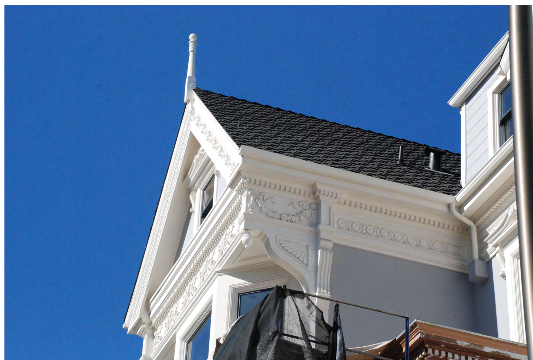
4 PHOTO: GABLE DETAIL
