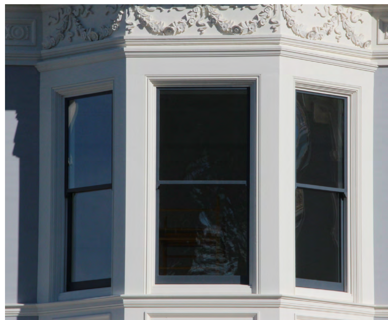
7 PHOTO: (N) WINDOWS
