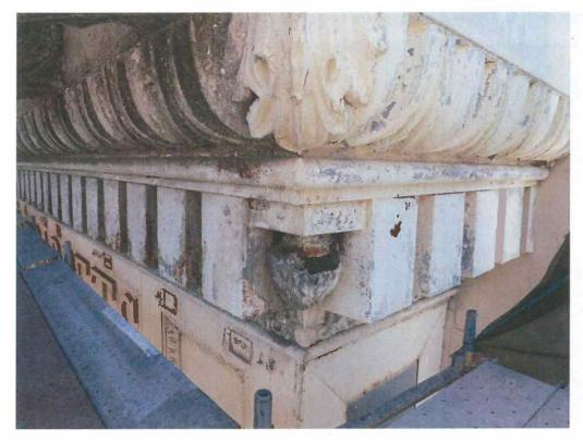
Detail of deteriorated element at dentil course
