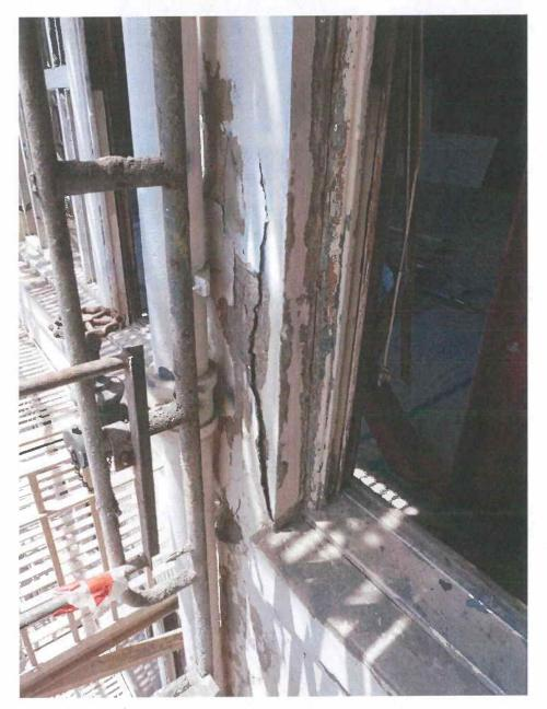
Typical spalling at parged concrete
