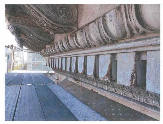
Detail of deterioration pattern at dentil course
