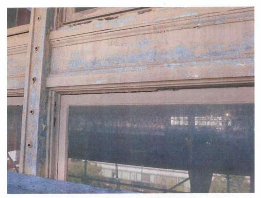
Detail of typical sheet metal spandrel panel
