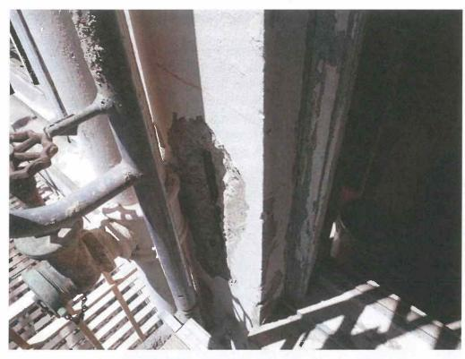
Typical spalling at parged concrete
