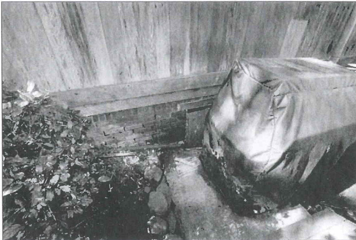
Photo 34. Burr House, 1772 Vallejo Street, 94123. Cottage, detail of URM foundation.
