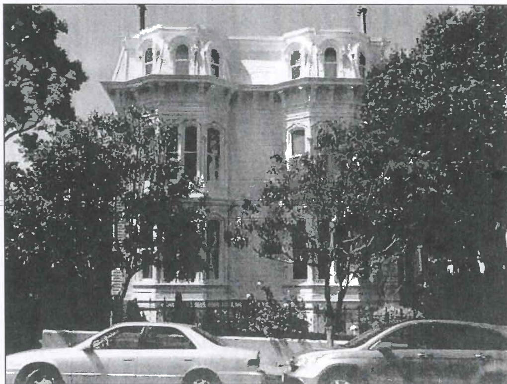
Photo 2. Burr House, 1772 Vallejo Street, 94123. Site, view northwest. After tree trimming. Note that trees are no longer encroaching on house or garden setting
