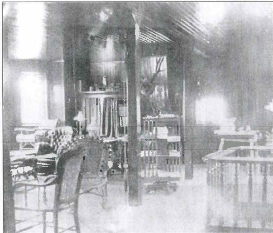
Figure 36. Third floor, n.d. Source: Burr-Allyne family papers and photographs, 1839-2012 (bulk 1900-1930), California Historical Society.
