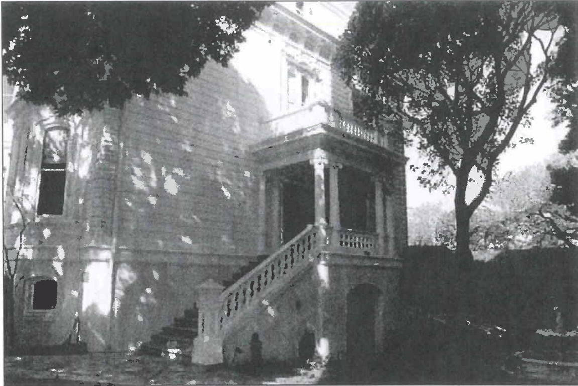
Photo 15. Burr House, 1772 Vallejo Street, 94123. East elevation, view northwest. Note mature trees encroaching on porch and house.
