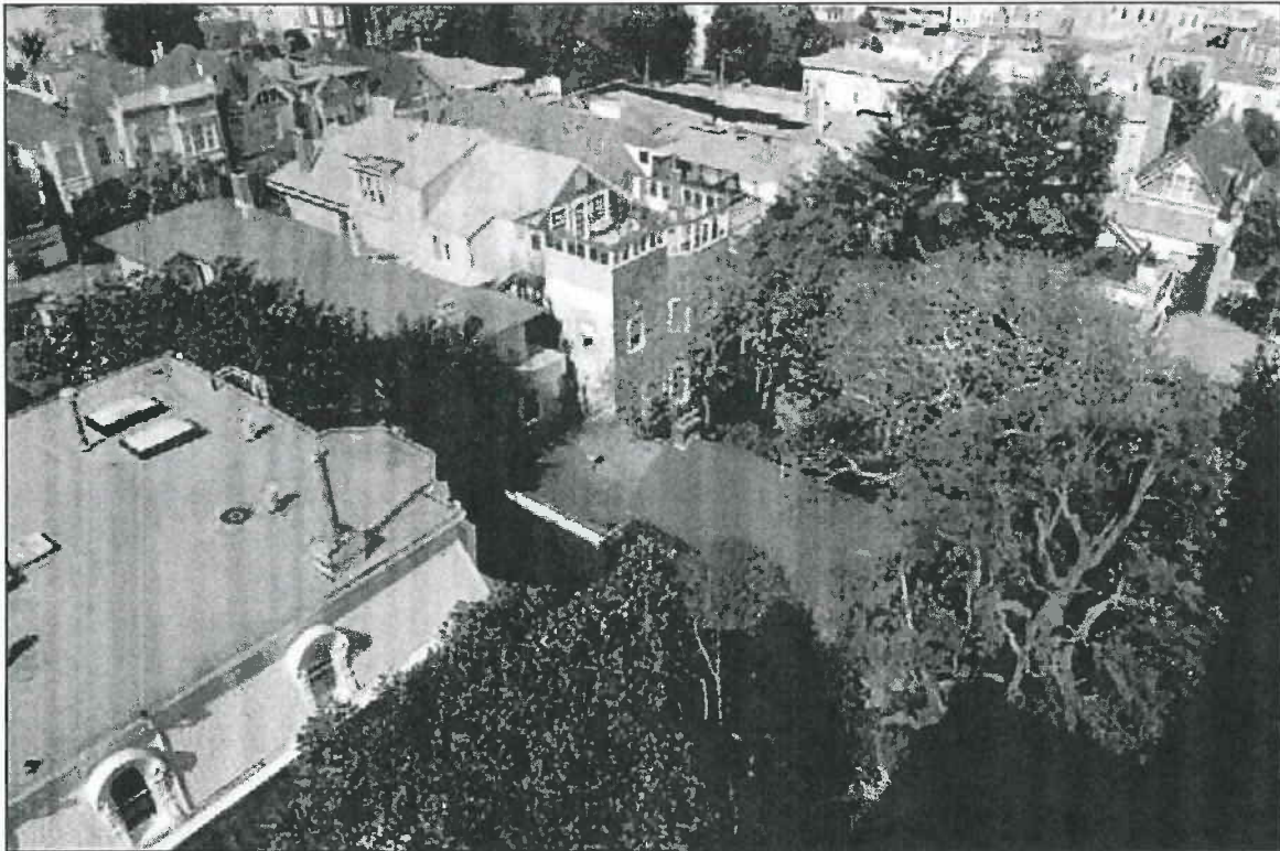
Photo 27. Burr House, 1772 Vallejo Street, 94123. Roof of garage and cottage, view northwest.
