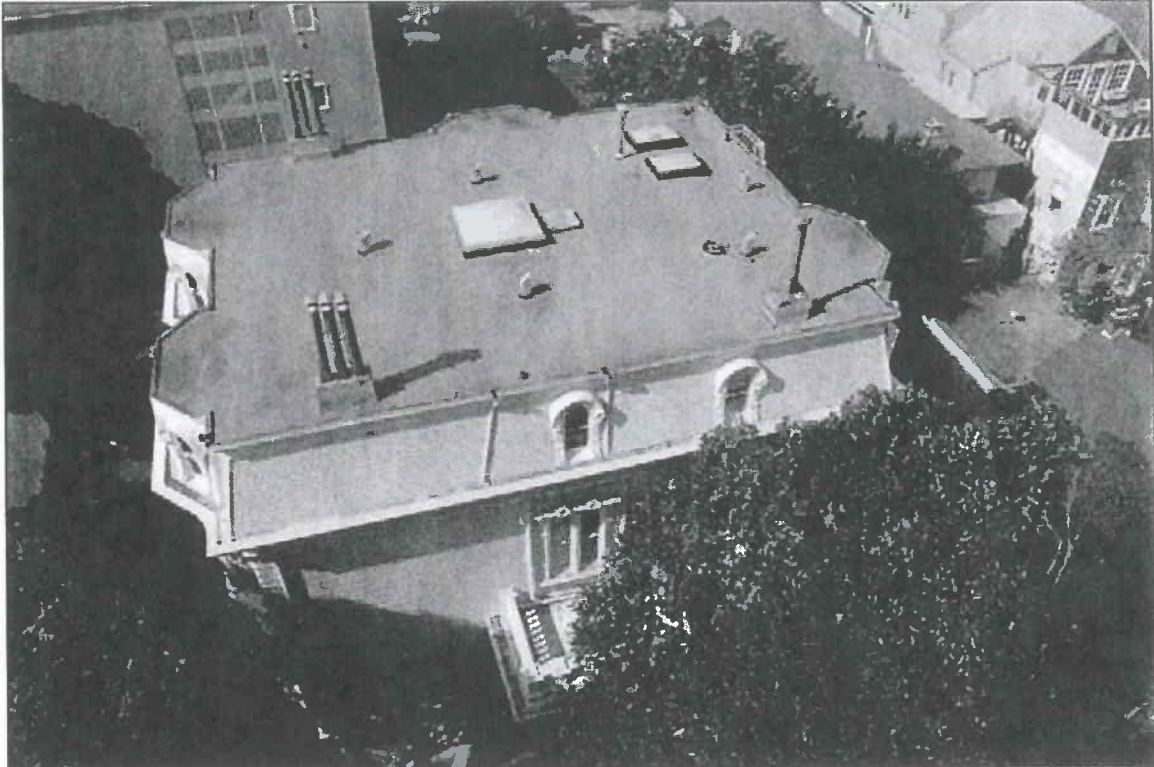
Photo 24. Burr House, 1772 Vallejo Street, 94123. Roof of house, view northwest.
