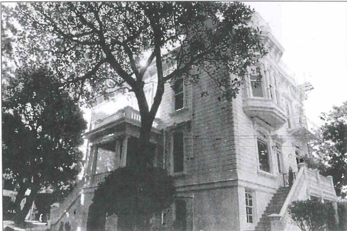
Photo 16. Burr House, 1772 Vallejo Street, 94123. East (left) and north (right) elevations, view southwest. Note mature trees encroaching on house.
