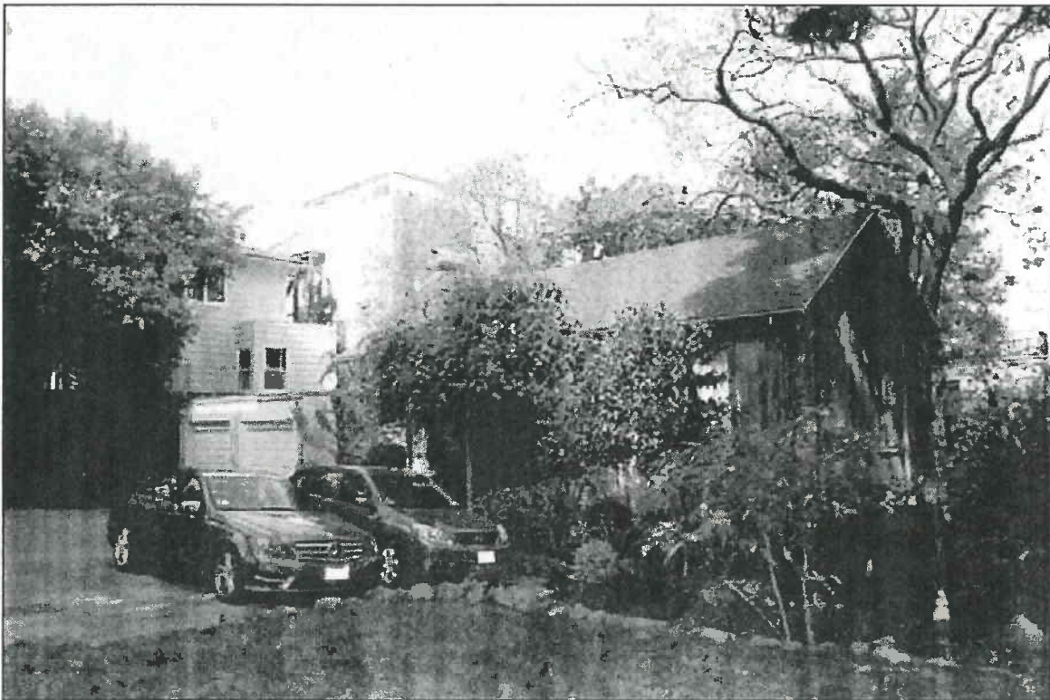
Photo 31. Burr House, 1772 Vallejo Street, 94123. Cottage, view northwest.
