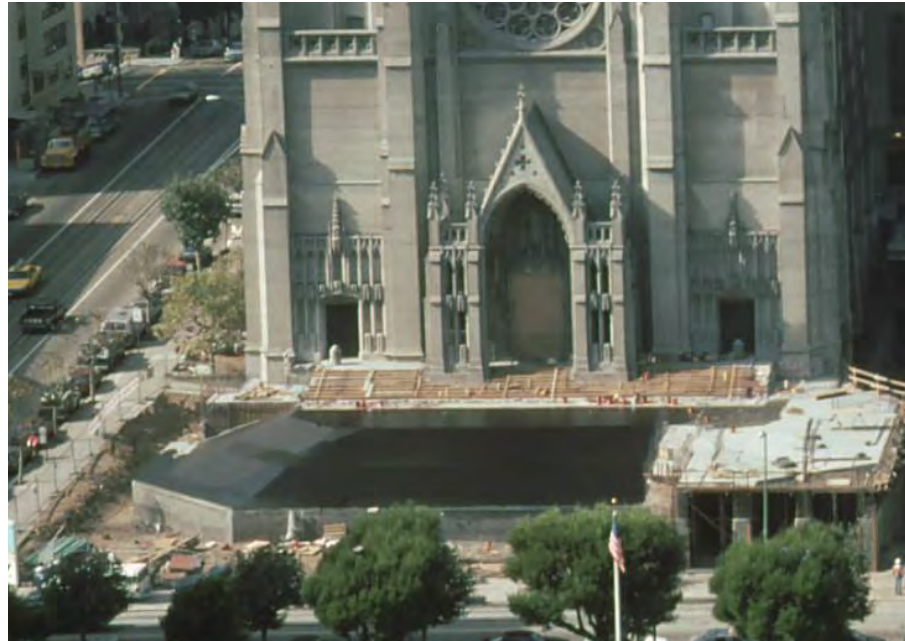
7. Overall View west showing project during construction, ca. 1994 (Michael Lampen)
