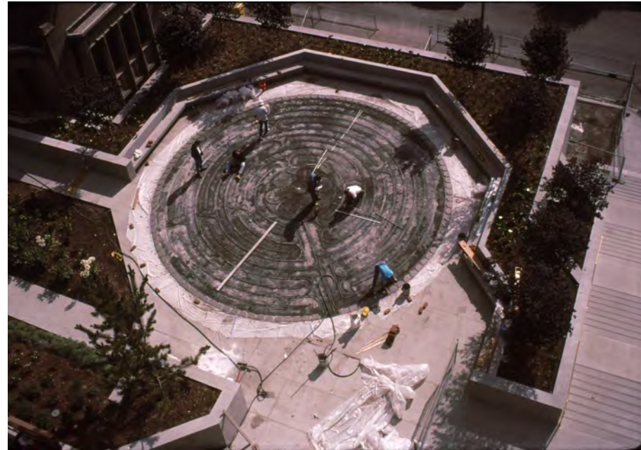
10. View south across new stairs construction, ca. 1994 (Michael Lampen)
