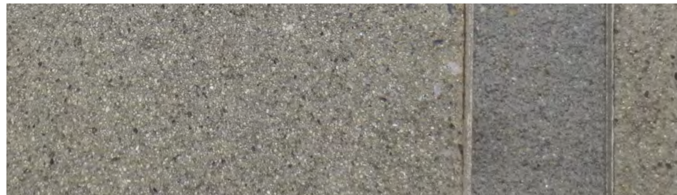
Existing concrete striping with metal insert
