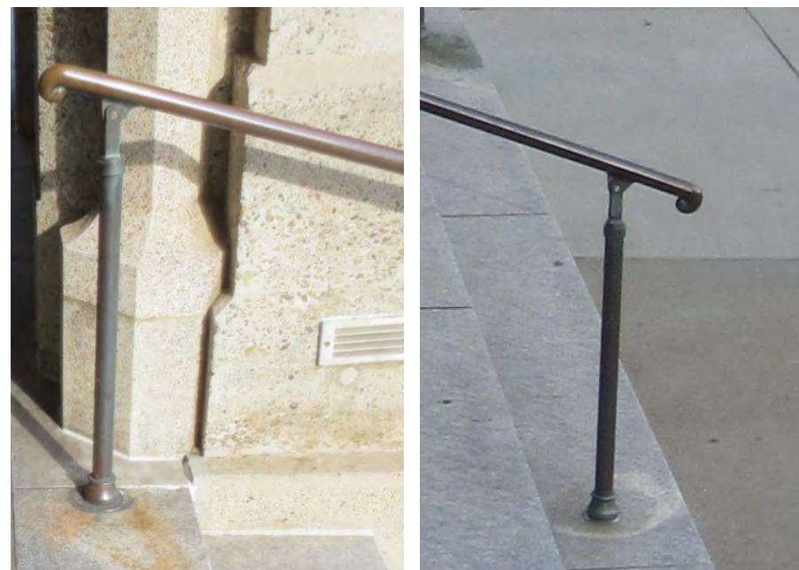
Existing Handrails at Stone Steps with Concrete Steps to plaza beyond.
