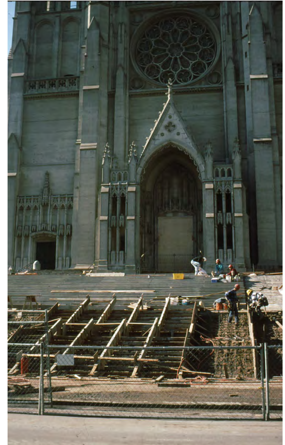
9. Construction of the new Great Stair. (Michael Lampen)
