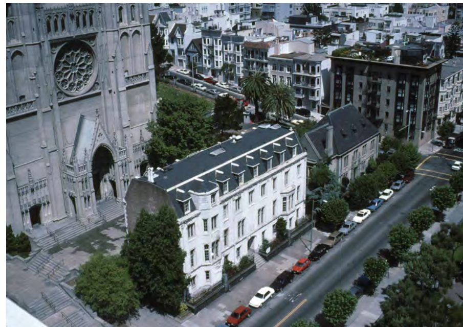
5. Gibbs Memorial hall, Ca. 1993 prior to demolition (Michael Lampen)
