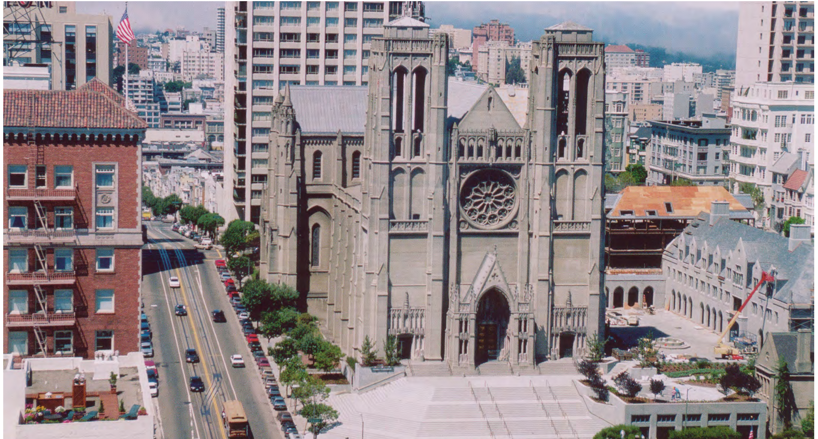
6. Overall view west showing project during construction, ca. 1994 (Michale Lampen)
