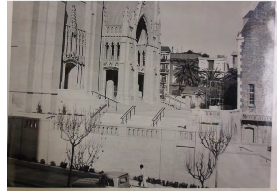
3. View from California St., showing the Great East Entrance of Grace Cathedral, Note: Handrails at porch are missing (Grace Cathedral Archives, #7366) November, 1964
