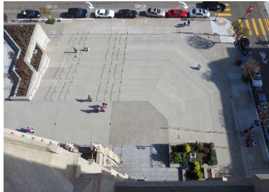
Concrete Steps at Great Stair Note: patched concrete
