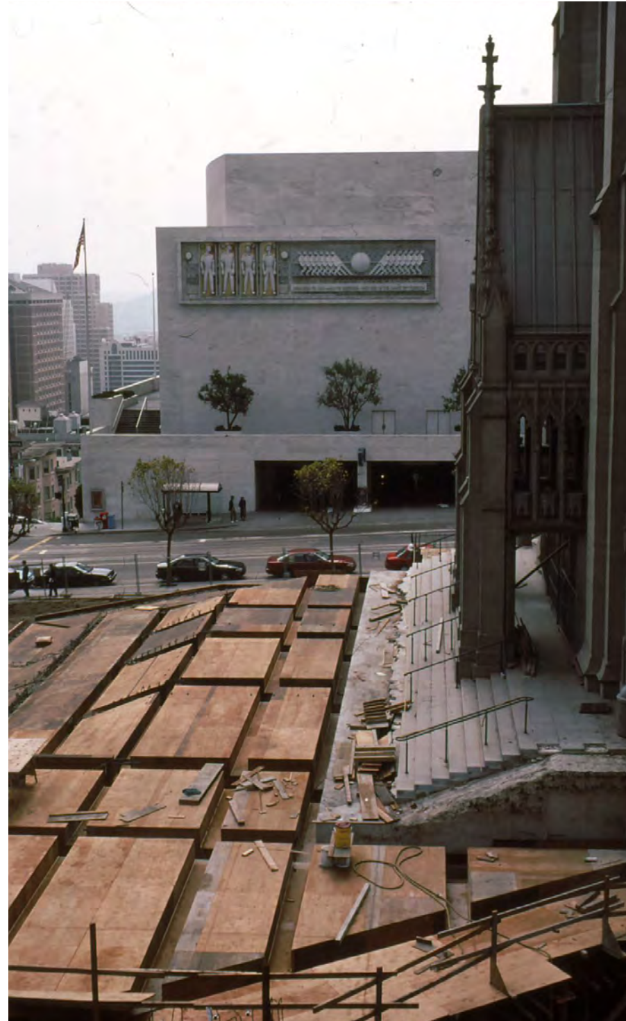
8. Construction of the new Great Stair. (Michael Lampen)
