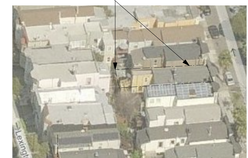
AERIAL VIEW FROM REAR
