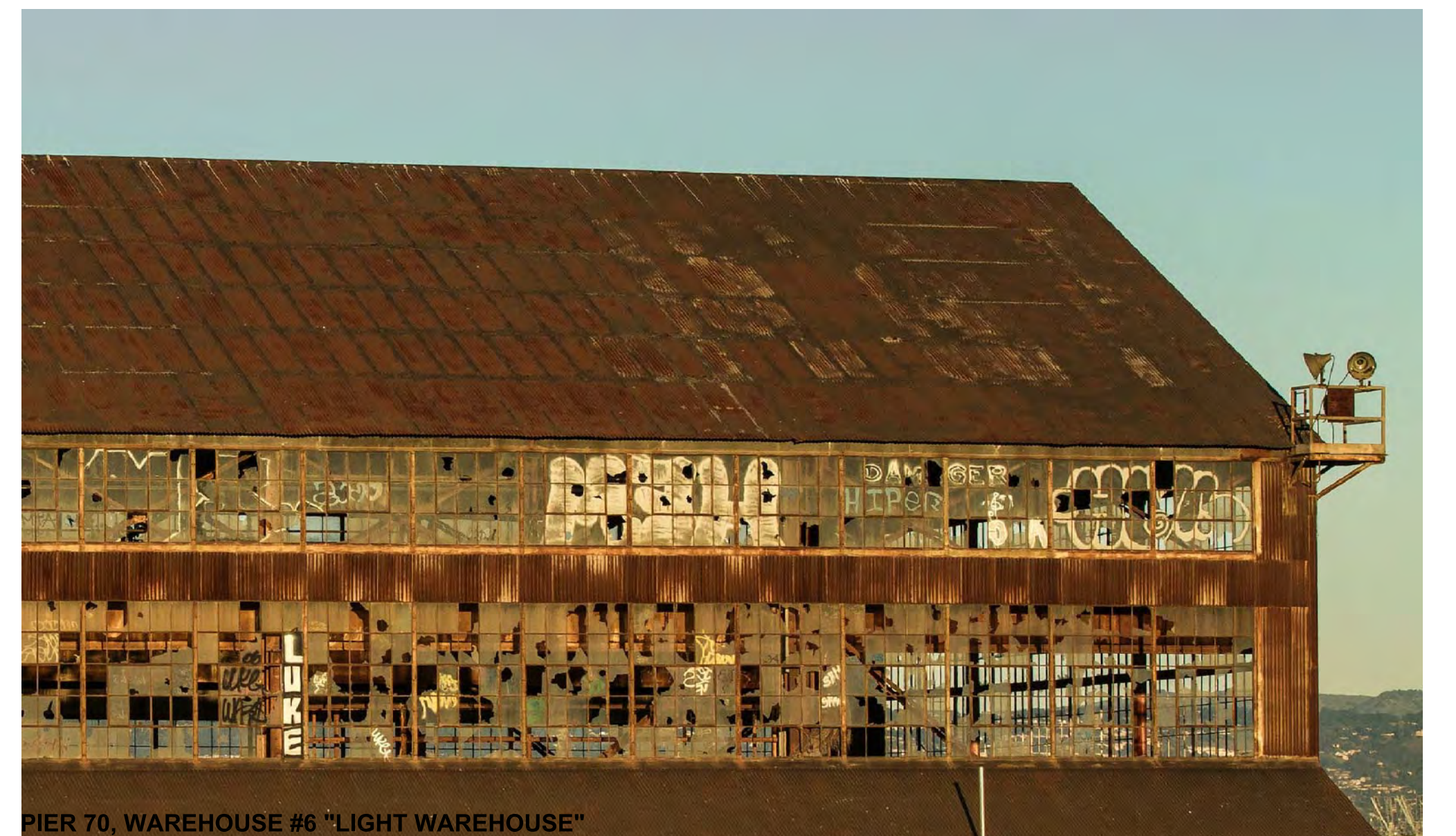
PIER 70, WAREHOUSE #6 "LIGHT WAREHOUSE"
