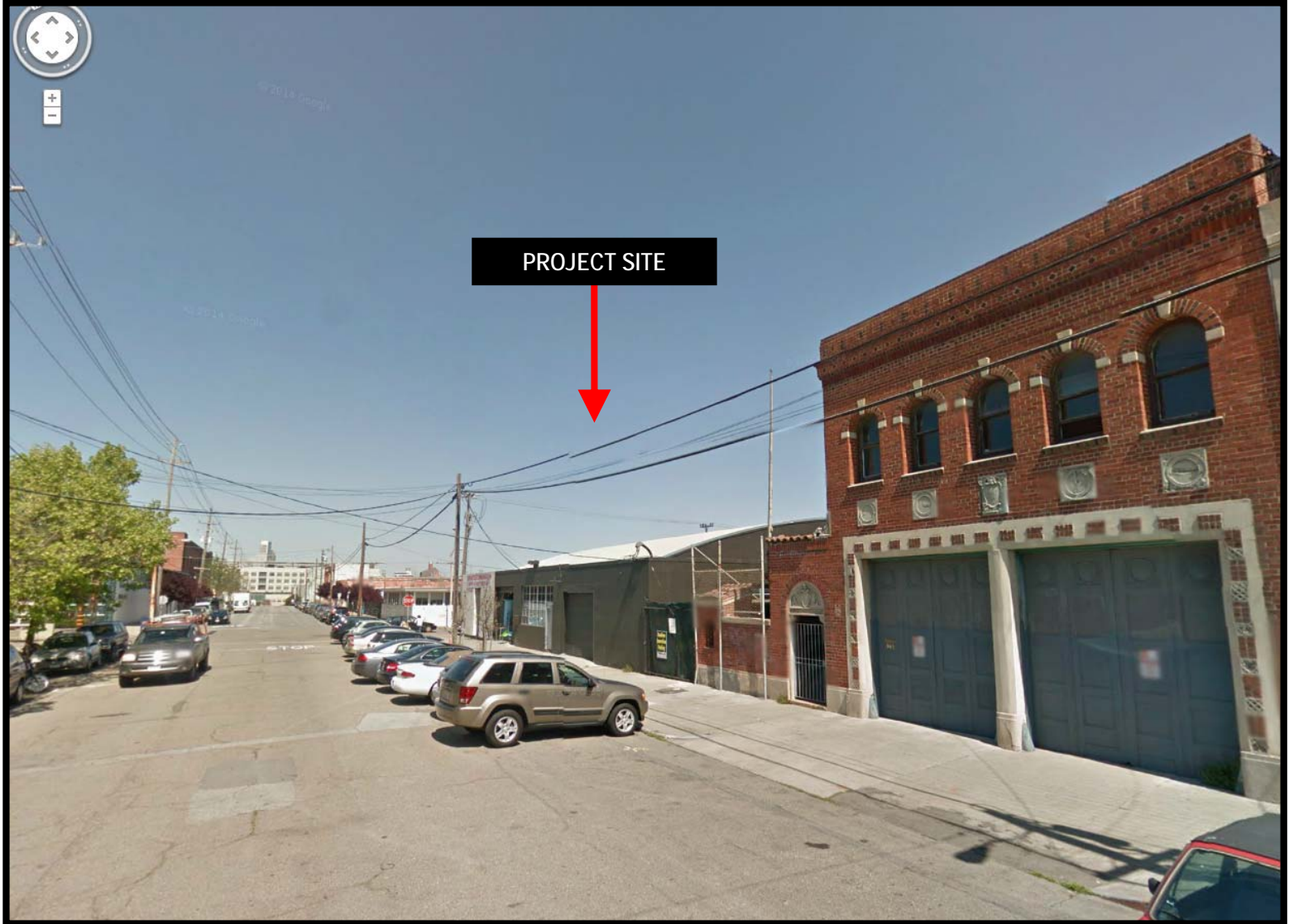
901 Tennessee Street, View down Tennessee Street
