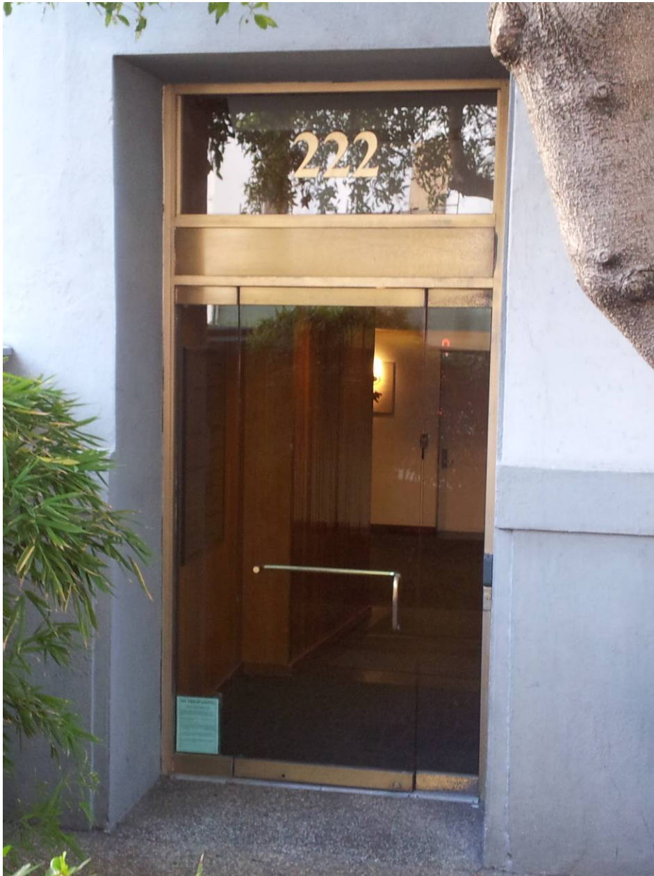
Figure A9. View of 220 Vallejo Street entrance, along south elevation near rear of building (Architectural Resources Group, January 2013). This currently serves as the building's primary entrance.
