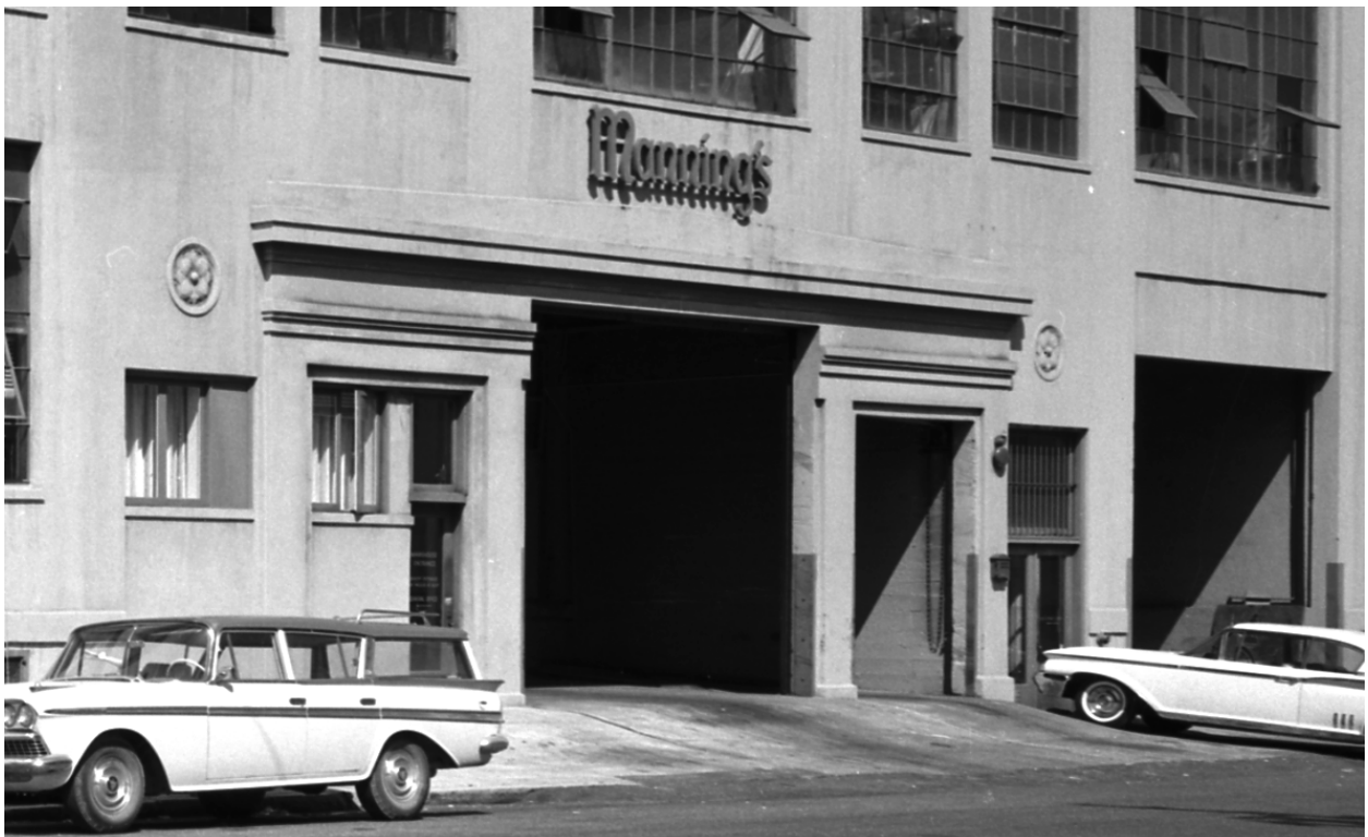
Figure 2. Detail of San Francisco Assessor's photograph (dated August 16, 1961) showing the building's main entry along Battery Street (San Francisco History Center, San Francisco Public Library). The building's main entrance had already undergone some alteration at the time this photograph was taken. In particular, the entablature appears to have been partially cut through to accommodate a service entry larger than the original main entrance.
