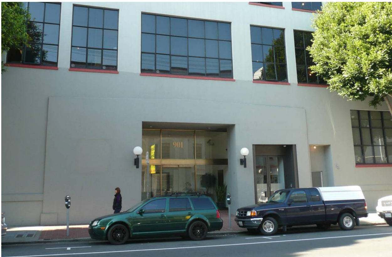
Figure A4. Main entrance, along east elevation (Architectural Resources Group, January 2013).
