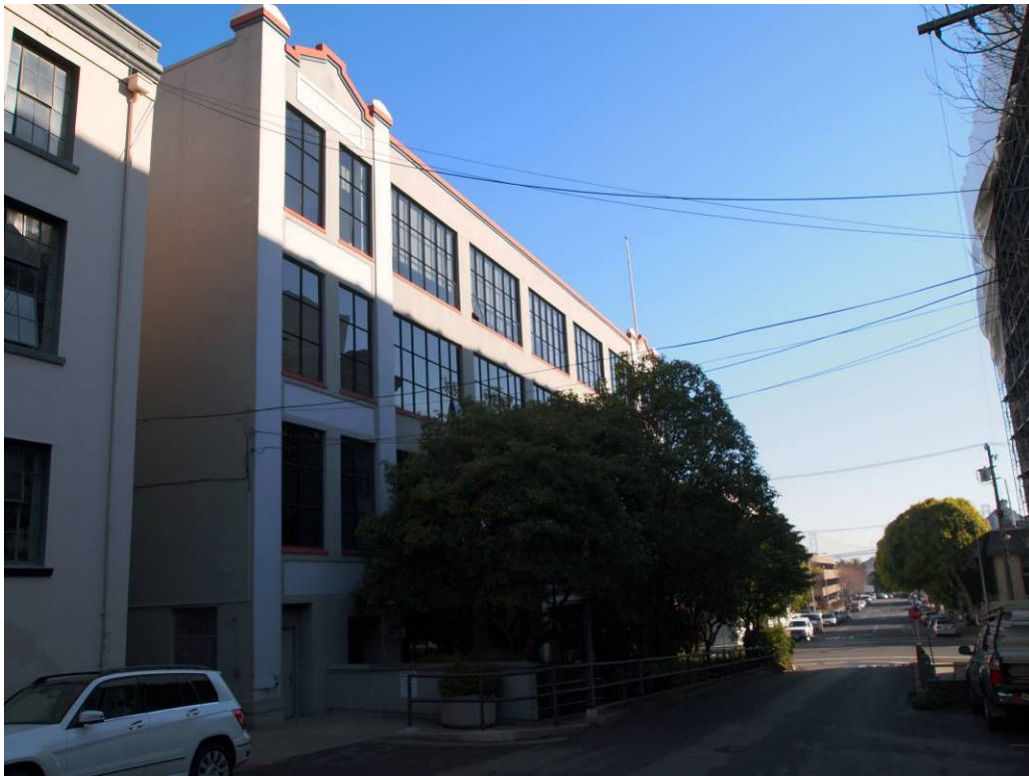
Figure A6. View of south elevation, looking east (Architectural Resources Group, January 2013).
