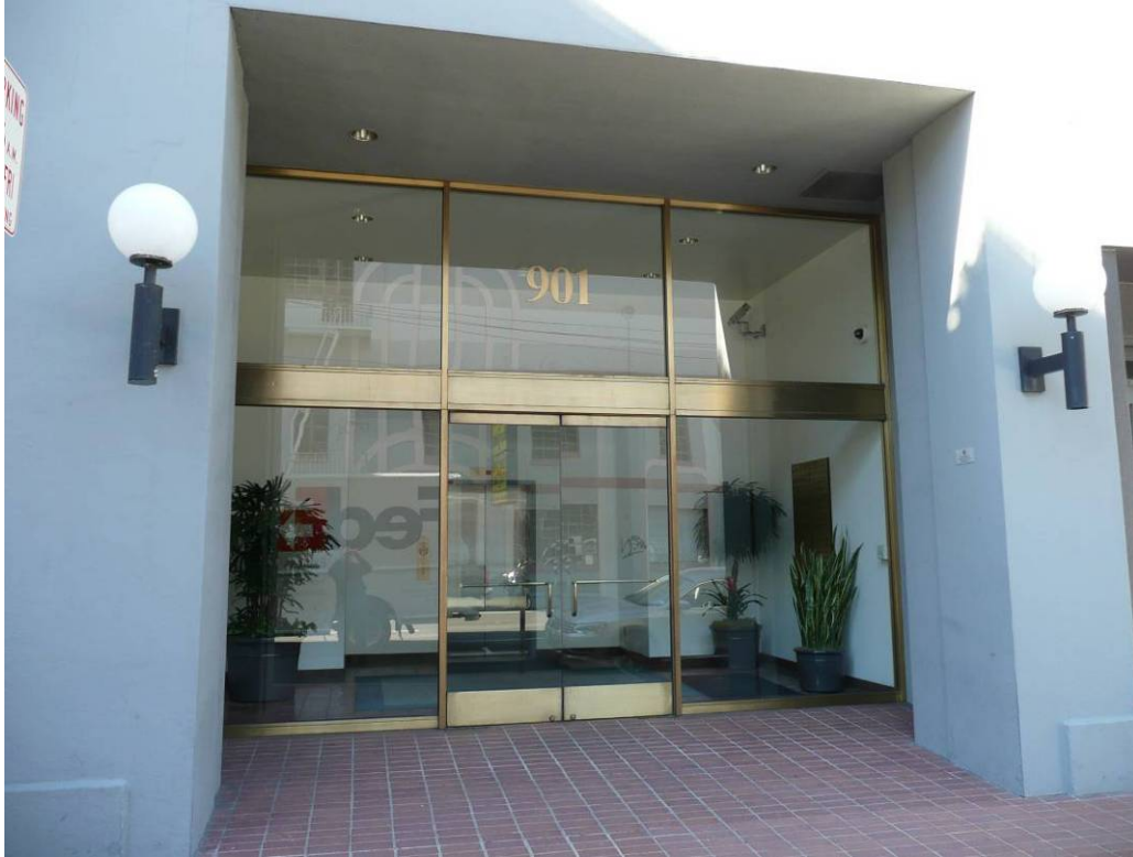
Figure A5. Detail of main entrance, along east elevation (Architectural Resources Group, January 2013).
