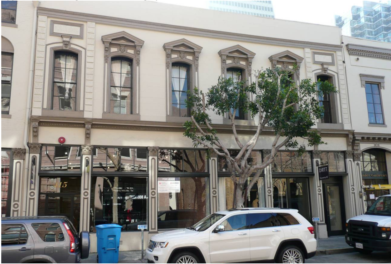
Figure A12. 415-431 Jackson Street, home of the Petri Italian-American Cigar Co. from 1912 to 1922 (Architectural Resources Group, February 2013). Compare Figure B1 below.
