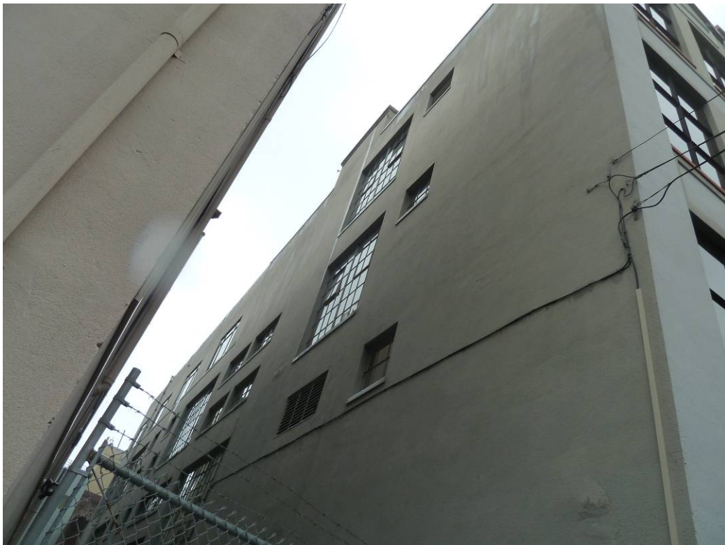
Figure A11. View of west elevation (Architectural Resources Group, January 2013).
