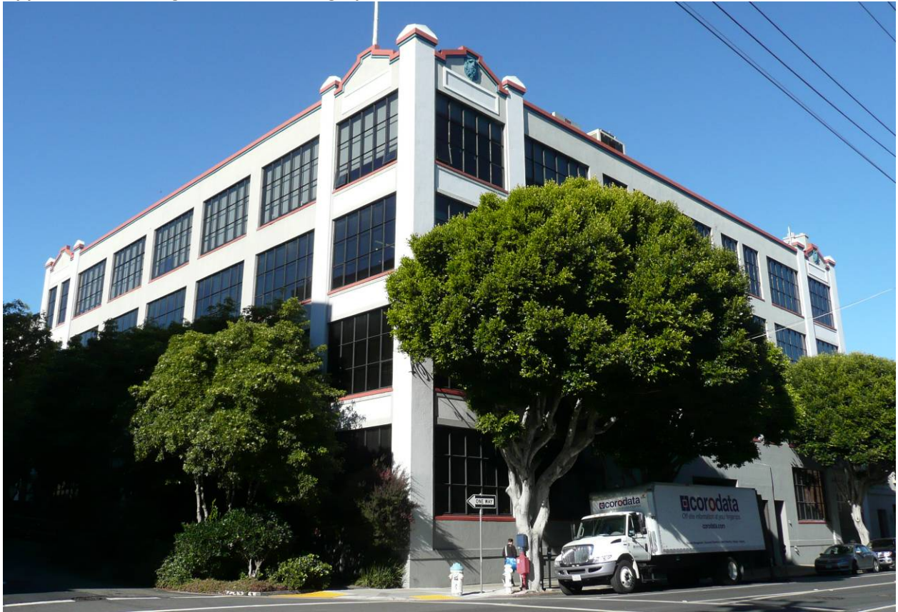
Figure A1. View of south and east elevations, looking northwest (Architectural Resources Group, January 2013).
