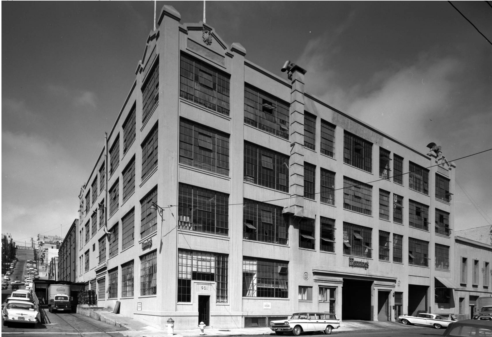
Figure B8. San Francisco Assessor's photograph (dated August 16, 1961) of 901 Battery Street, looking northwest (San Francisco History Center, San Francisco Public Library).
