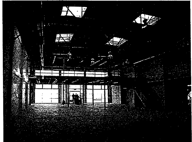
Interior space, looking northeast toward front of building.
