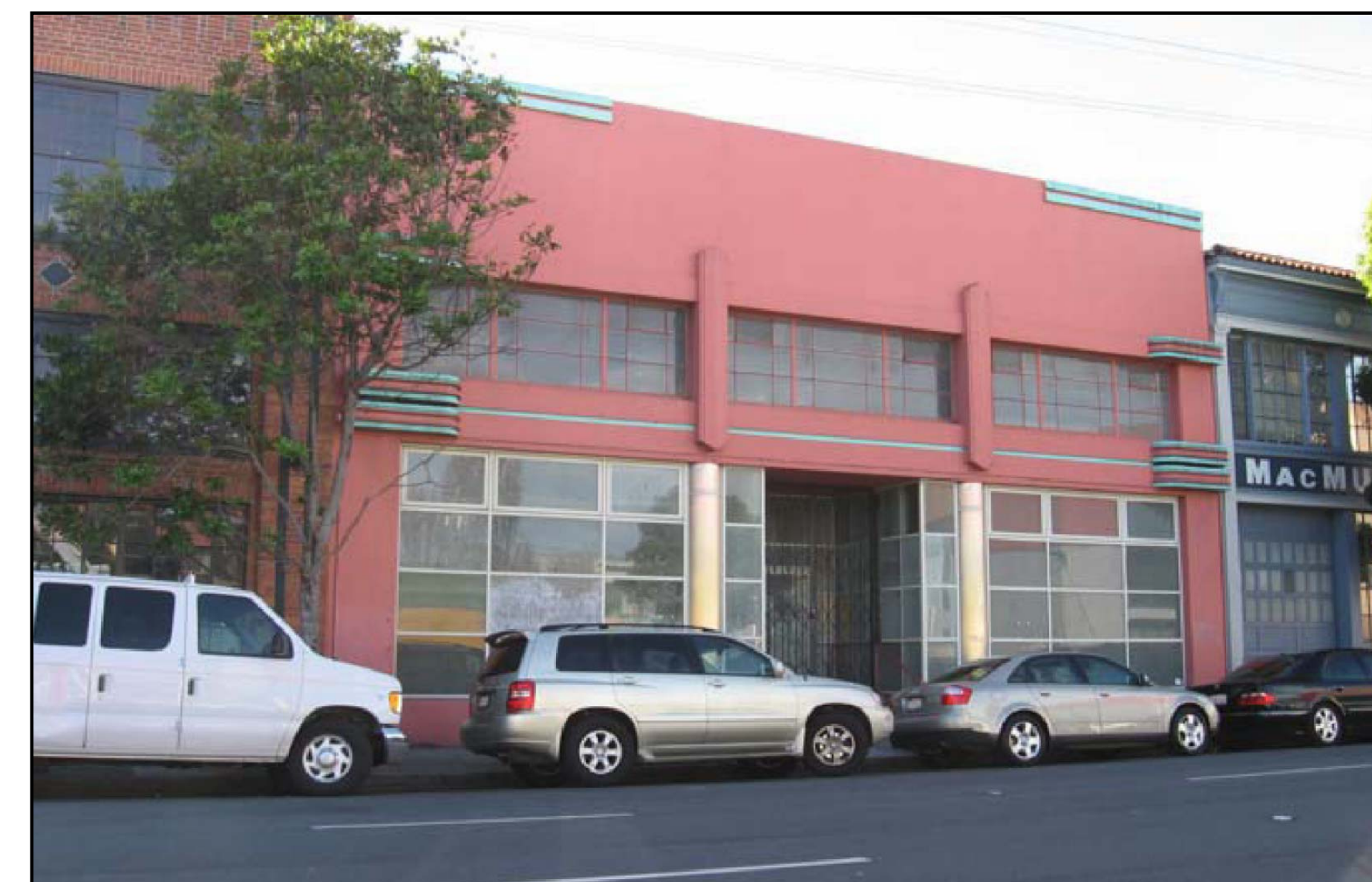
SEVENTH STREET FACADE PHOTO SCALE:
