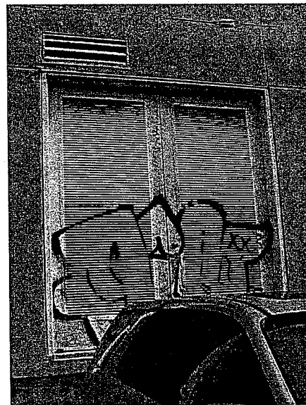
Service entrance, rear facade.
