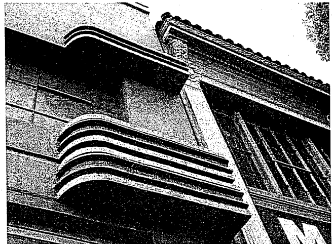
Art Moderne brackets, primary facade.
