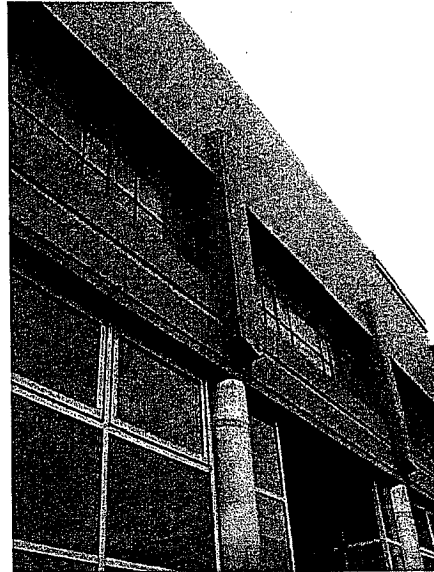
Second story, primary facade.
