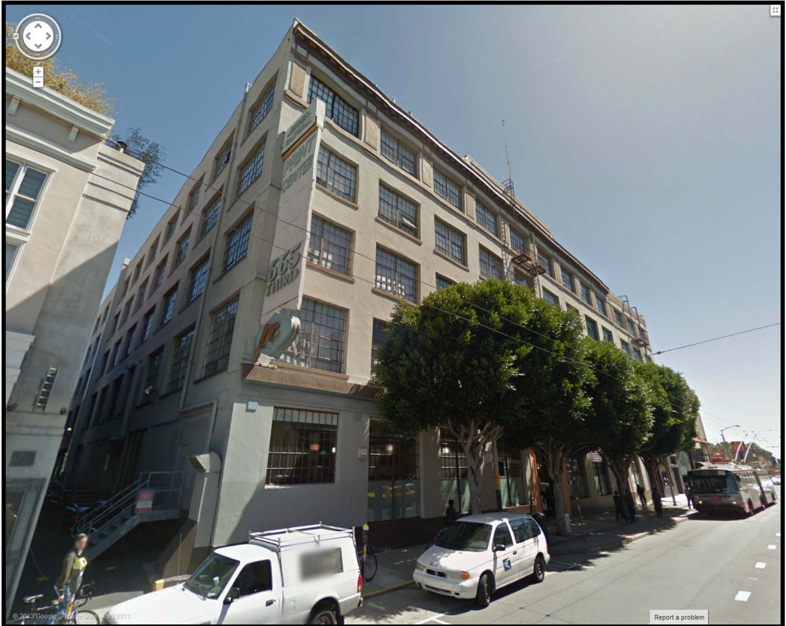
665 3 rd Street, View along 3 rd Street
