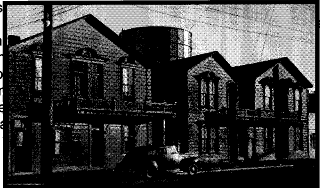
Figure 2: Southwest corner of 22nd and Minnesota Streets, 1951.
