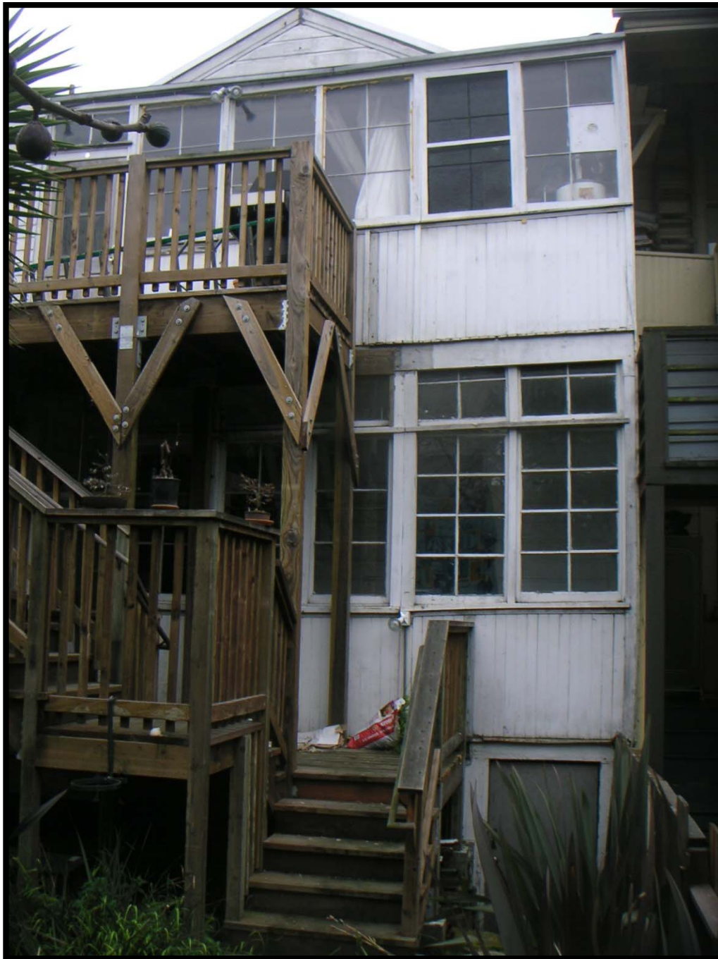
812-814 22 nd Street, Rear Facade (Source: Project Sponsor)
