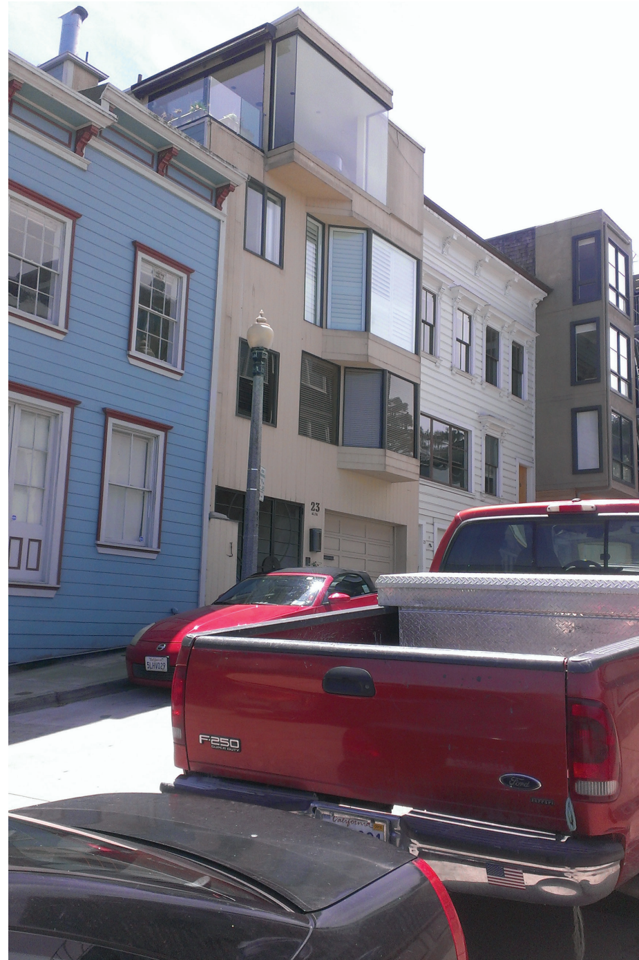
Adjacent buildings along Alta Street
