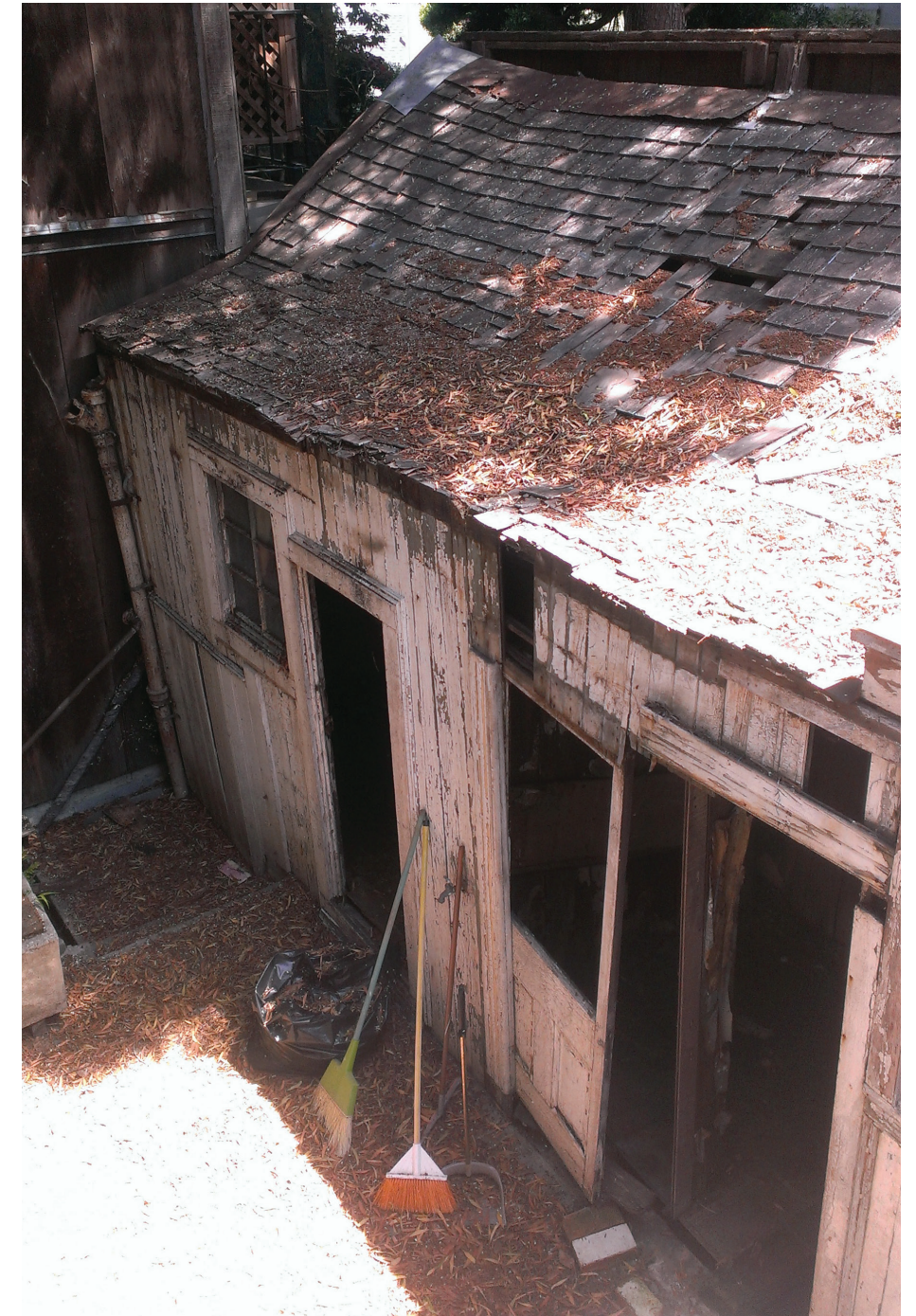
Existing condition of the outhouse
