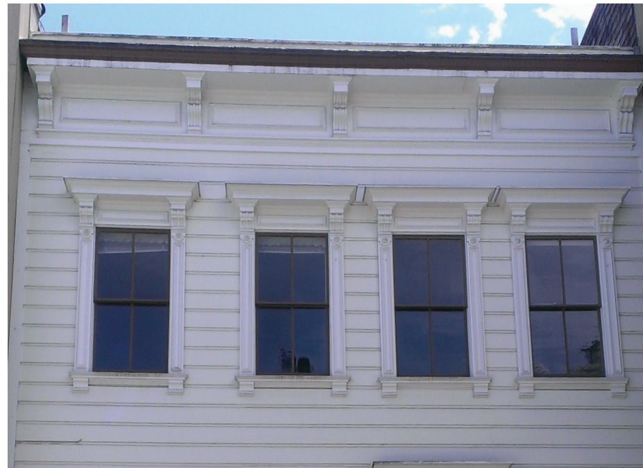
Second floor windows and roof line
