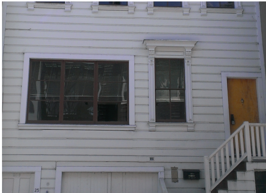
First floor windows and door
