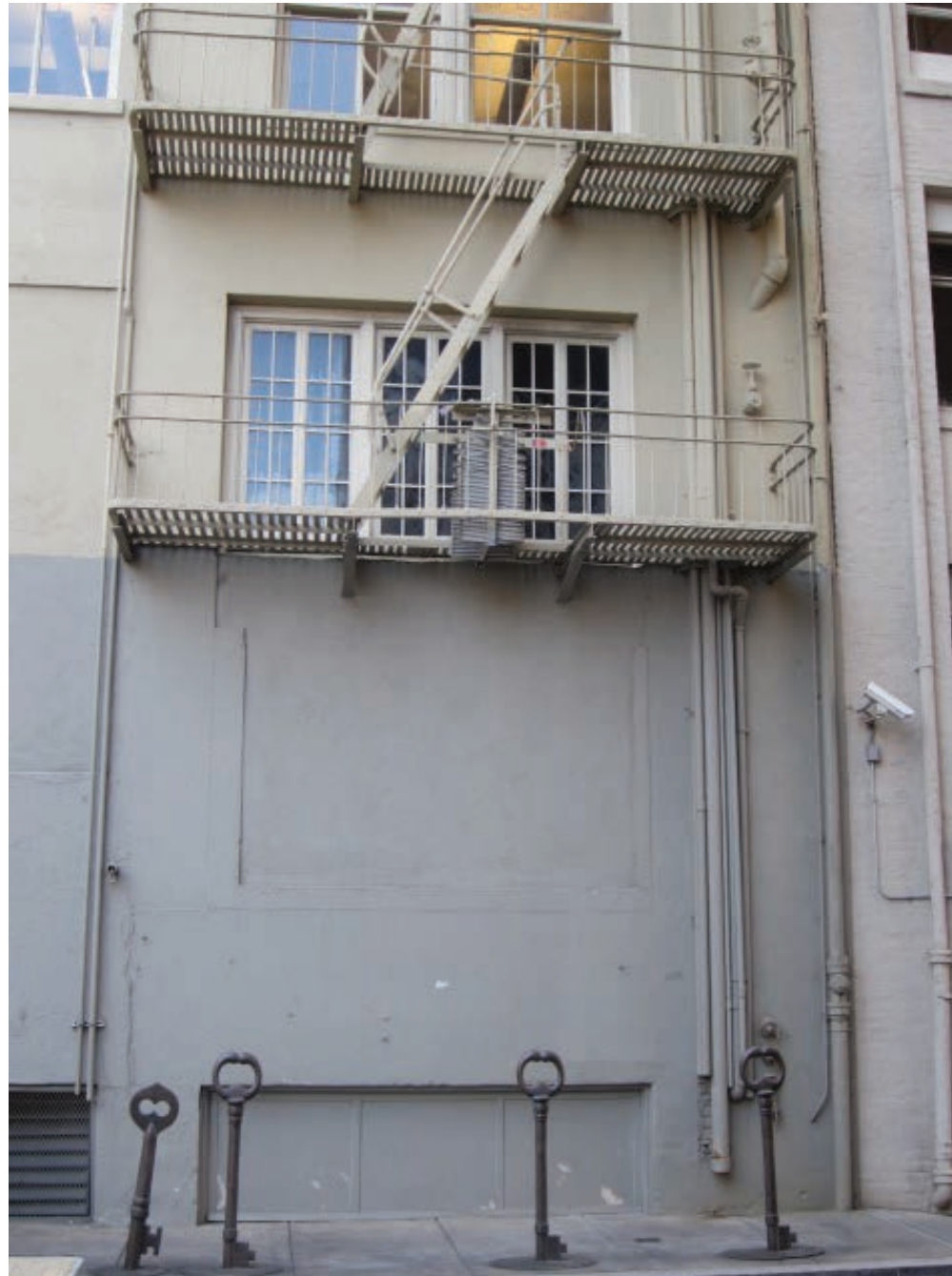
LEVEL 1 WINDOWS - EAST END
