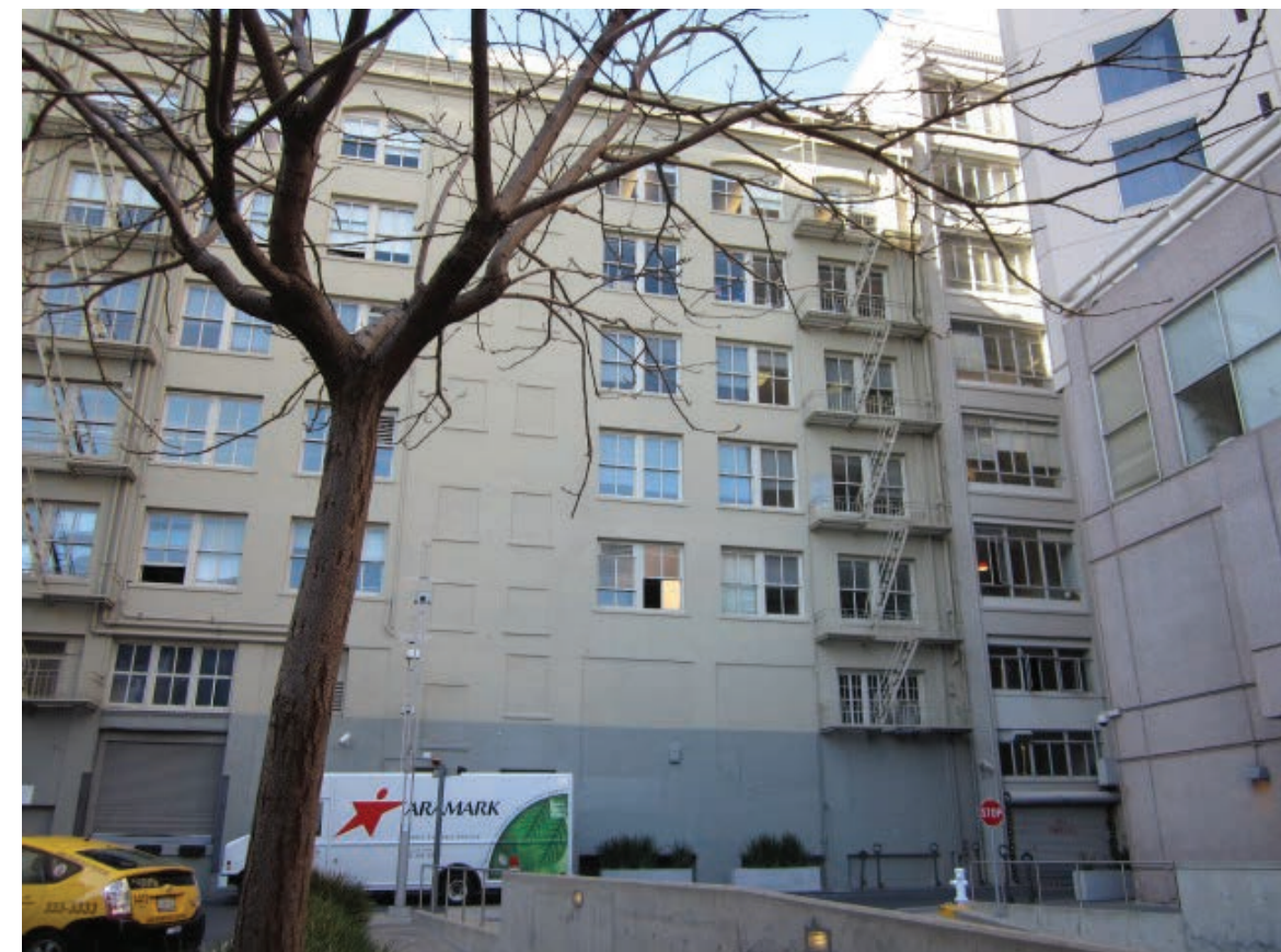
SOUTH FACADE - S-E CORNER
