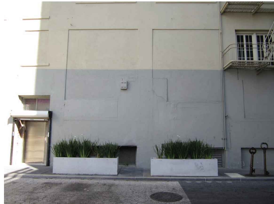
SOUTH FACADE - DETAIL VIEW 01
