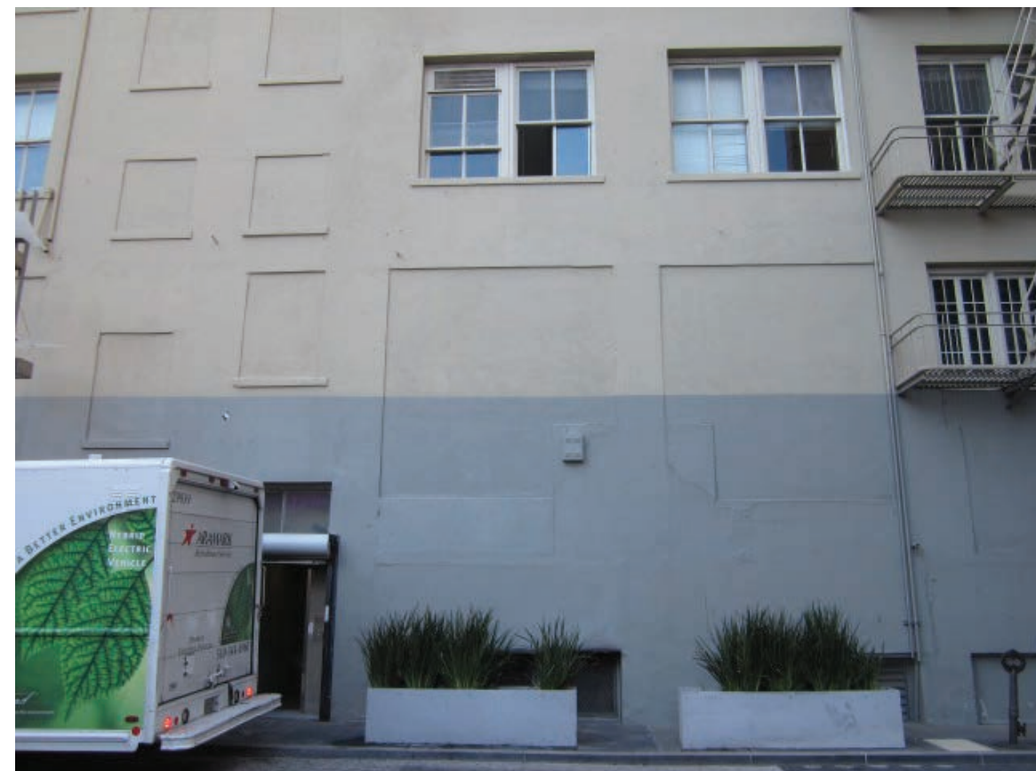
SOUTH FACADE - DETAIL VIEW 02
