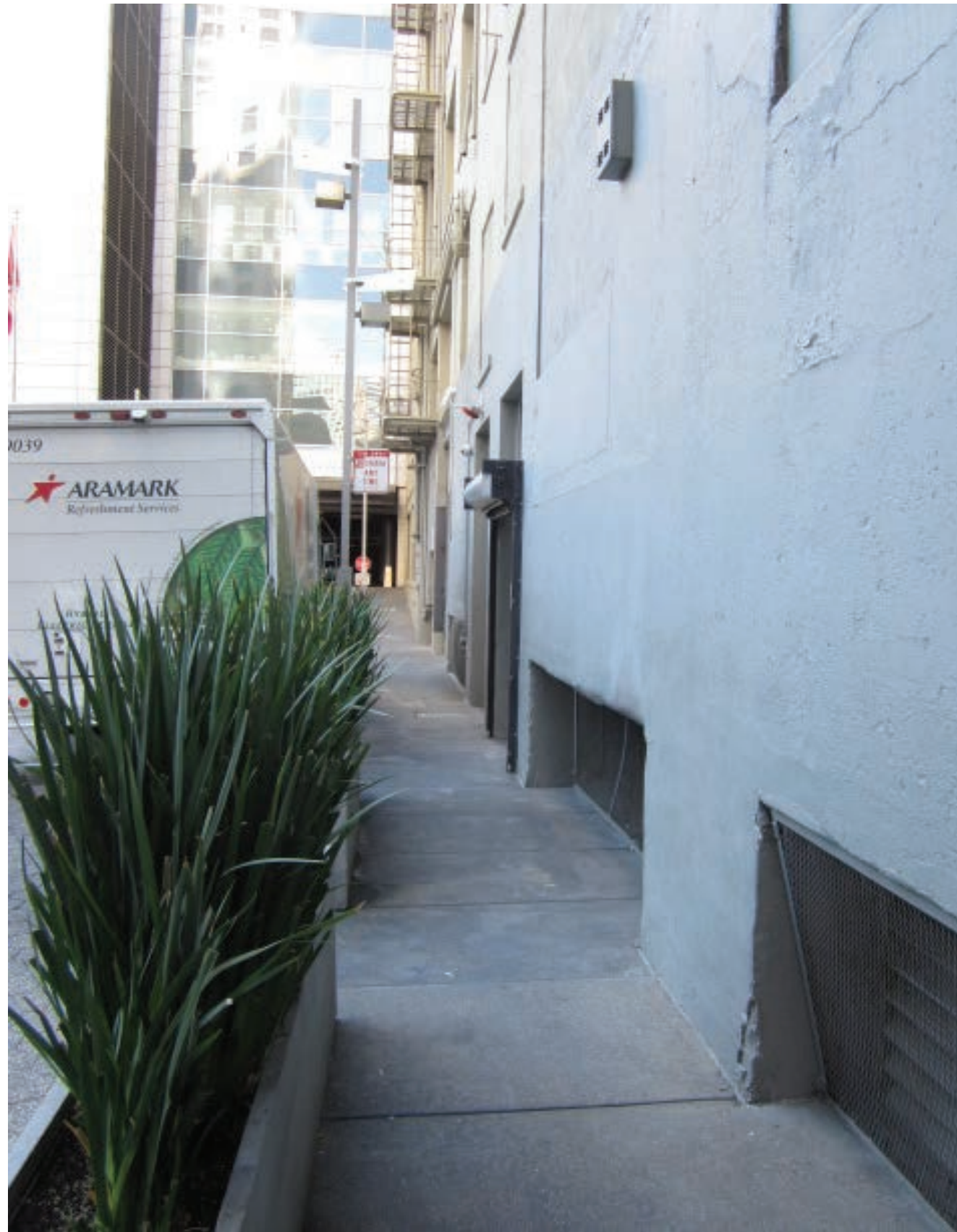
BASEMENT CLERESTORY - LOOKING WEST
