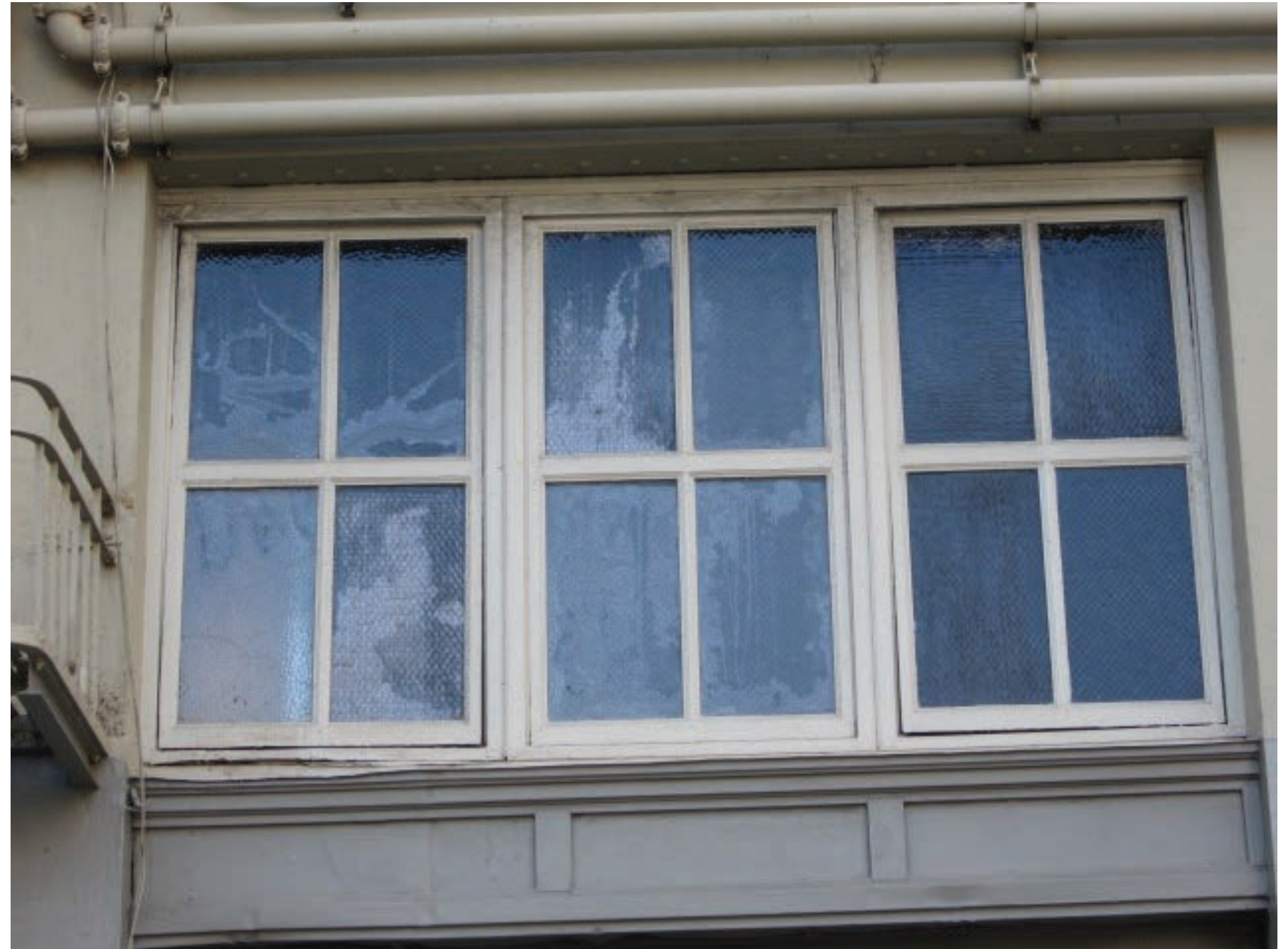
LEVEL 1 WINDOWS - DETAIL
