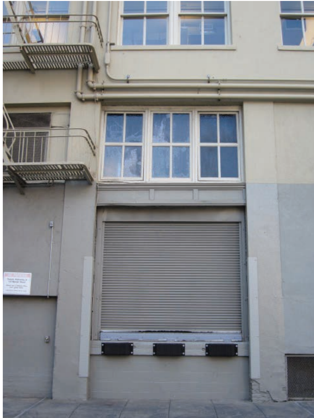
LEVEL 1 WINDOWS - WEST END
