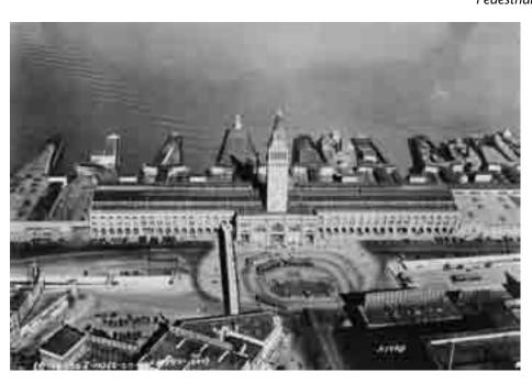
View of historic intermodal terminal, showing the vehicular subway, the transit turnaround and the elevated pedestrian bridge and multiple ferry slips, 1930s
