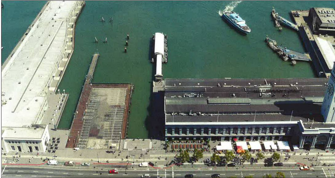
Oblique View North Basin, Showing Existing Conditions (facing east)
