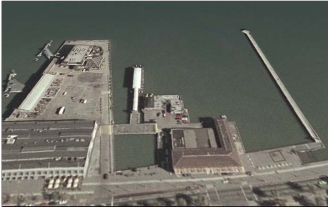
View of South Basin, Showing Existing Conditions (facing southeast)
