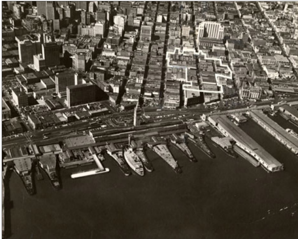
Oblique Aerial View of the Project Area (Ferry Building at Center) 1954
