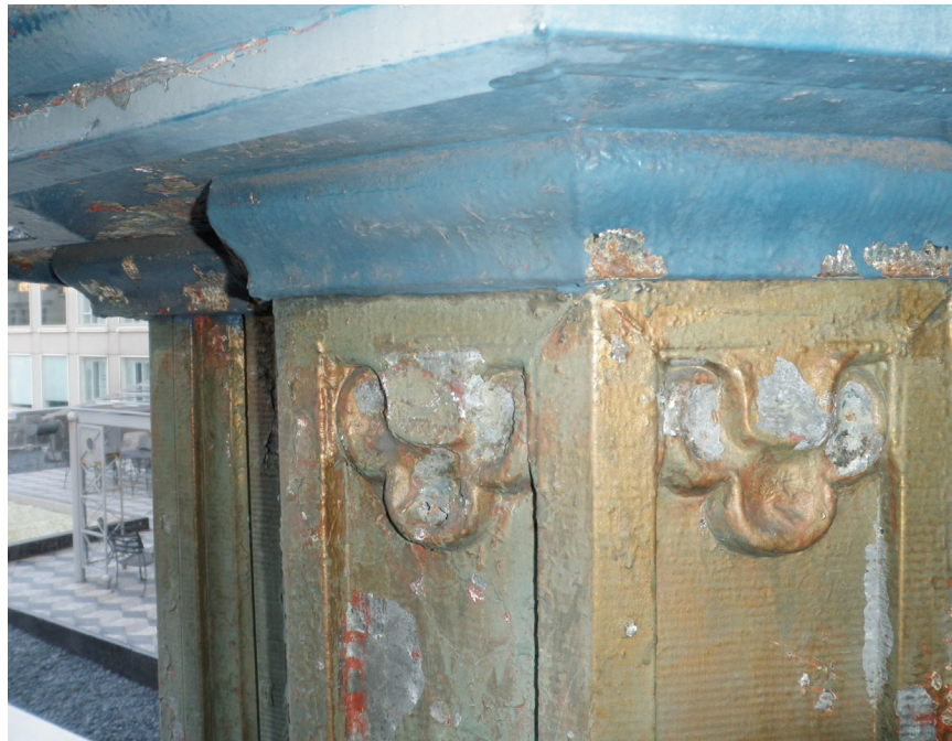
Florets on pendant prior to repairs
