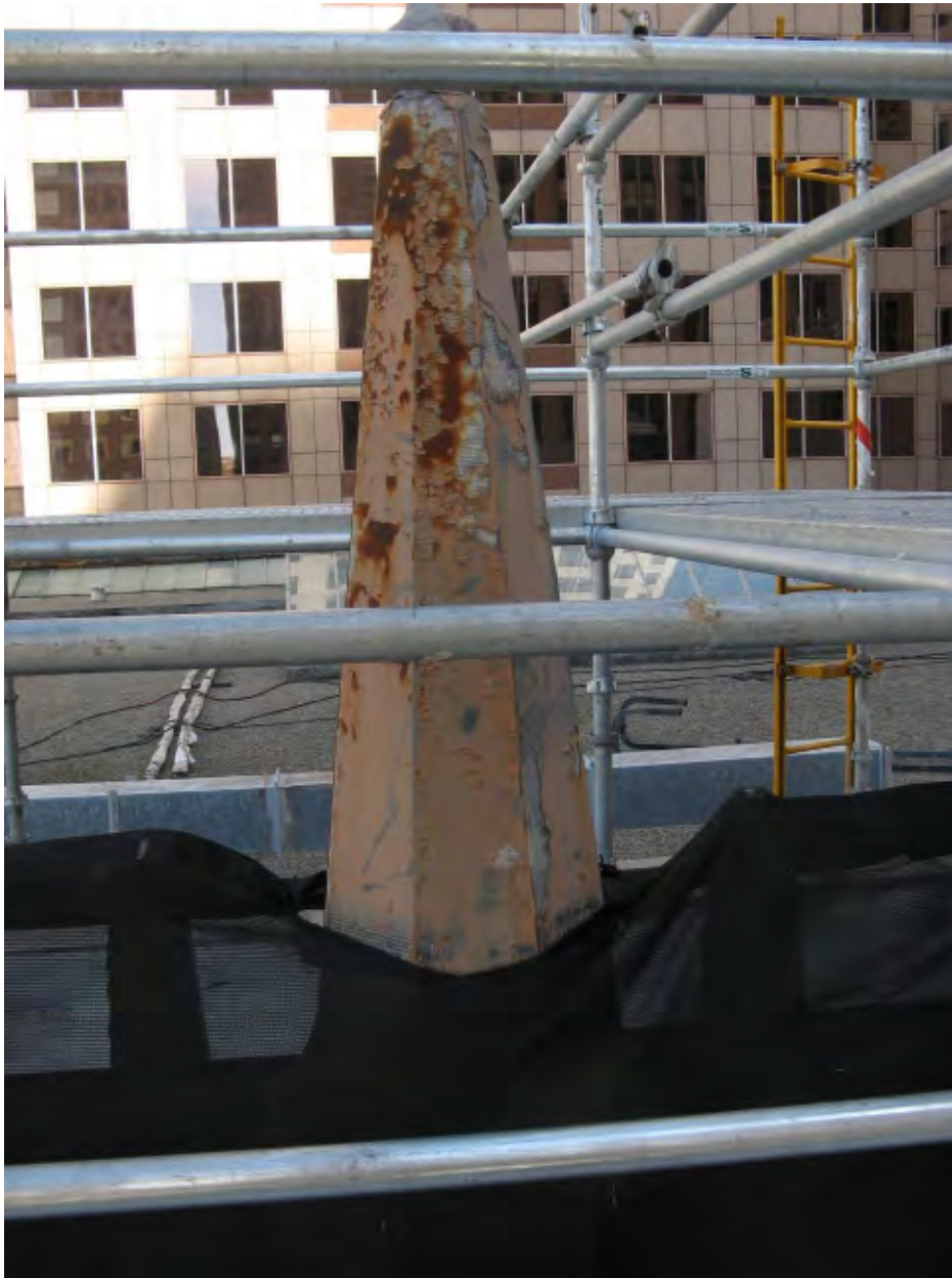
Figure 4: Spire at cornice showing existing condition and color.
