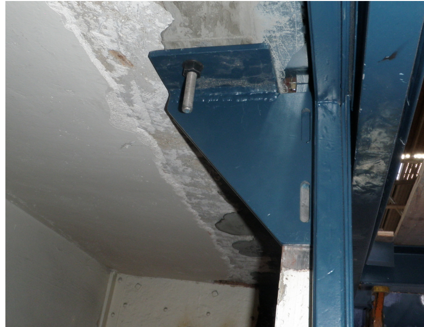
New wind anchor (Photo from Phase 1)
