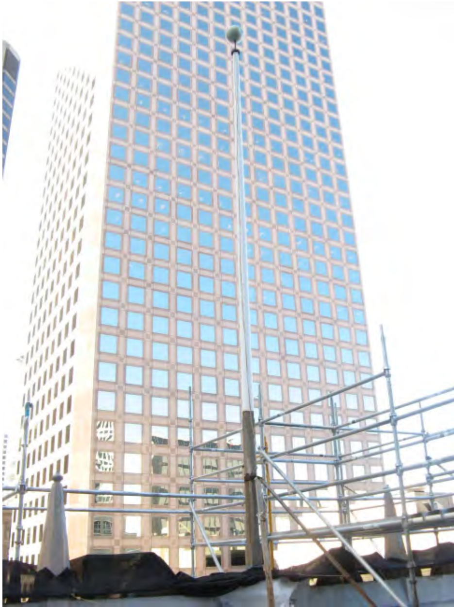
Figure 1: Hallidie Building flagpole located at roof
