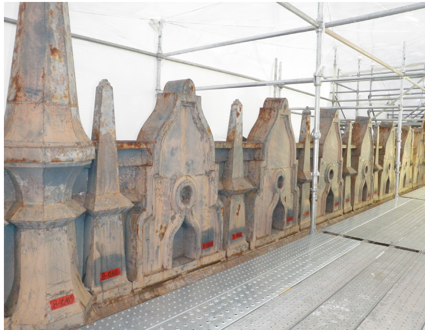
Roof cornice prior to repairs
