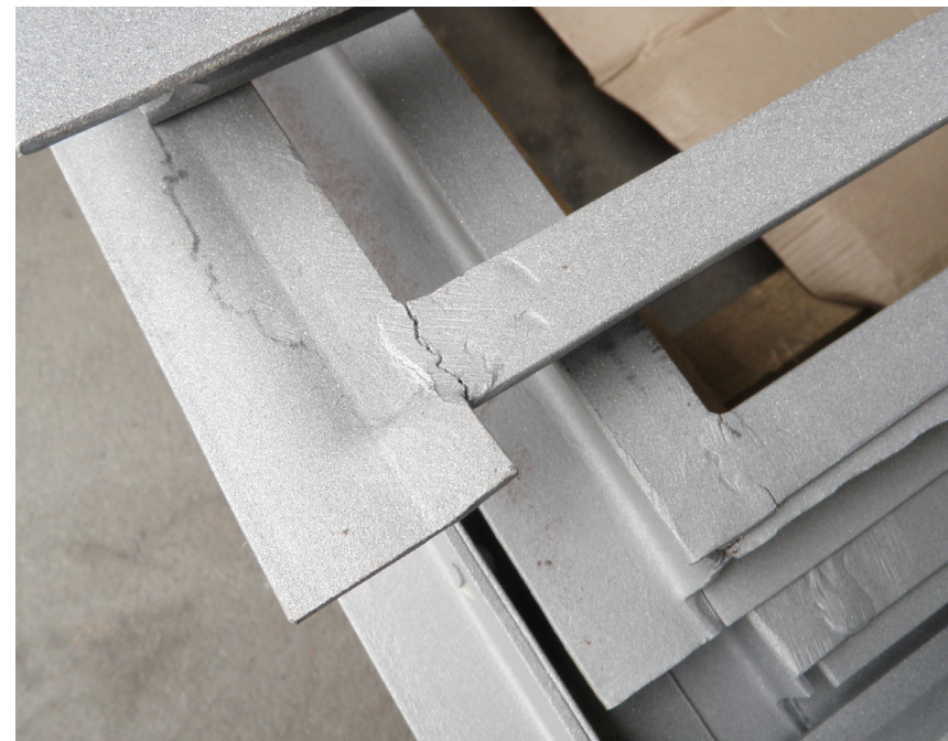
Windows during repairs
