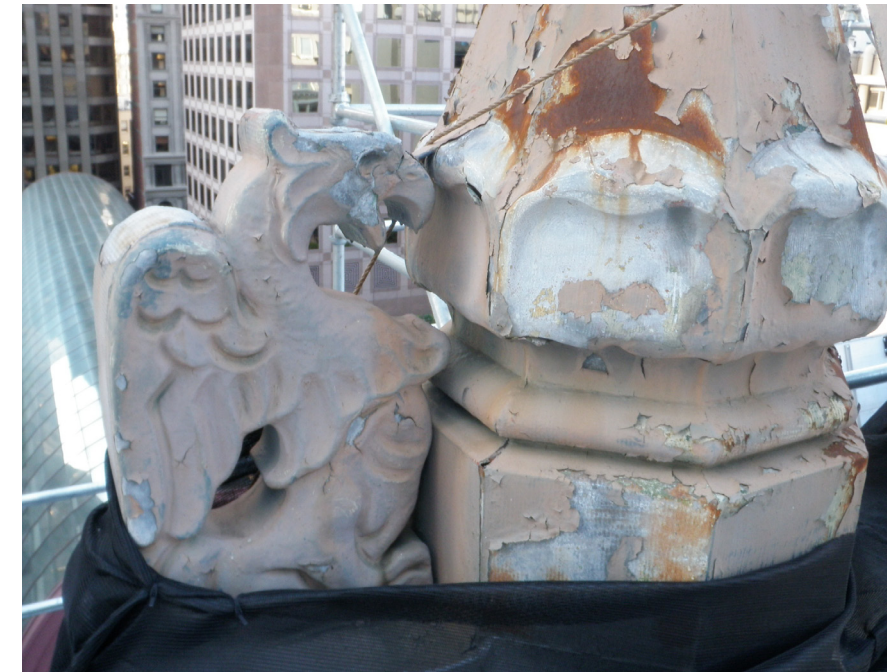
Griffin prior to repairs
