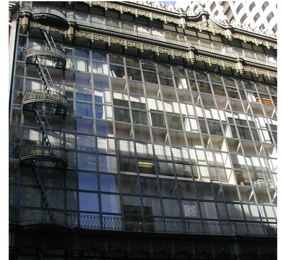
Photo of curtain wall prior to Phase 1
