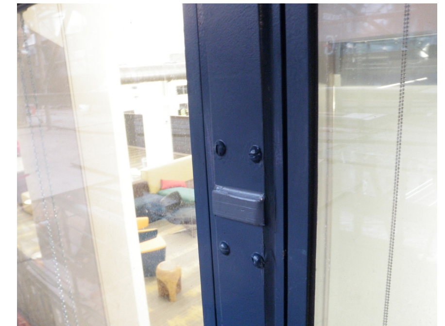
Splice at cover plate (photo from Phase 1)
