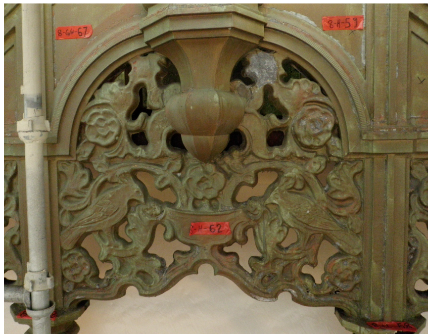
Frieze panel prior to repairs
