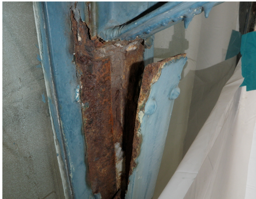
Vertical plate, prior to repairs
