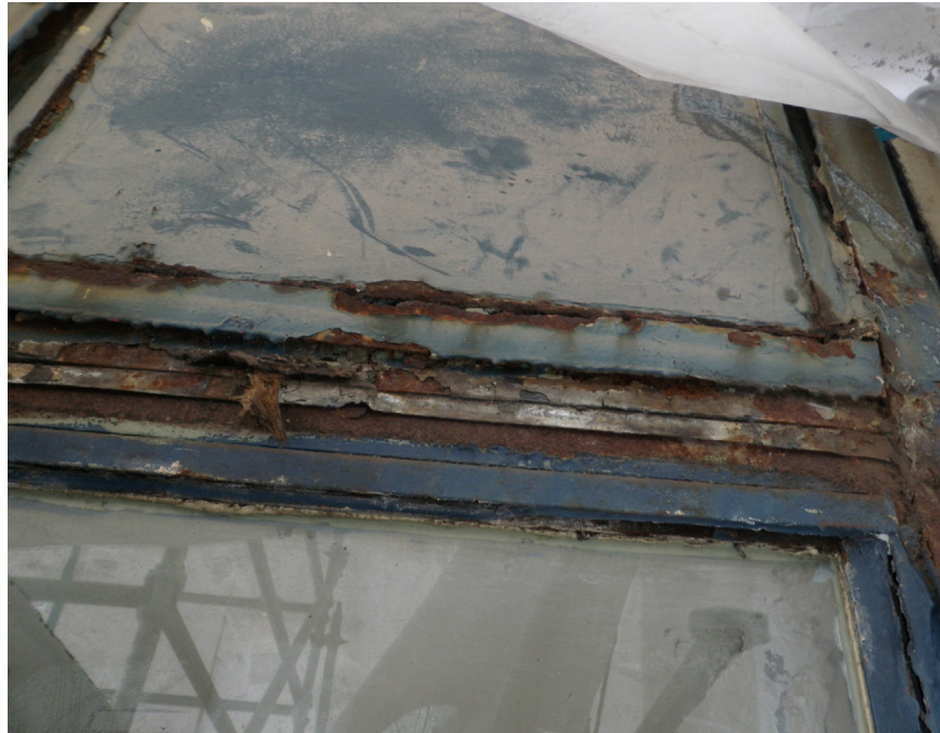
Windows prior to repairs
