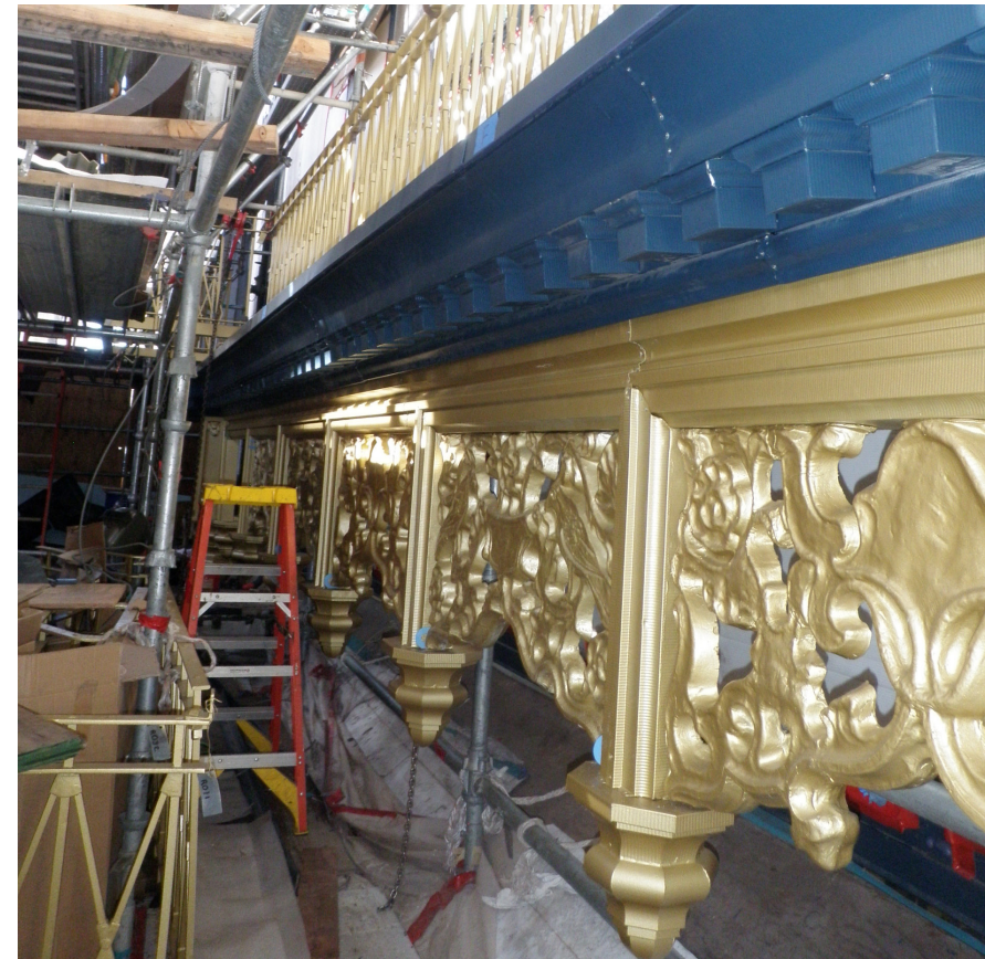
Current Repairs: Reinstallation of frieze panels and railings at second floor
