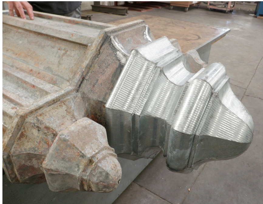
Replacement pendant, note striated surface
