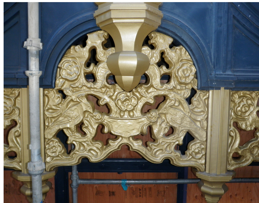
Frieze panel, repaired and installed
