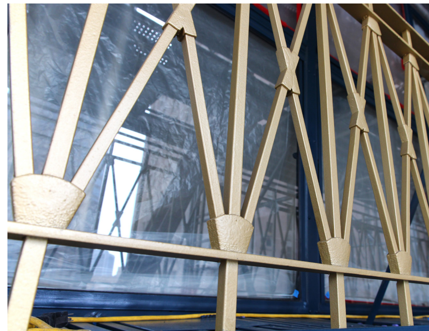
Replacement railing brackets ("bow ties")
