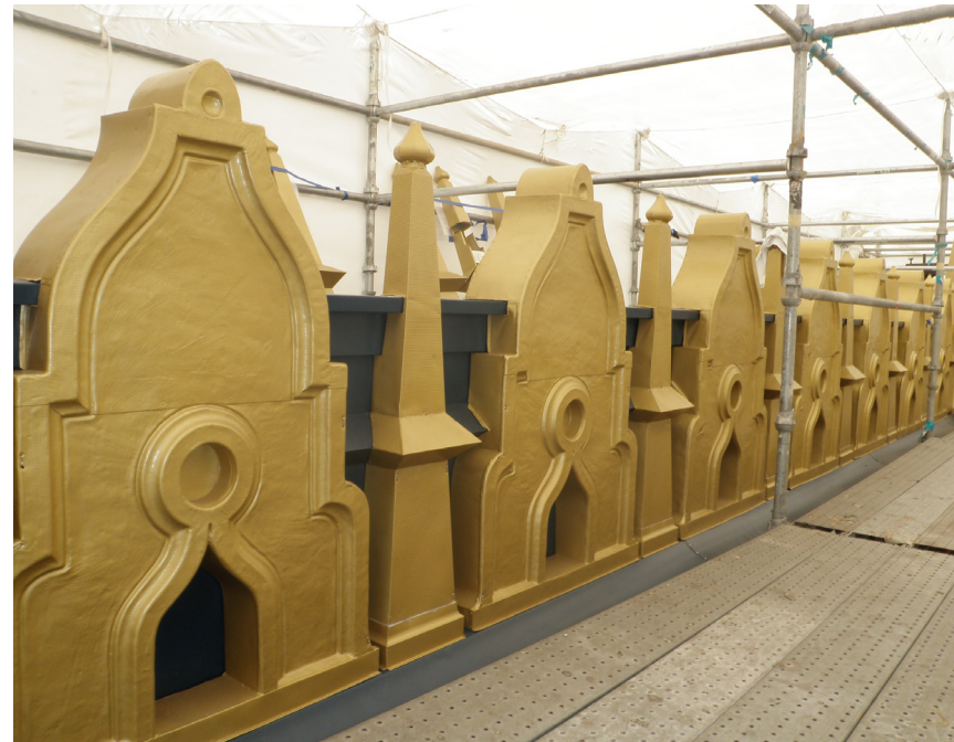
Roof cornice after repairs
