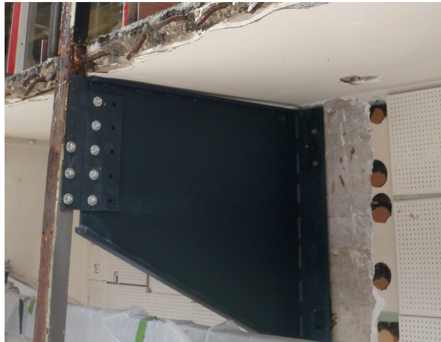
New bearing anchor (Photo from Phase 1)
