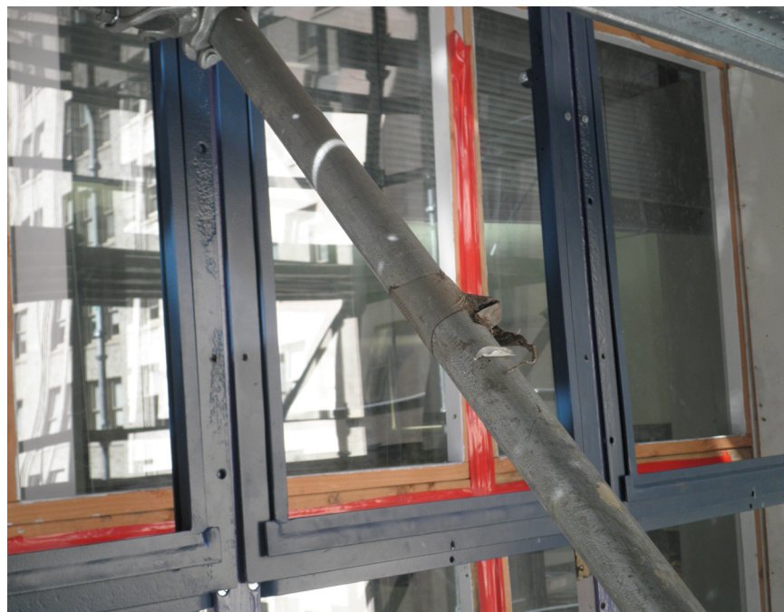
Windows during installation
