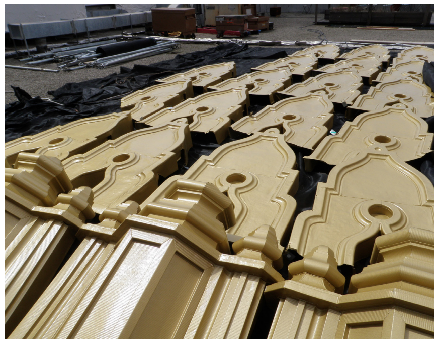
Roof cornice elements after repairs
