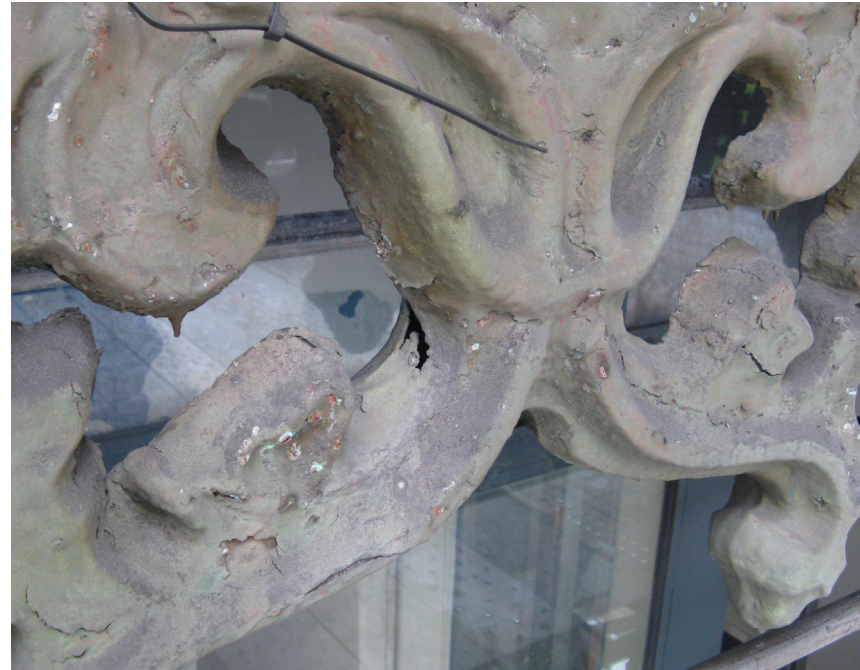
Frieze panel prior to repairs
