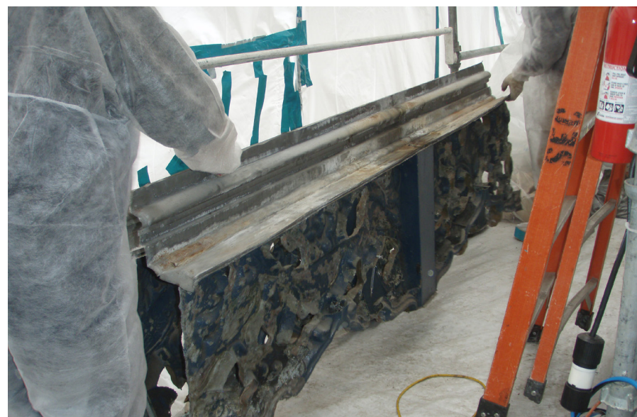
Decorative sheet metal is being removed where there are existing seams
