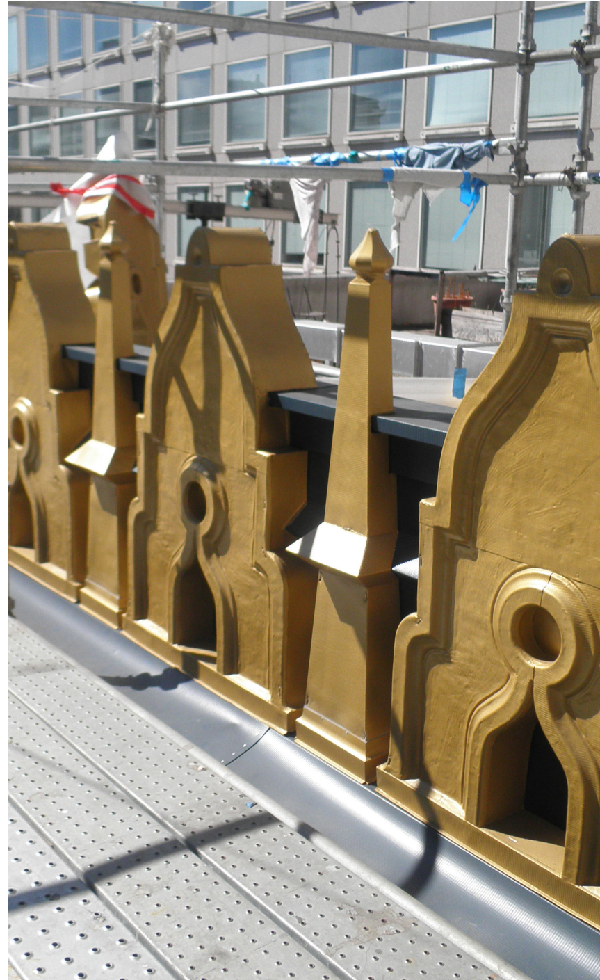
Roof cornice spires after repairs
