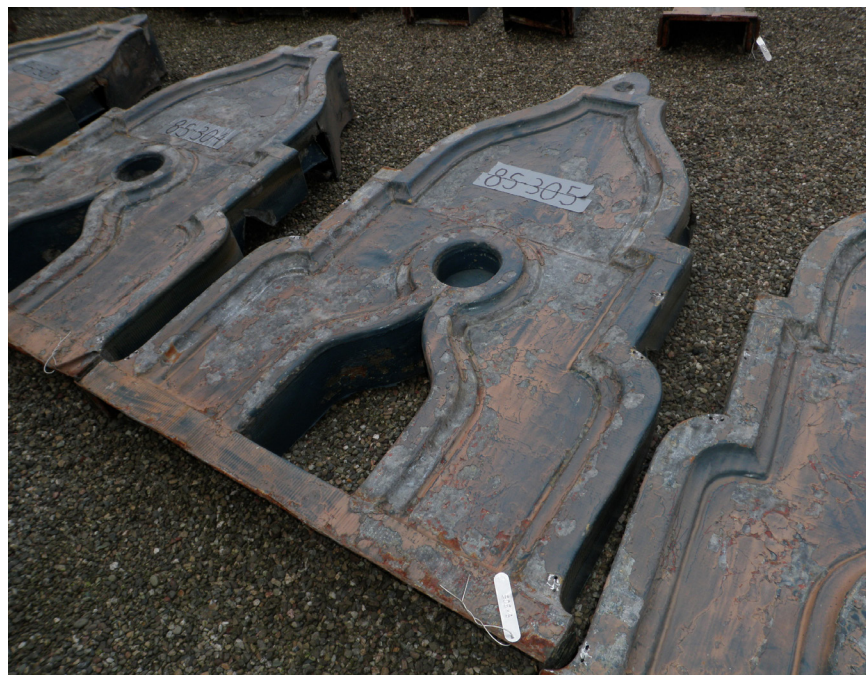
Roof cornice elements prior to repairs
