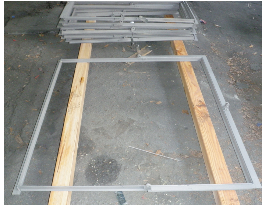
Windows during repairs
