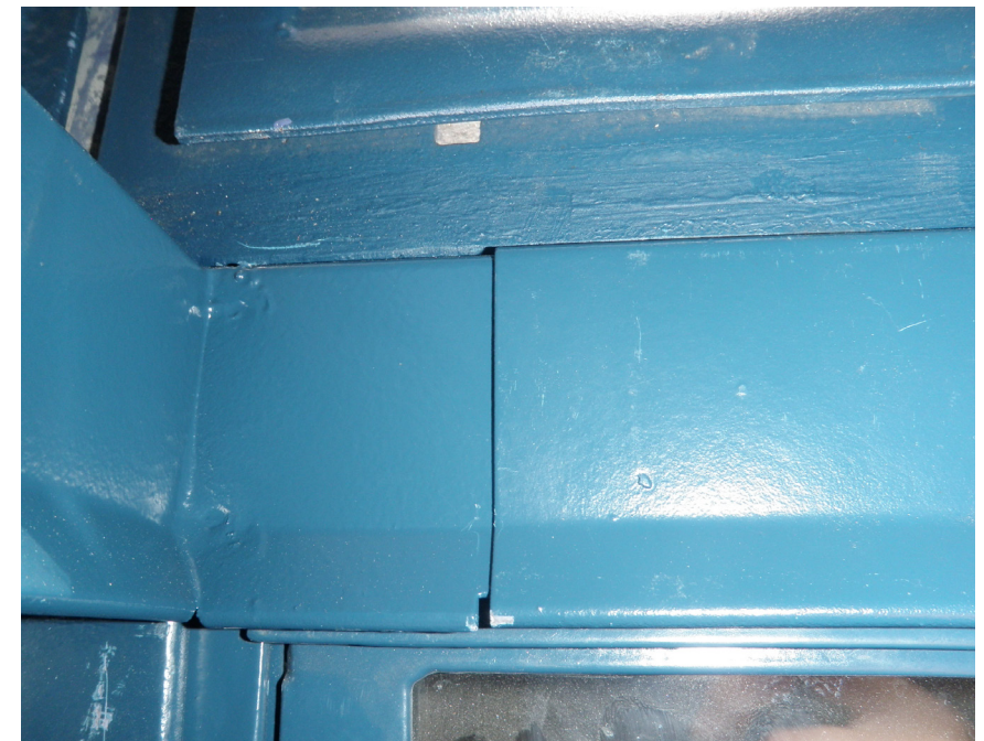
Flashing at windows aligned with balconies and fire escapes
