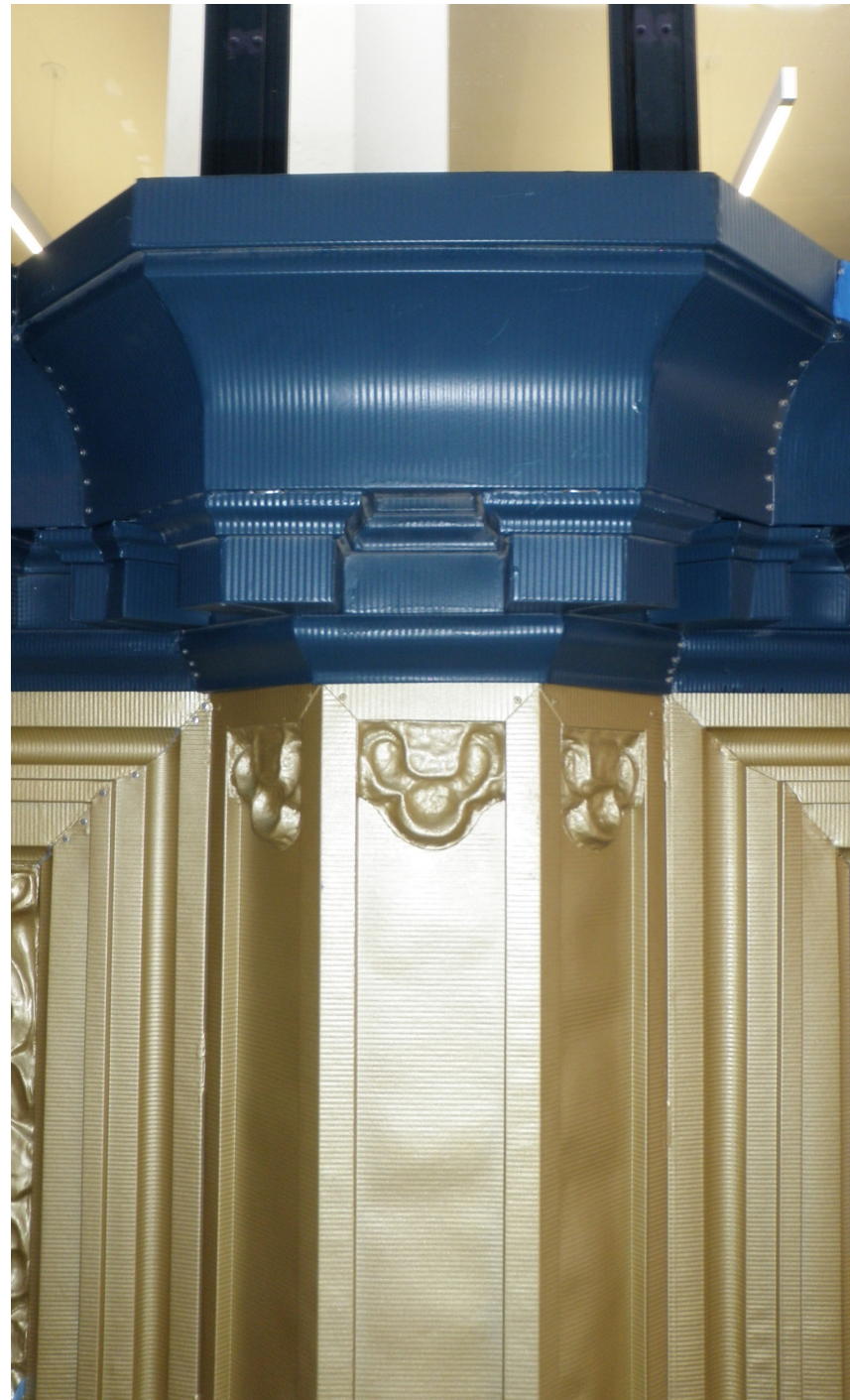
Florets on pendant, installed
