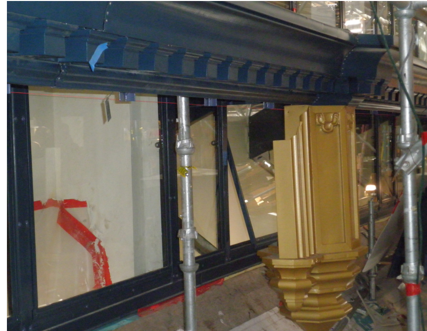
Large pendant, repaired and installed
