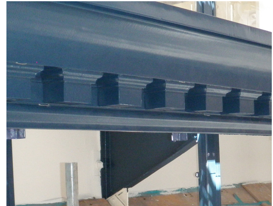
Dentils after repairs
