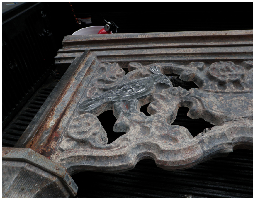
Frieze panel prior to repairs
