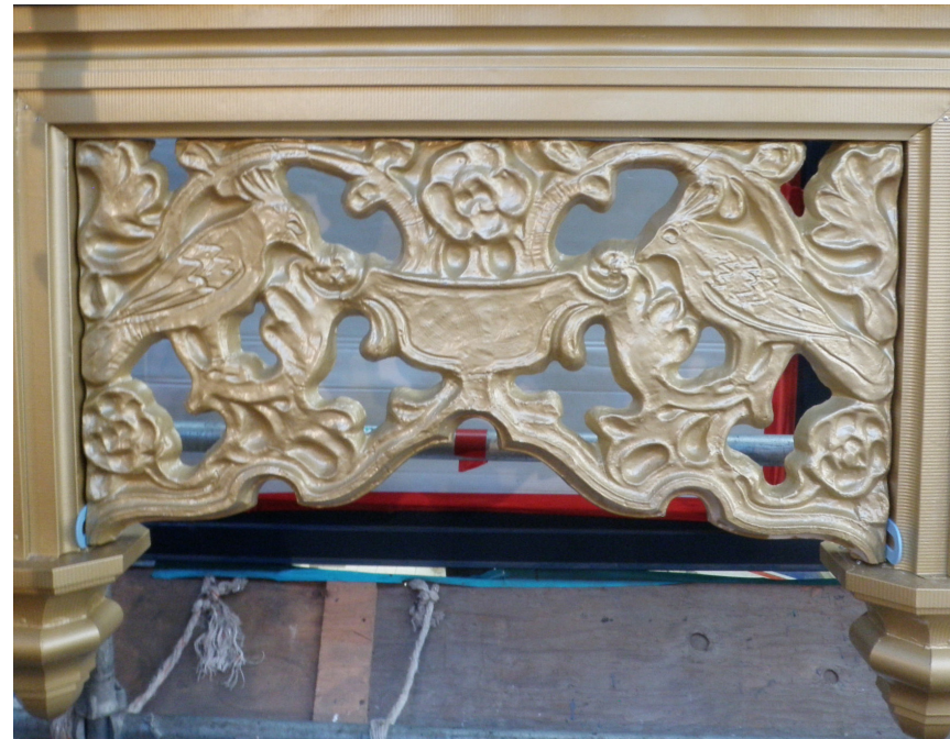
Frieze panel, repaired and installed
