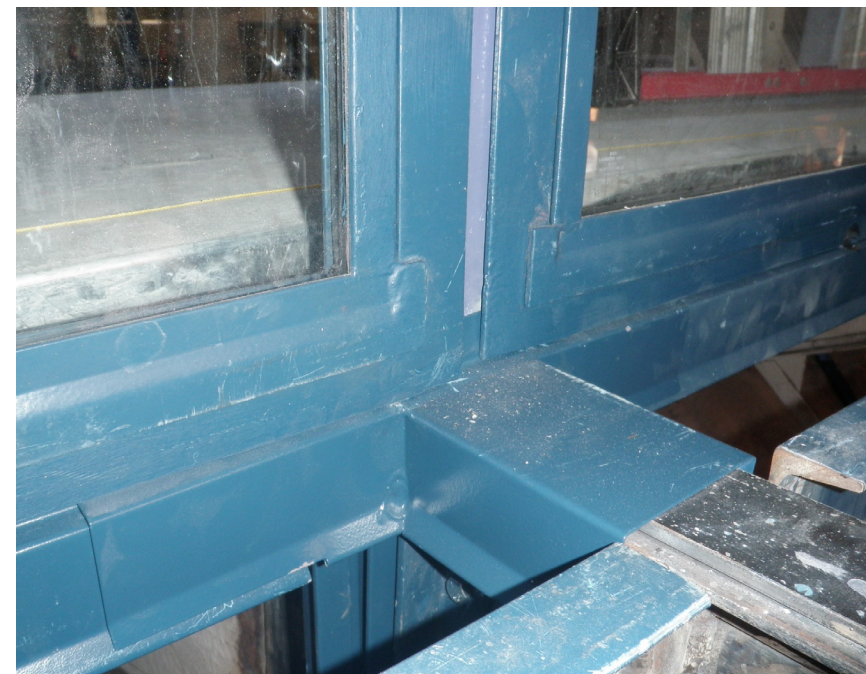
Saddle flashing at outrigger I-Beam
