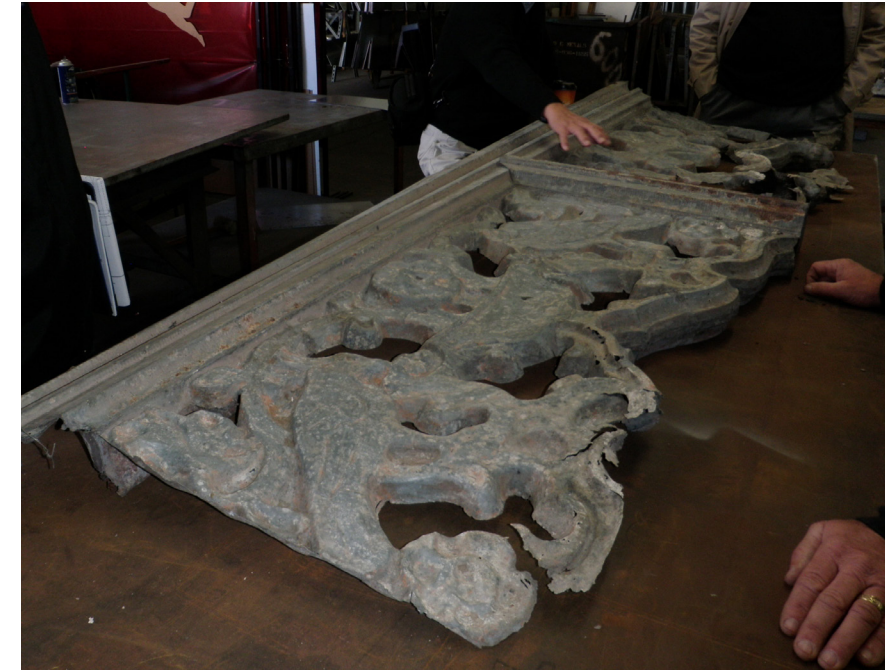
Frieze panel prior to repairs
