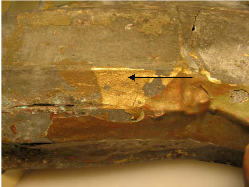
Figure 4: Detail of metal tracery showing historic gold leaf gilding revealed under later paint layers. The gold leaf was applied over a thin red clay bol preparatory layer.
