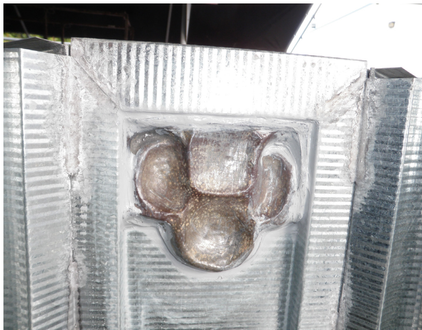
Florets on pendant, stripped, prior to painting
