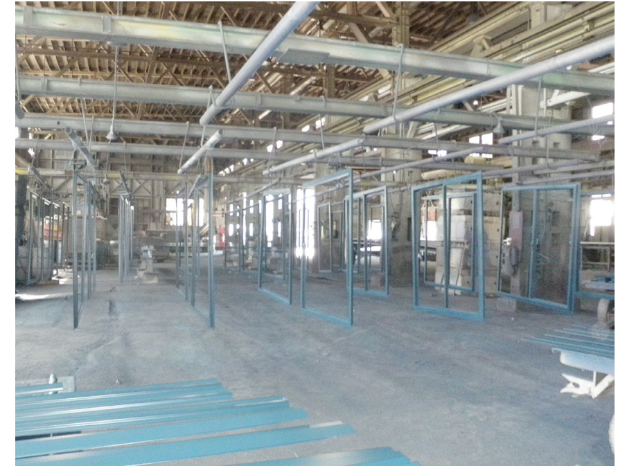
Windows during repairs
