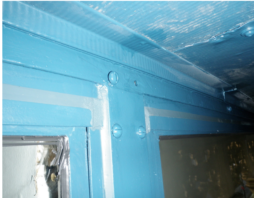
Soffit at 7th floor windows
