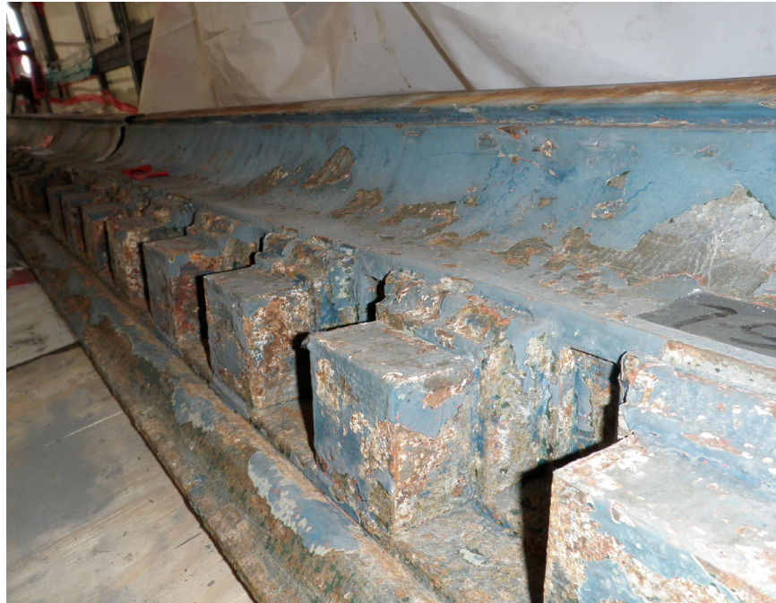
Dentils prior to repairs
