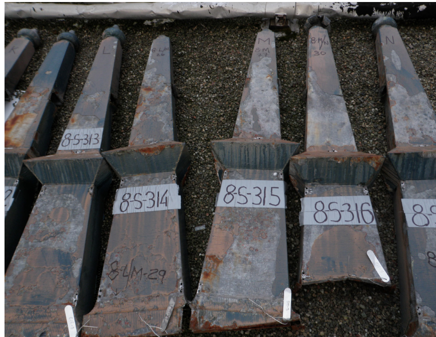
Roof cornice spires prior to repairs
