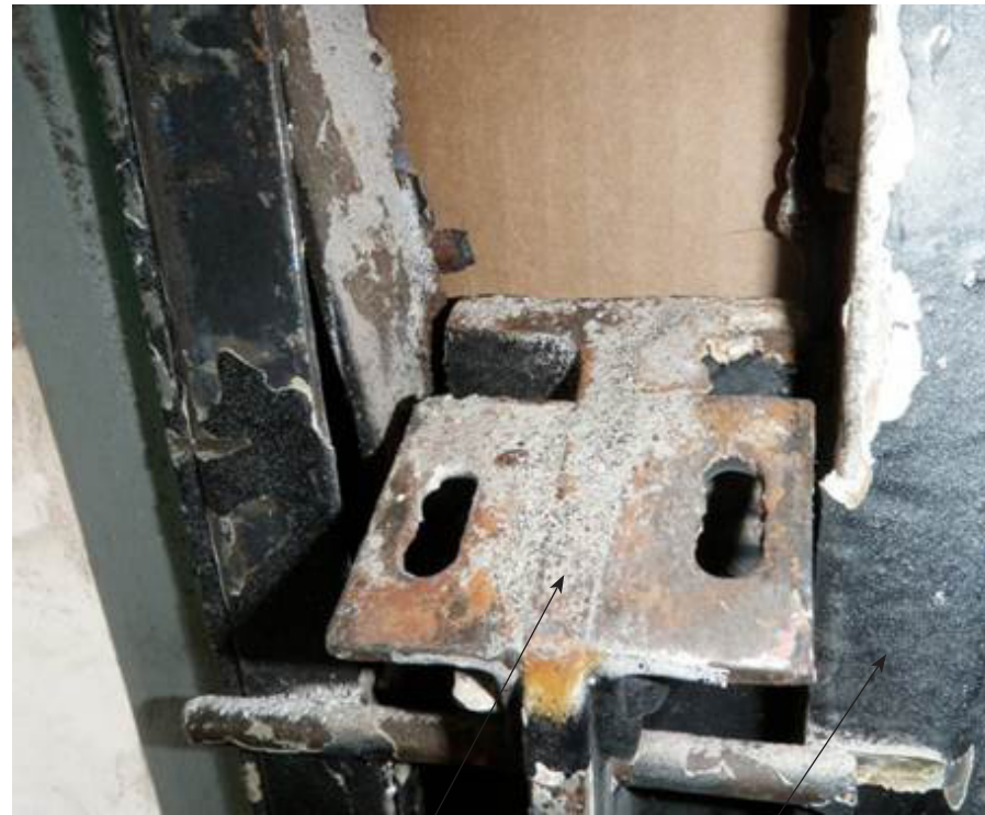
existing T-mullion at vertical spans of curtain wall existing windows on each side
