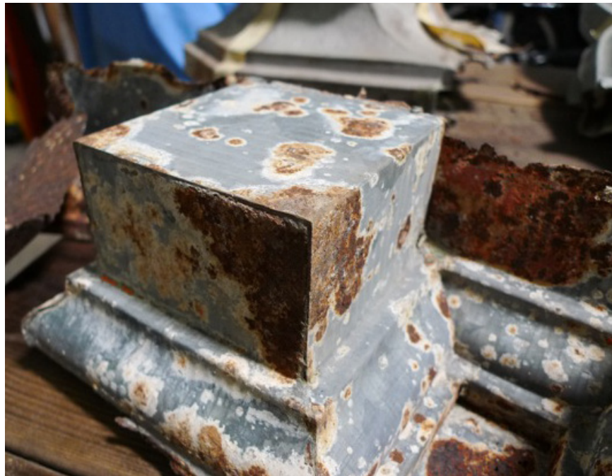
Dentils prior to repairs
