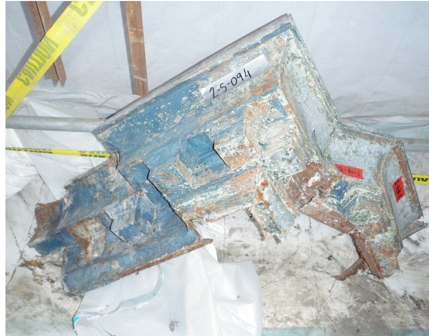
Dentils prior to repairs
