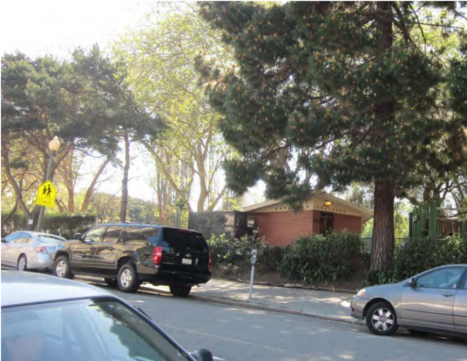
FILBERT STREET FACADE
