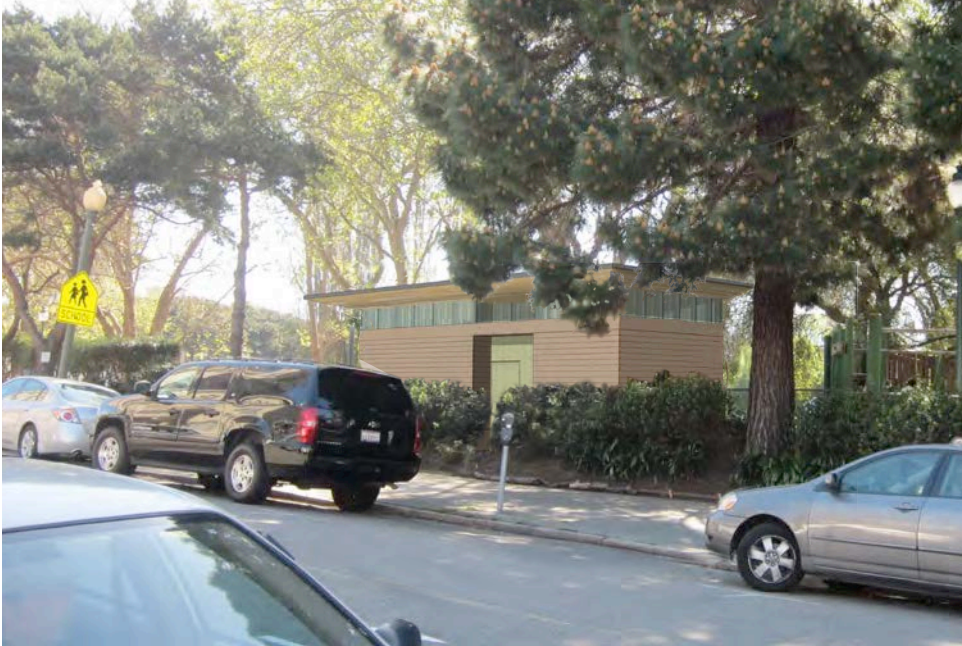
FILBERT STREET FACADE
