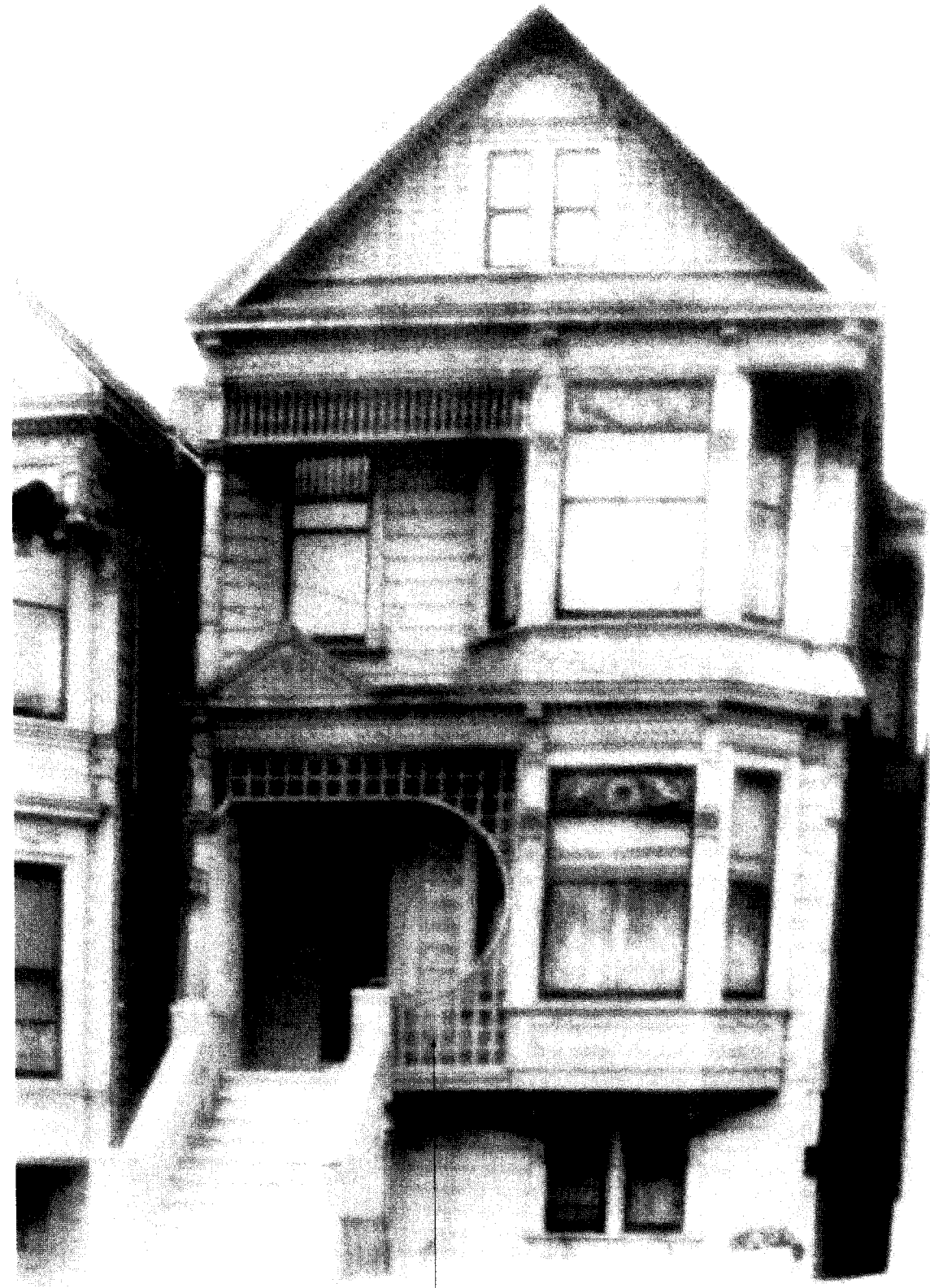
HISTORIC PHOTO OF FRONT FACADE WITH ORIGINAL P.G. 'TRELLIS' ORNAMENTATION AT STOOP
