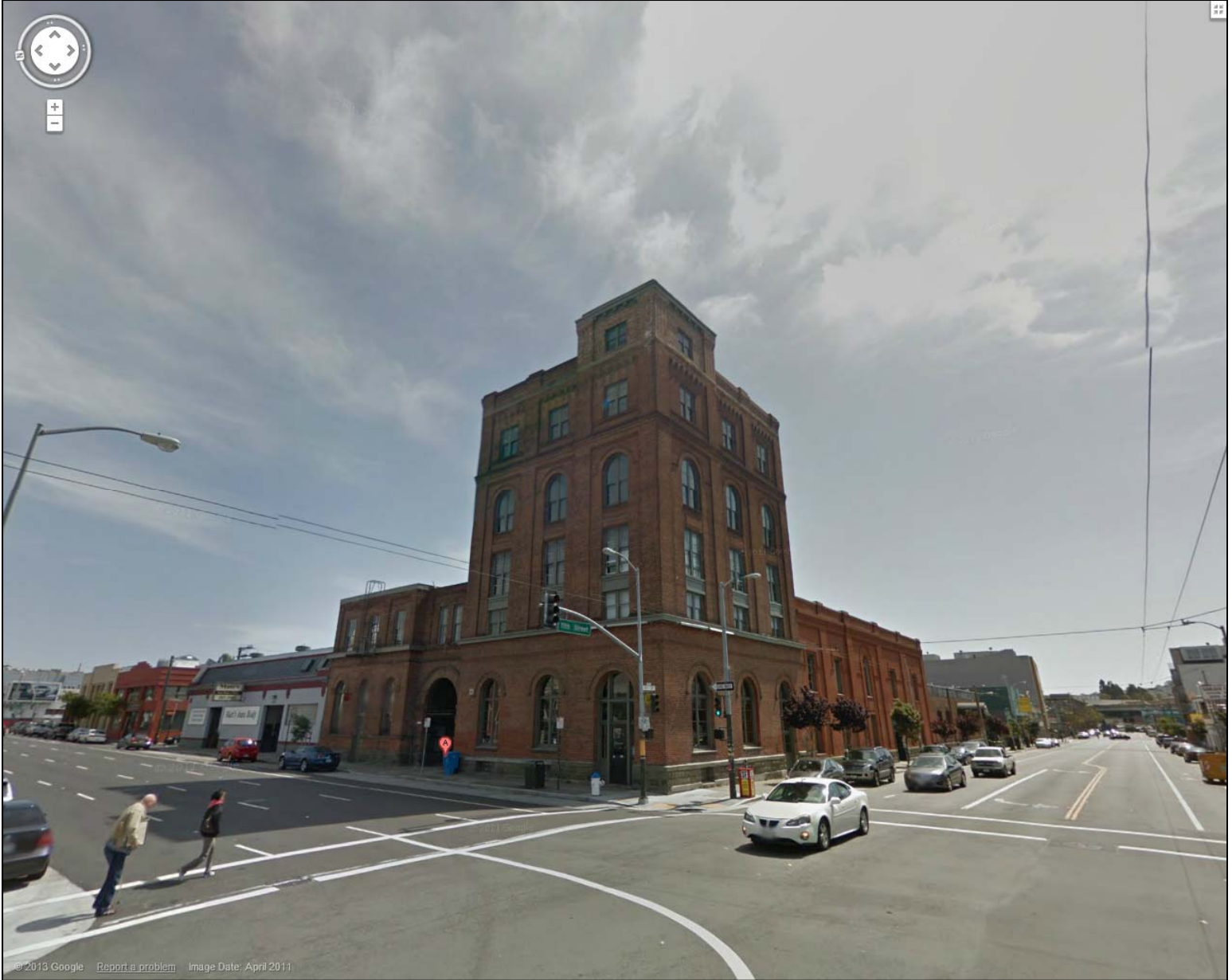
1475-1479 Folsom Street, View of Folsom and 11 th Streets (Source: Google Maps, Accessed February 11, 2013; Image Date March 2011)
