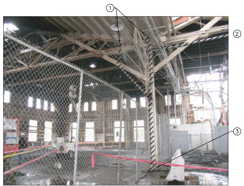
DEMOLITION PHOTO NTS 1 P1.1|P3.2
