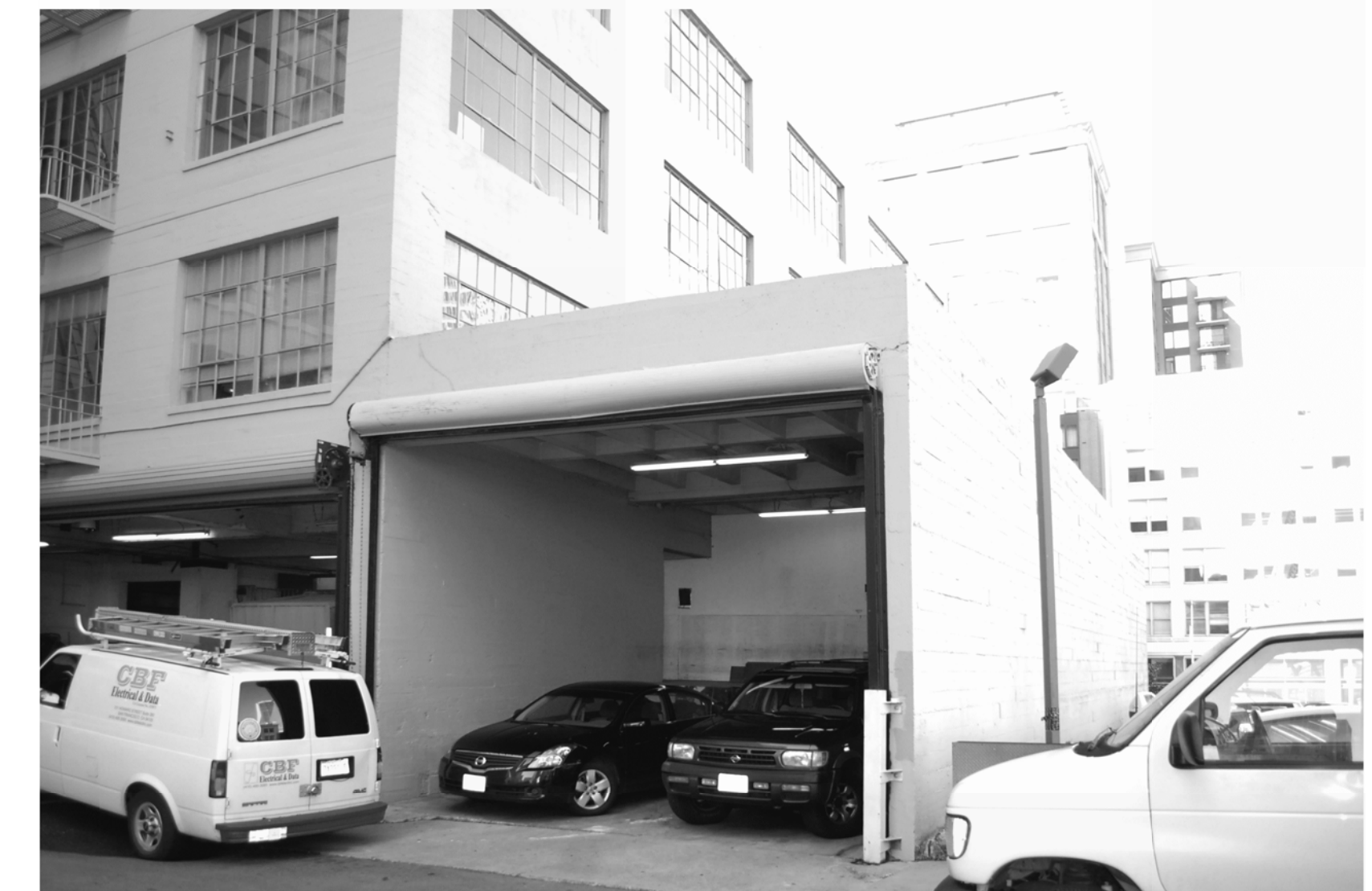
EXTERIOR VIEW AT LOADING DOCK
