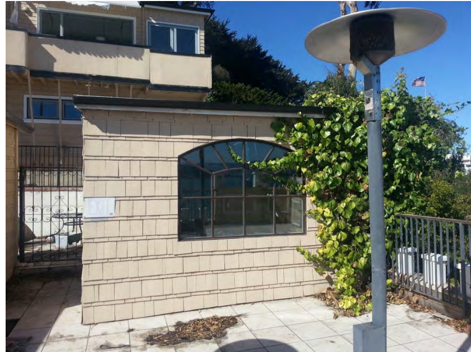
Figure 14 - East side of detached structure, existing window (to be replaced)
