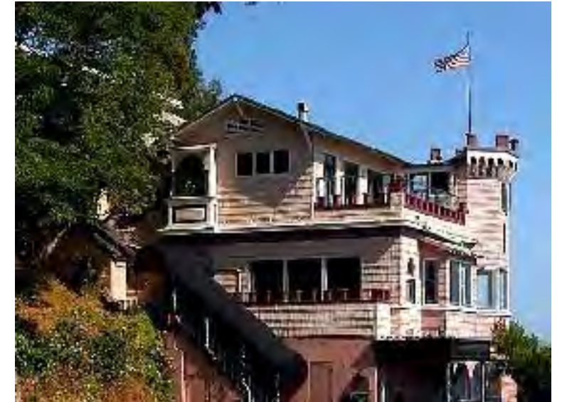
Figure 5 - Building before non-permitted changes (circa 2000)
