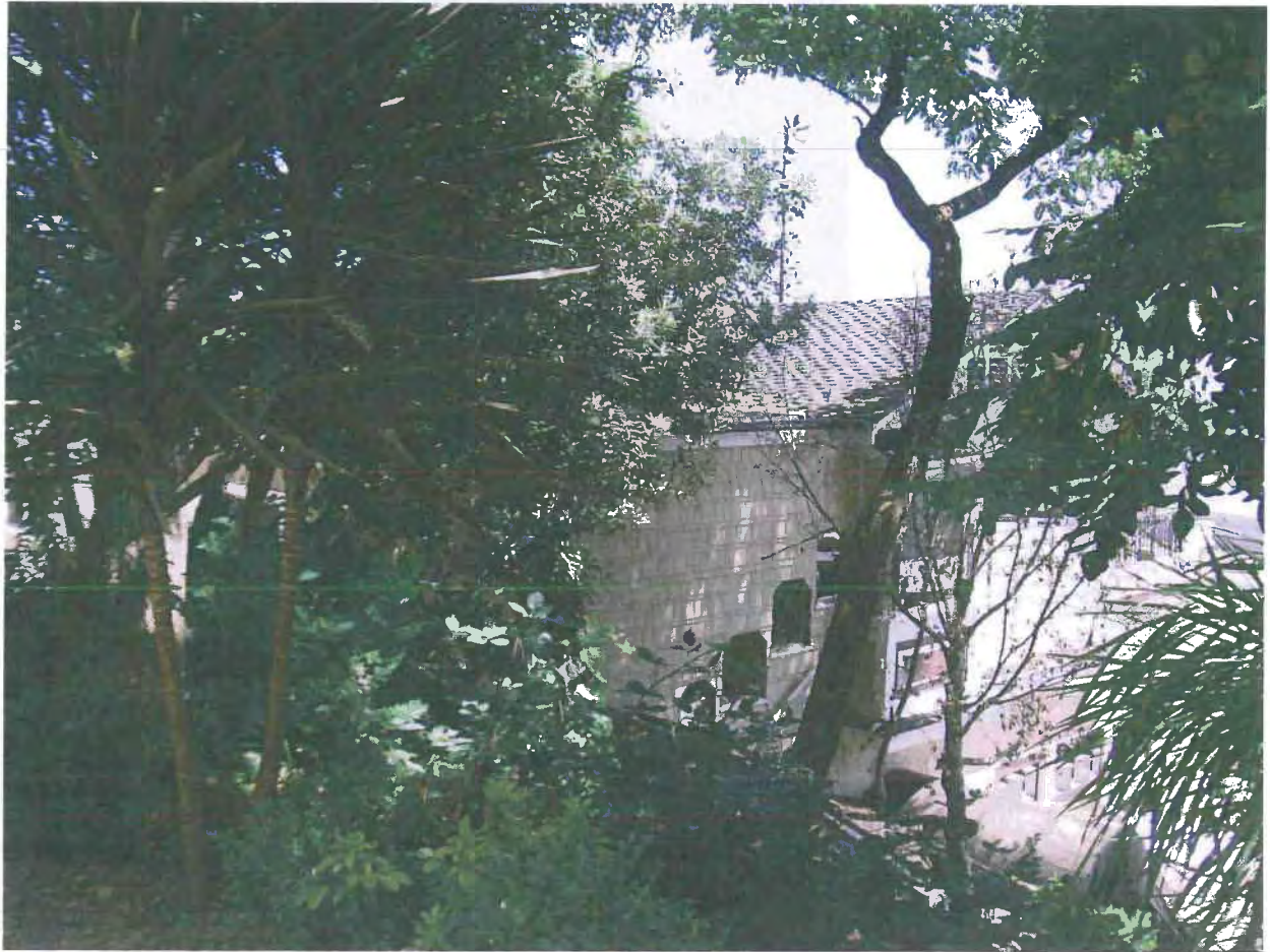
D: 302 Greenwich Southern Façade from Greenwich Steps
