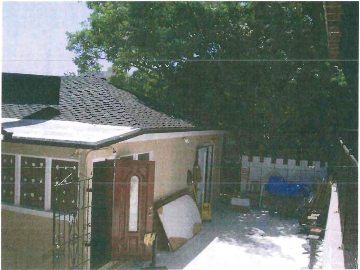
G: 302 Greenwich: New Patio Area and Addition at Southwestern Corner
