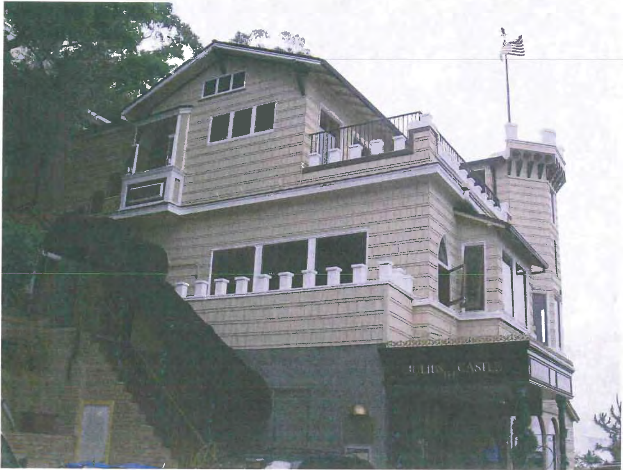
B: Southern Façade of Subject Property: From Parking Lot/Montgomery Street
