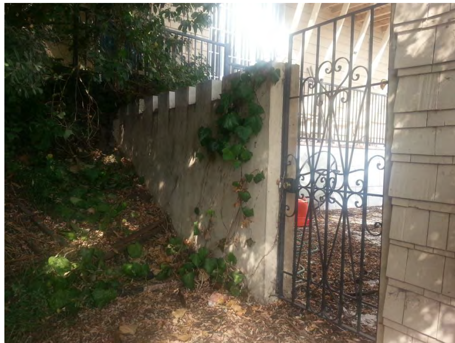
Figure 29 - Existing wall from south east perspective
