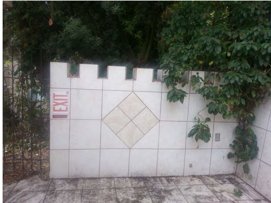
Figure 28 - Existing wall, view from courtyard from north perspective
