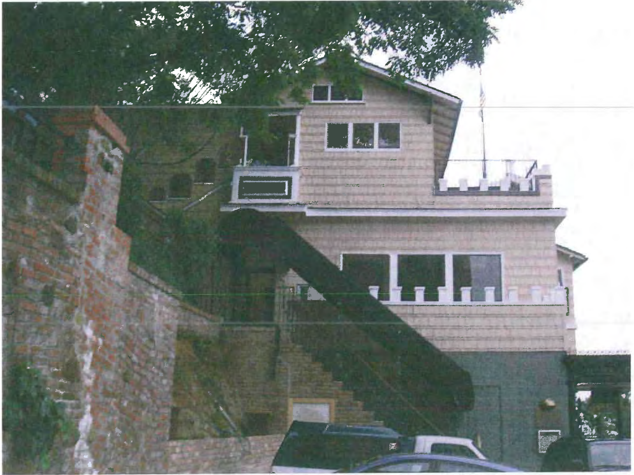
C: Southern Façade of Subject Property: From Parking Lot
