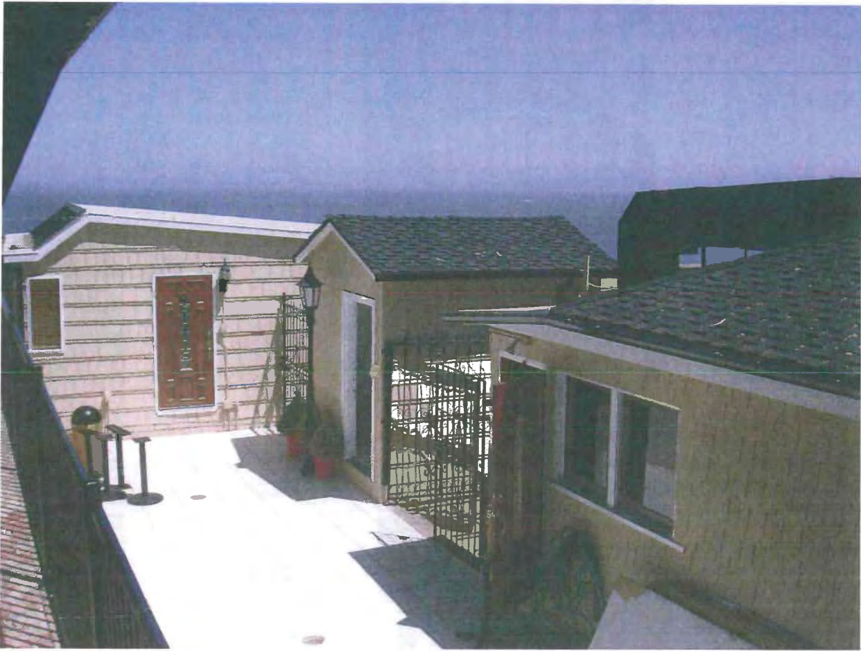
H: 302 Greenwich: New Patio and New Addition to Detached Structure at Northwestern Corner
