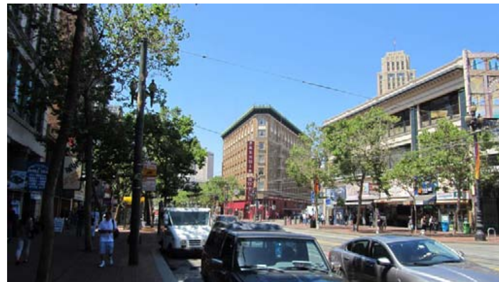
With New Roof Construction
