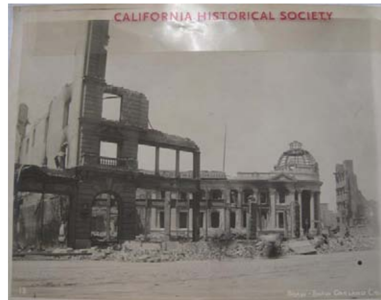
Historic Photos of 1906 Earthquake and Fire Damage Photos courtesy of SFPL & California Historical Society
