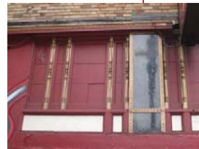
Existing Historic Storefront Transom Windows
