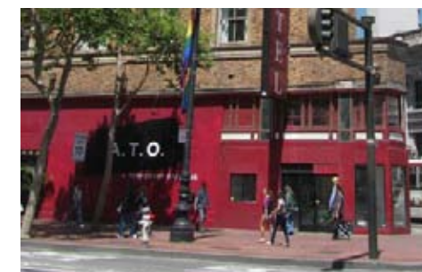
Existing Market St. Storefront
