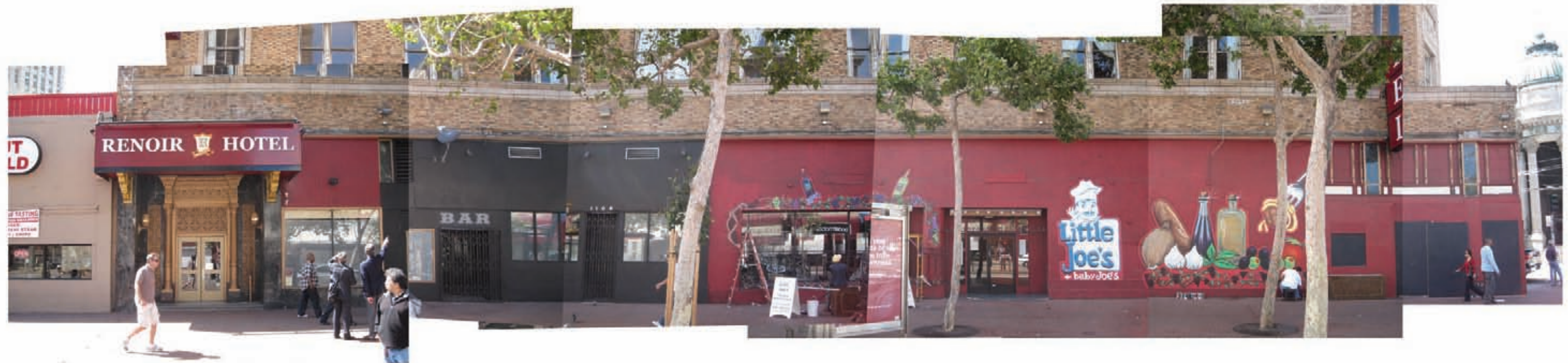
Existing Market Street Storefront
