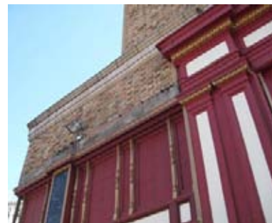
Existing Mezzanine Windows and Column Capitals
