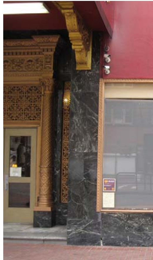
Existing Pilaster Base near Lobby Entrance Market Street
