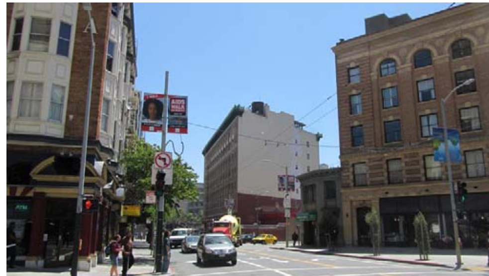
With New Roof Construction
