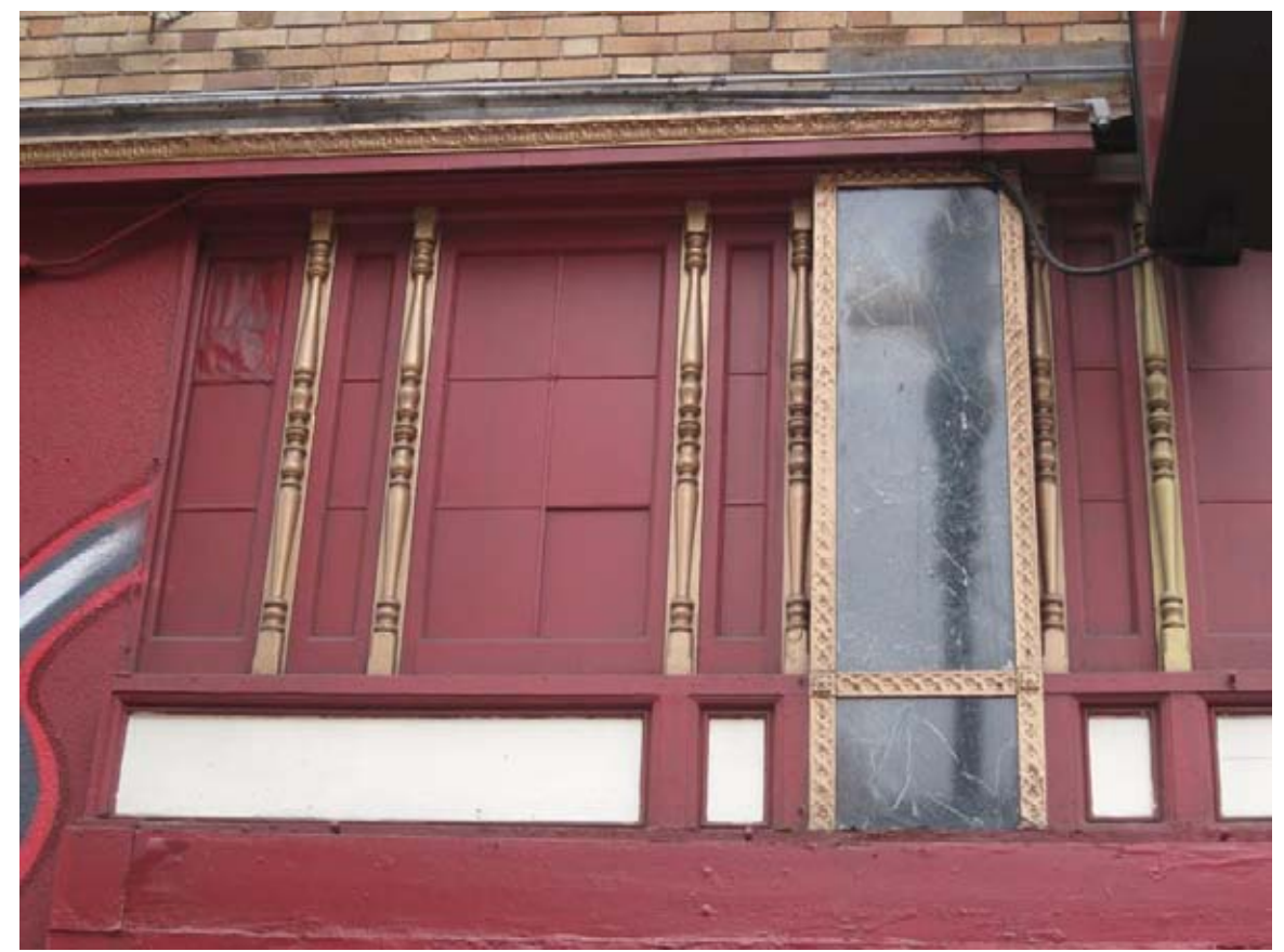
Existing Pilaster and Mezzanine Transom Windows with Spindle Market Street
