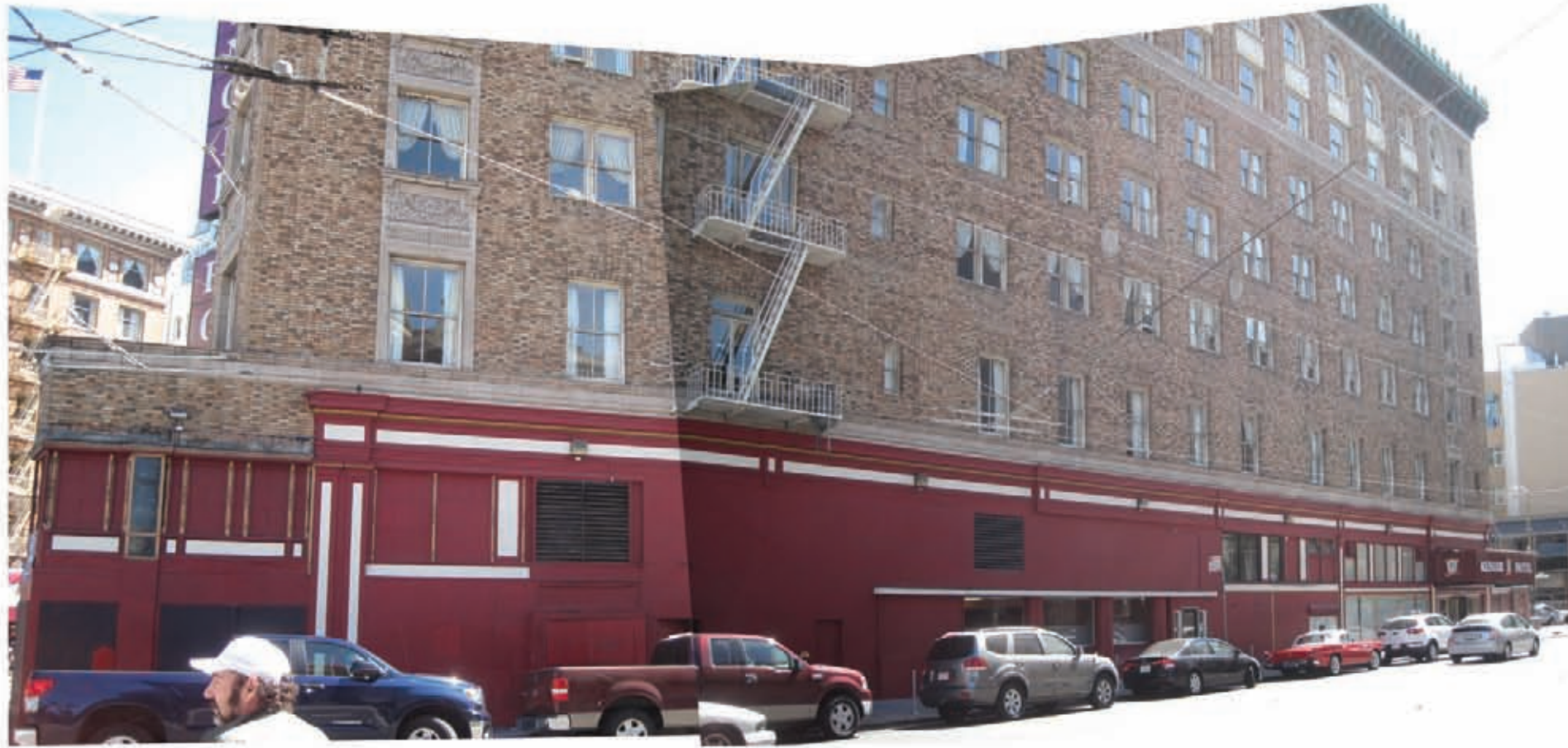
Existing McAllister Street Facade
