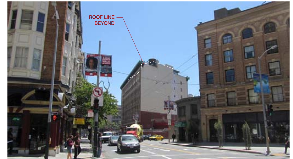
With New Roof Construction (Building Outline Beyond)
