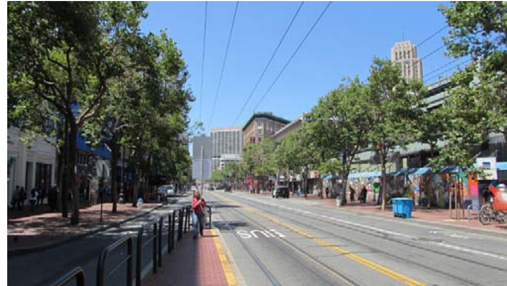
With New Roof Construction
