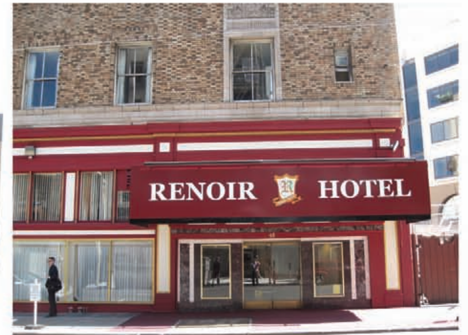
Existing McAllister Street Entrance
