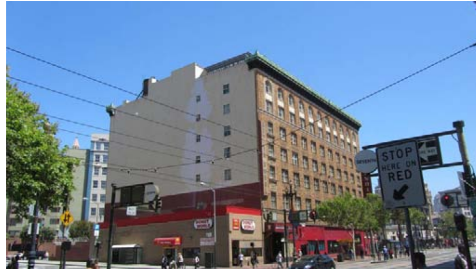
With New Roof Construction
