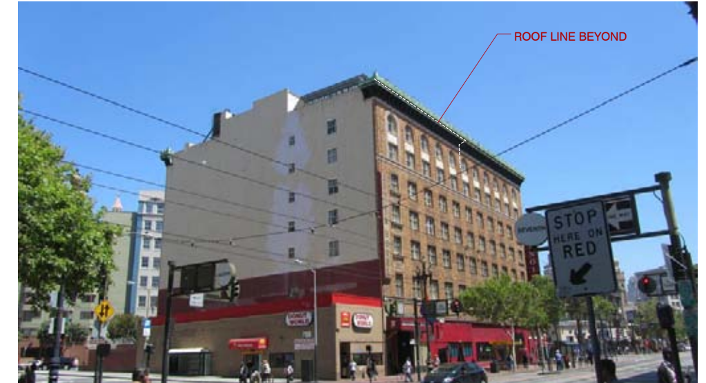
With New Roof Construction (Building Outline Beyond)
