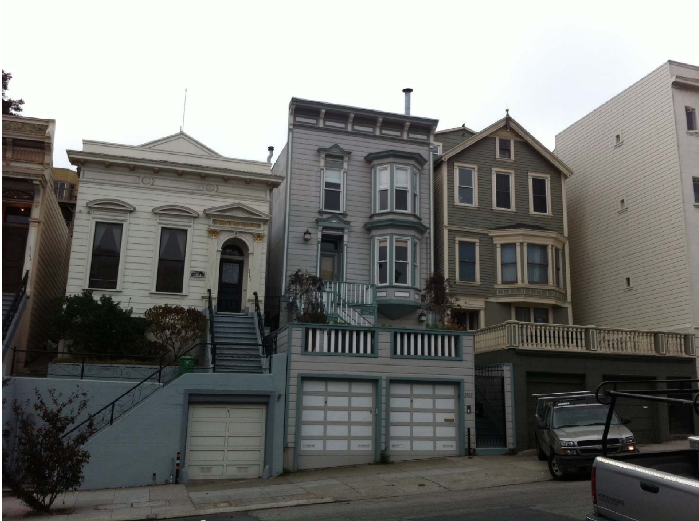
① VIEW FROM STREET
