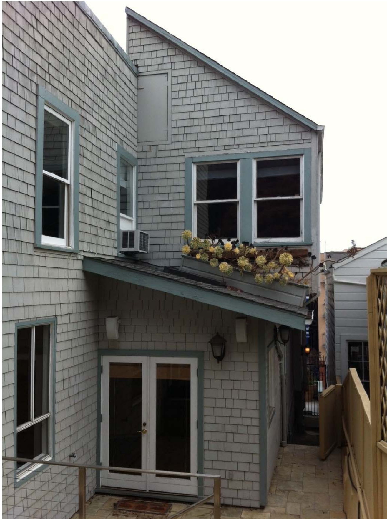
② VIEW OF REAR FACADE
