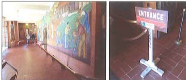
Existing mural barrier system
