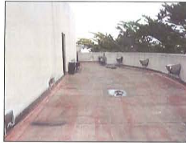
Second floor roof membrane
