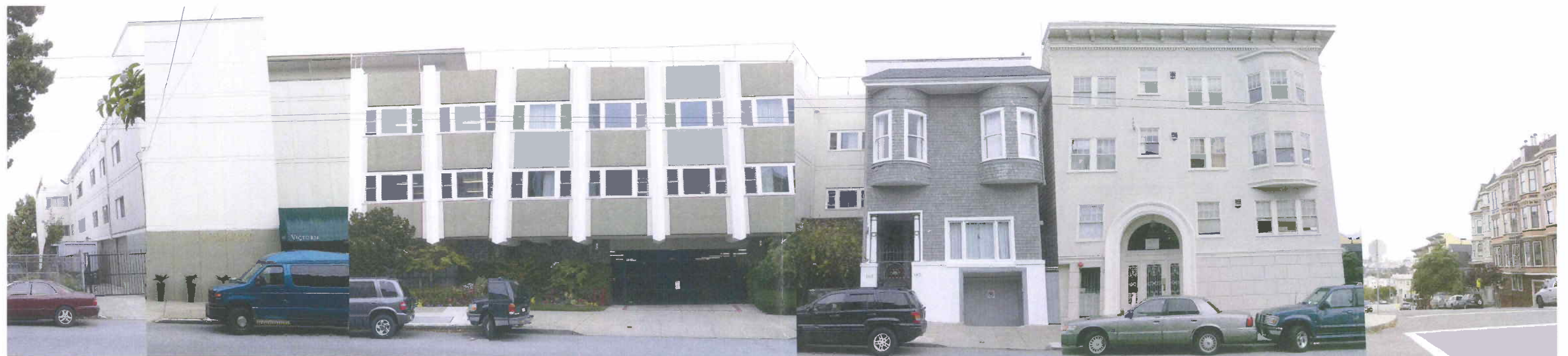
McALLISTER STREETScape SEGMENT #2
