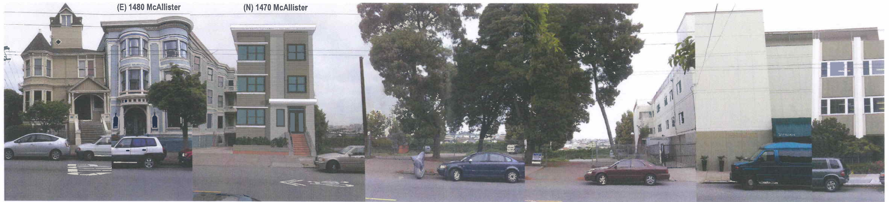
McALLISTER STREETScape SEGMENT #1
