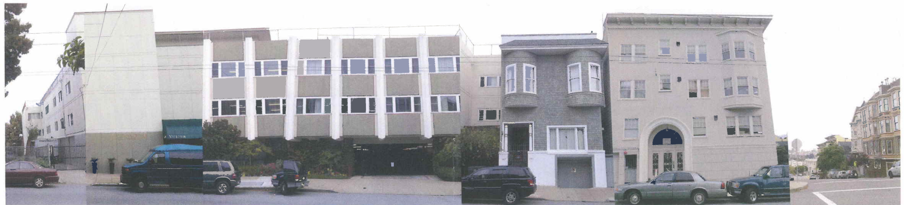
McALLISTER STREETScape SEGMENT #2
