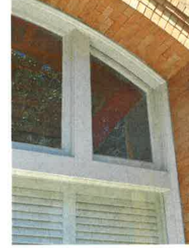
11 VIEW TO INTERIOR BRACE FRAME SCALE: NONE
