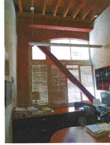
6 INTERIOR VIEW OF (E) BRACE FRAME SCALE: NONE
