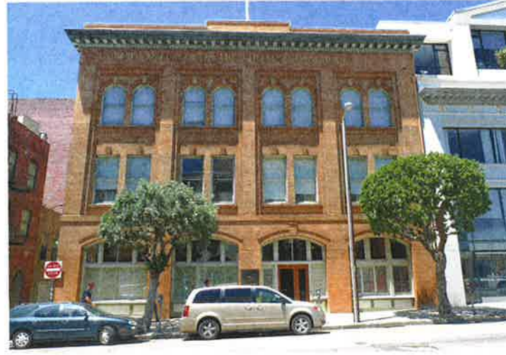
3 EXISTING EAST (SANSOME) FACADE SCALE: NONE
