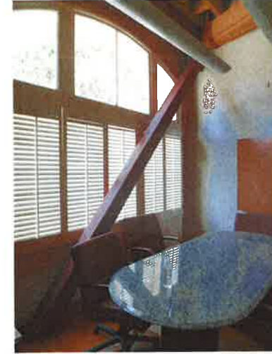
13 INTERIOR VIEW OF (E) BRACE FRAME SCALE: NONE
