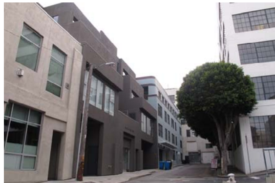
Figure 13. The east leg of Federal Street, looking southwest. The subject property is located behind the buildings on the left (41 and 51 Federal Street) (Source: Page & Turnbull, January 2013)
