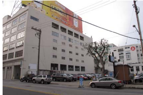
Figure 6. 274 Brannan Street to the west of the subject property, looking west. (Source: Page & Turnbull, January 2013)
