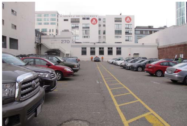
Figure 2. 270 Brannan Street, looking northwest. Source: Page & Turnbull, January 2013.
