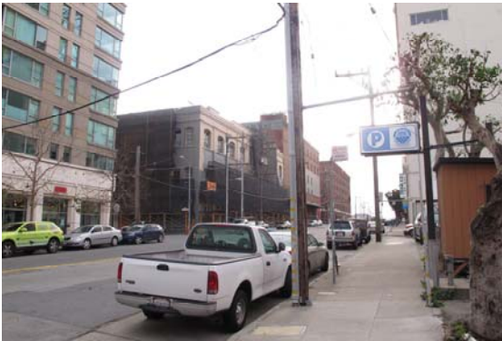
Figure 7. South side of Brannan Street, looking southwest from 270 Brannan. (Source: Page & Turnbull, January 2013)
