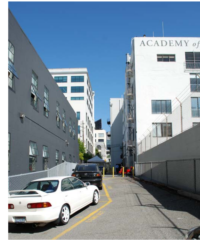
3 EASEMENT LOOKING NORTHWEST
