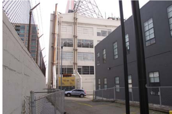
Figure 12. Unnamed alley between De Boom Street and Federal Street, with the wall of 270 Brannan abutting the street on the left, looking southeast. The back of 274 Brannan visible at the end of the street. (Source: Page & Turnbull, January 2013)
