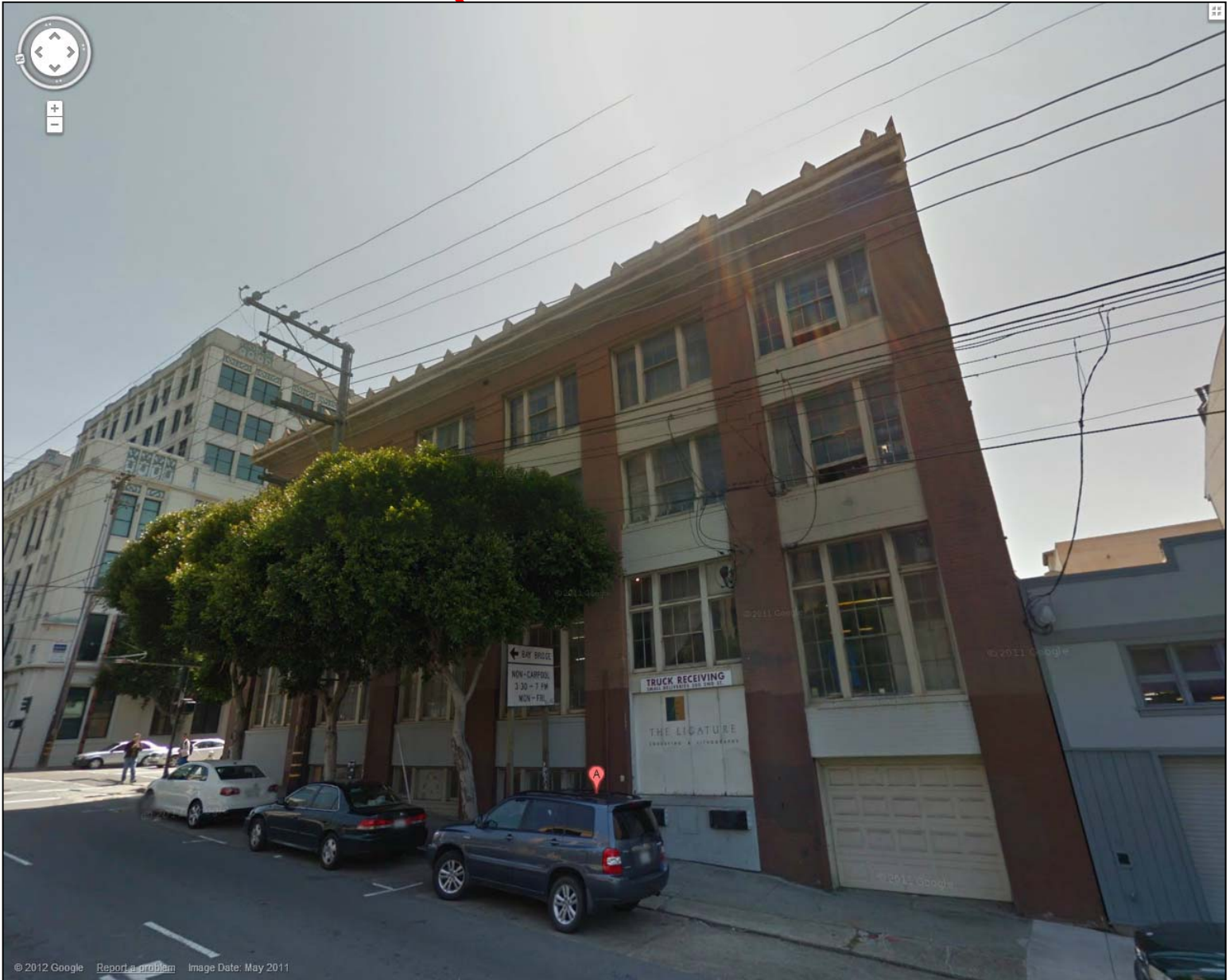
500 2 nd Street, View along Bryant Street (Source: Google Maps, Image Date April 2011; Accessed September 11, 2012)
