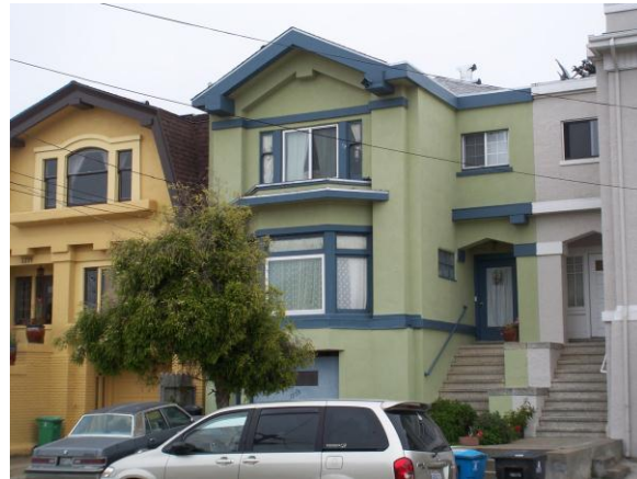
Figure 3. 1238 43 rd Avenue Source: KVP Consulting
