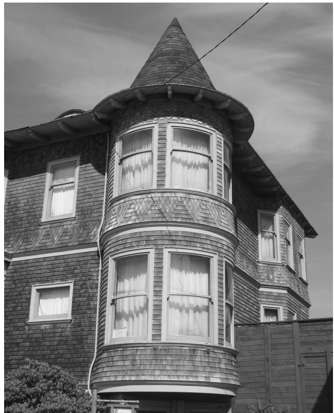
Example of the Shingle Style: Detail of Theodore Henn house, 1468 47th Avenue
