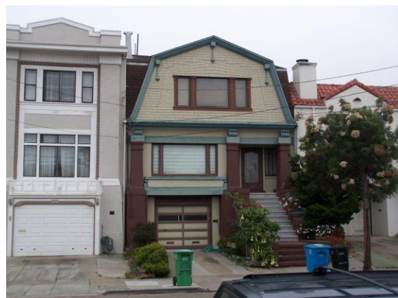
Figure 5. 1246 43 rd Avenue Source: KVP Consulting
