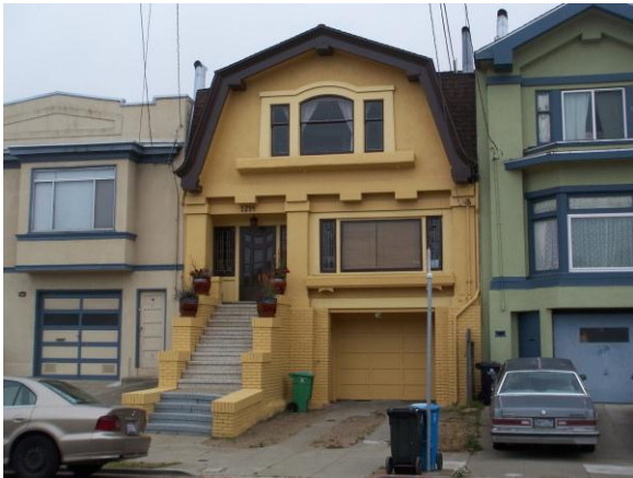
Figure 2. 1234 43 rd Avenue Source: KVP Consulting
