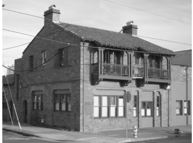
Commercial architecture in the Oceanside: 3655 Vicente Street.
