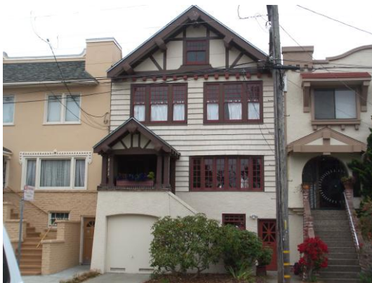
Figure 4. Typical Period Revival-style rowhouse at 1255 37 th Avenue Source: KVP Consulting
