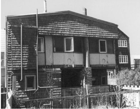
Rear facade of 1632 Great Highway Source: Woody LaBounty
