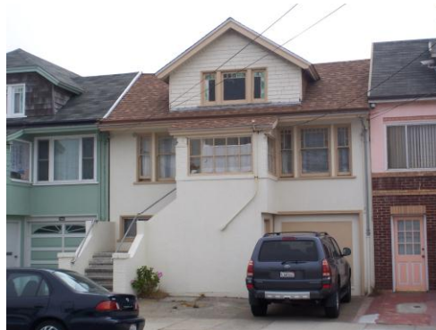
Figure 3. 1566 46 th Avenue Source: KVP Consulting
