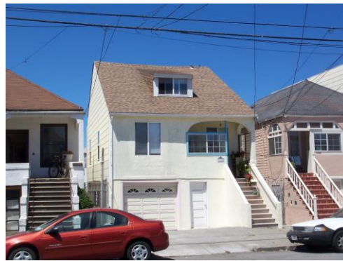
Figure 3. 1347 48 th Avenue Source: KVP Consulting
