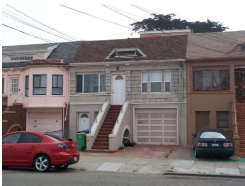
Figure 4. 1574 46 th Avenue Source: KVP Consulting
