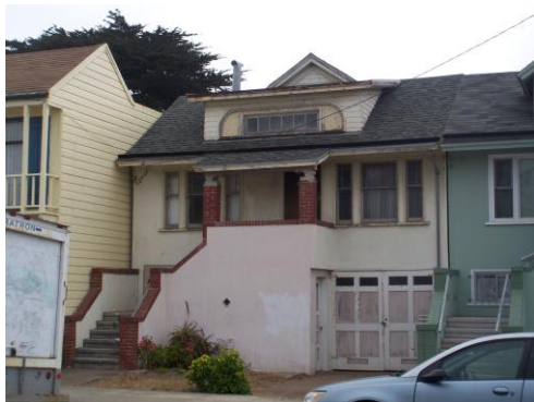
Figure 2. 1558 46 th Avenue Source: KVP Consulting
