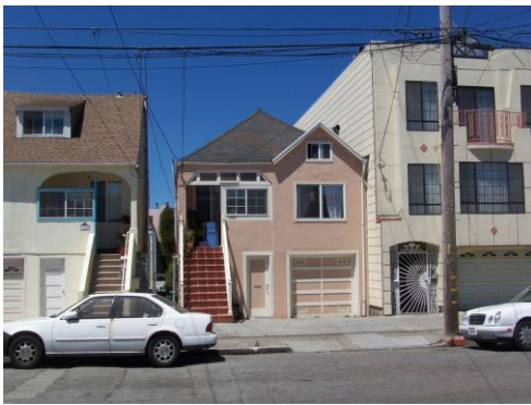
Figure 2. 1343 48 th Avenue Source: KVP Consulting
