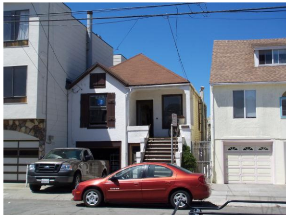
Figure 4. 1351 48 th Avenue Source: KVP Consulting
