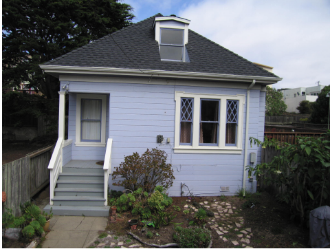
Cottage at rear of 1620 48th Avenue
