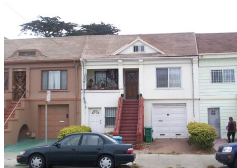
Figure 5. 1582 46 th Avenue Source: KVP Consulting
