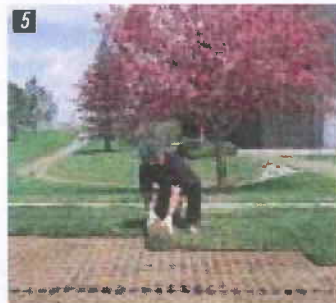
5 Hydroseed or lay sod.
