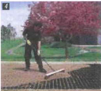
4 Fill rings with clean sharp concrete sand.
