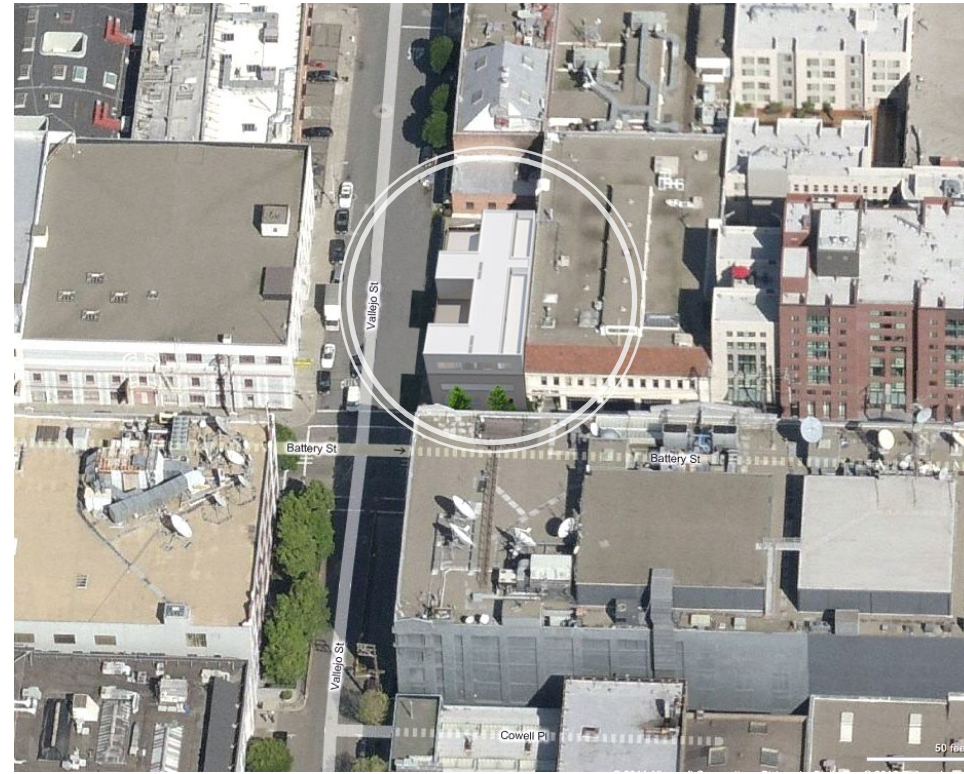
Aerial View Looking East
