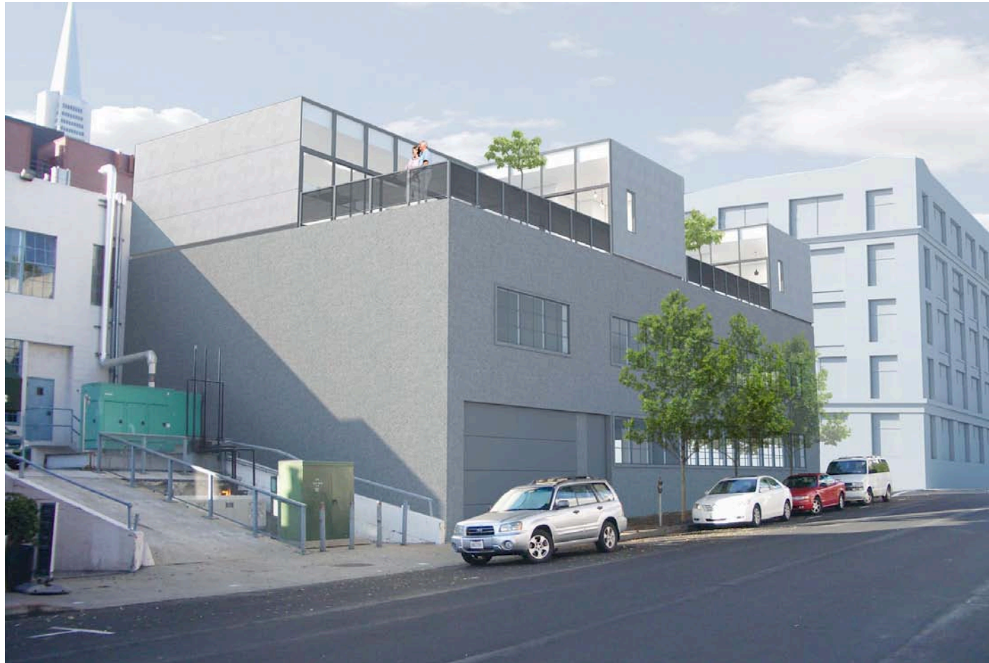
Vallejo Street View - Looking West
