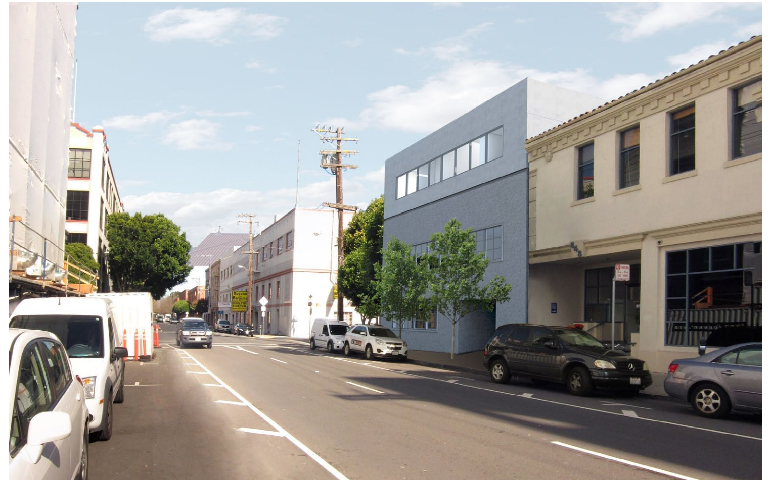
Battery Street View (Primary Façade) - Looking North
