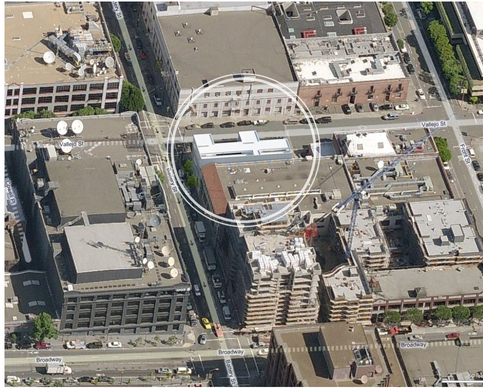
Aerial View Looking North
