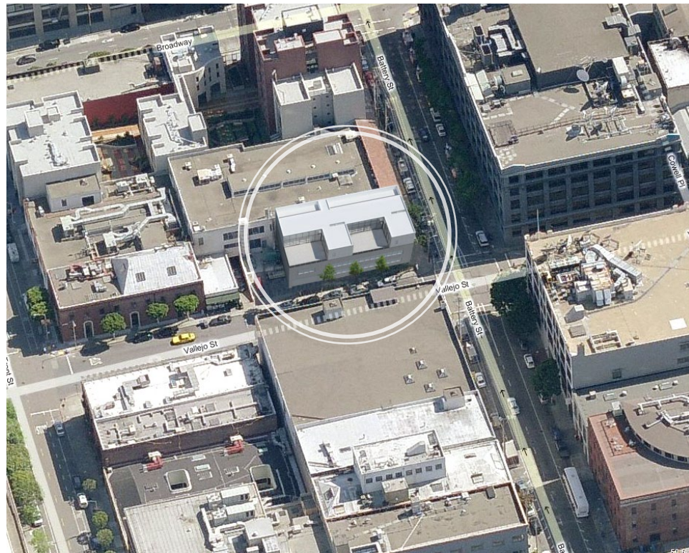
Aerial View Looking South
