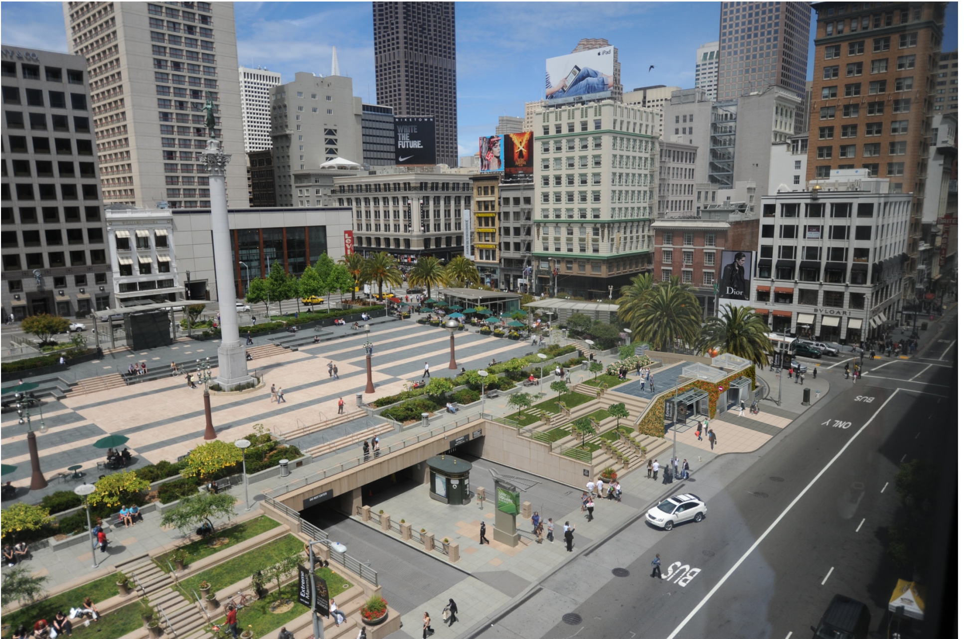
Aerial View of Station Entrance Looking toward Stockton and Geary Streets
