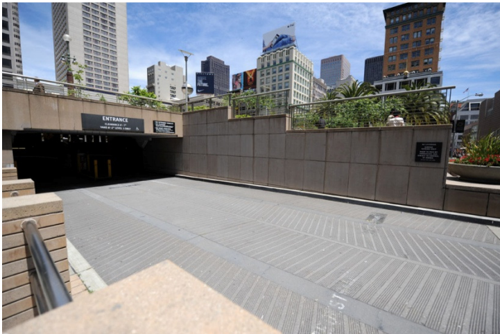
Existing garage entrance with stepped wall at Union Square
