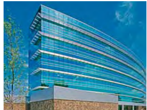
1600 Wall System®2 with 1600 SunShade®, Alcoa – Reynobond® and Reynolux® Panels Arkansas Department of Environmental Quality, Little Rock, Arkansas LEED® Gold certified Architects: Taggart Foster Currence Gray Architects, Inc., North Little Rock, Arkansas, and Williams & Dean Associated Architects, Little Rock, Arkansas Glazing Contractor: ACE Glass Co., Inc., Little Rock, Arkansas
