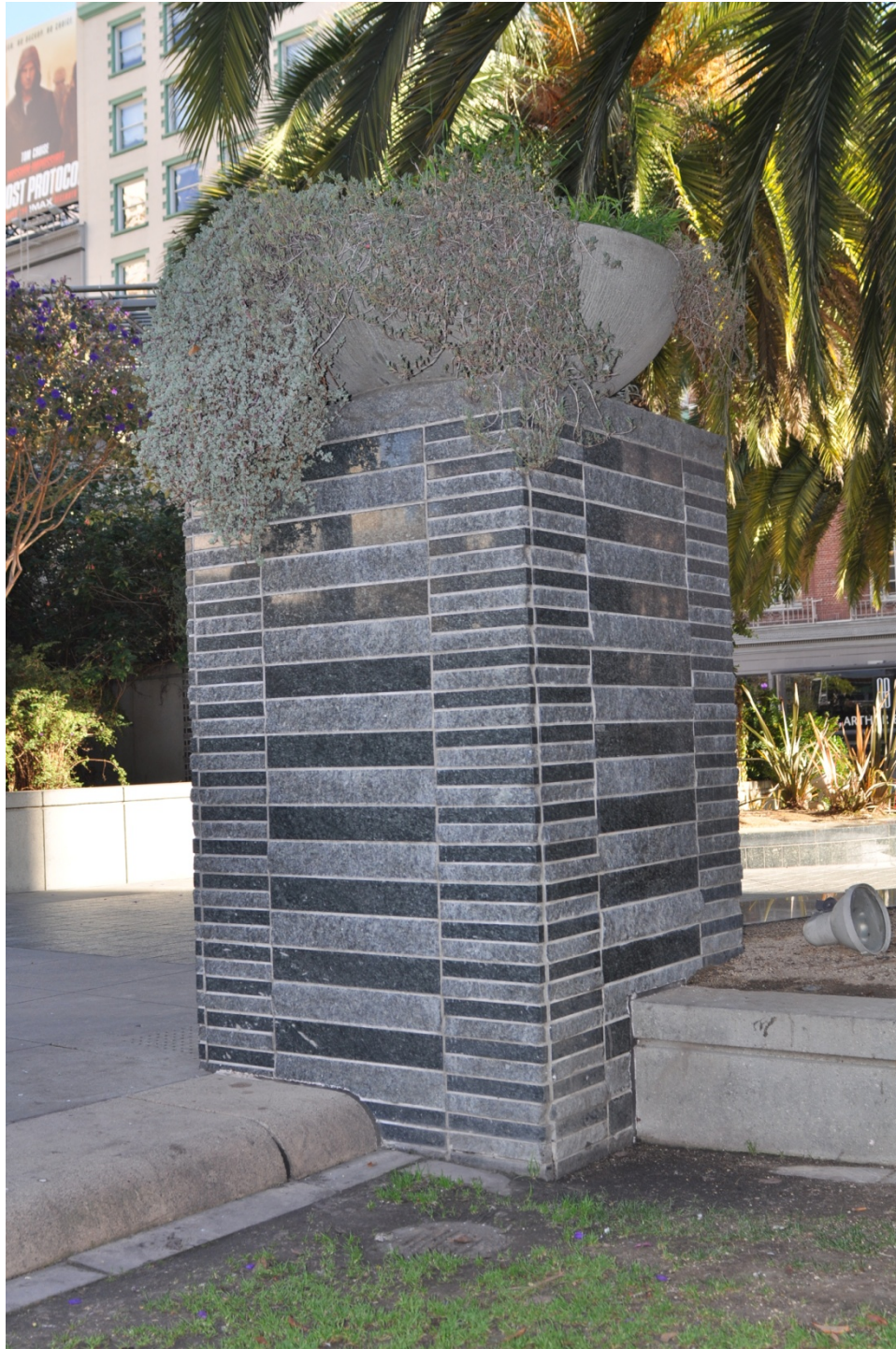
Existing Stone Pilaster at Intermediate Plaza Level (to remain)
