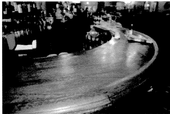
Figure 2. Curved bar was existing in 1954 when the space was remodeled to include restrooms. An exact date for installation is unknown.
