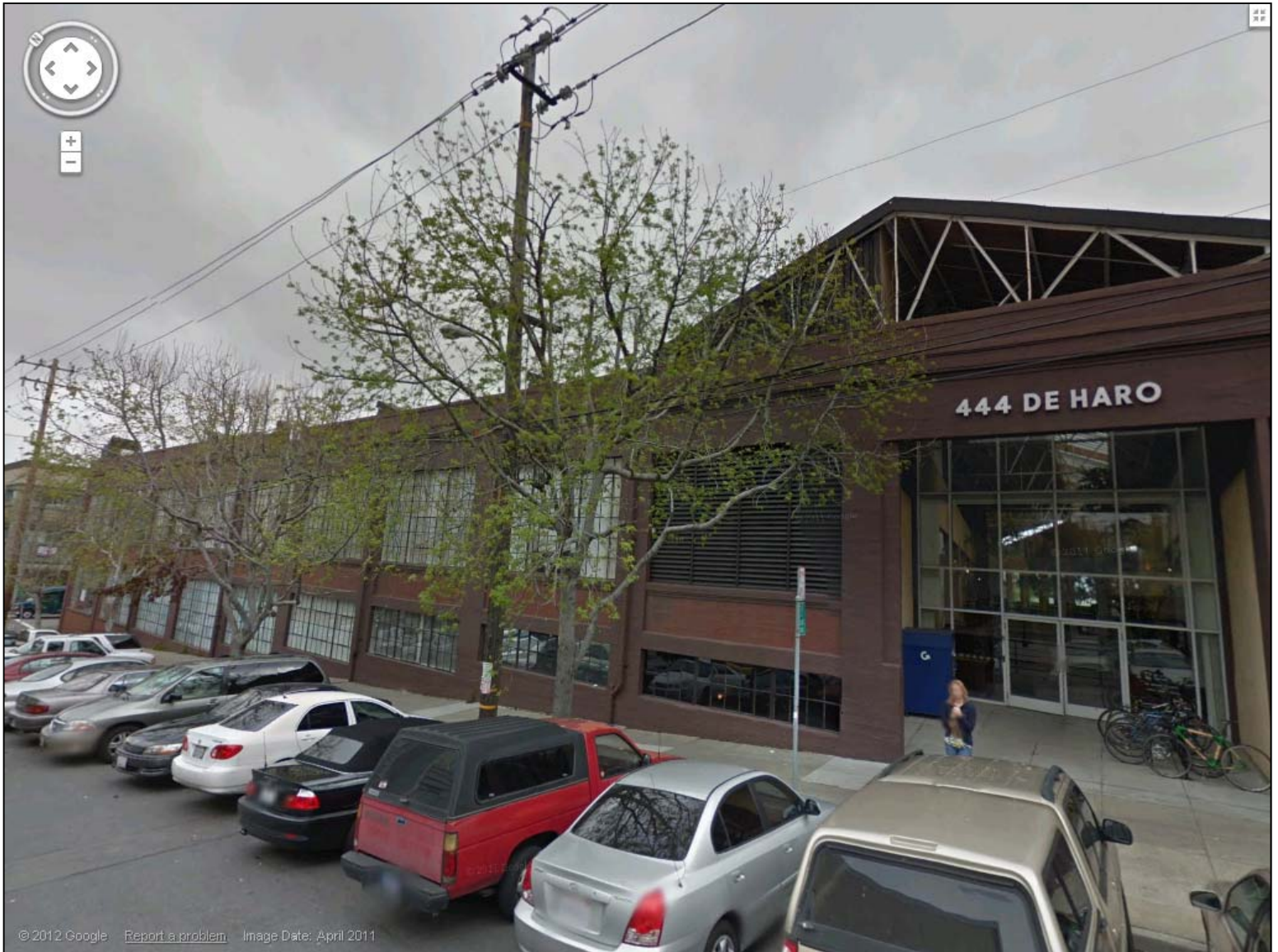
444 De Haro Street, View along Rhode Island Street
