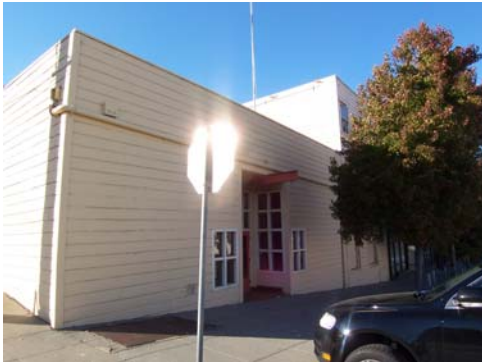
100_2146.JPG, 11/20/07, view to W, frame addition
