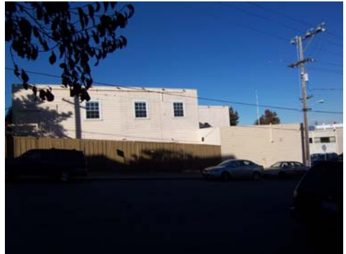
100_2148.JPG, 11/20/07, view to N, frame addition
