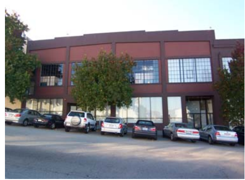
100_2145.JPG, 11/20/07, view to W, concrete addition
