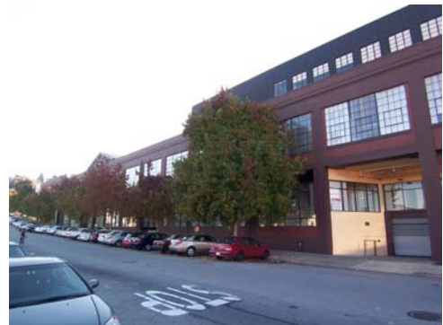
100_2142.JPG, 11/20/07, south elevation
