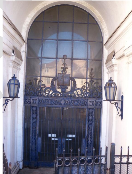
Figure 17. Main entrance to Woods Hall, 2012 Source: Christopher VerPlanck
