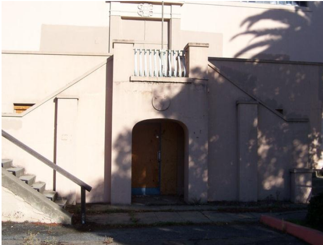
Figure 12. Historic stair and entrance to Middle Hall, 2012
