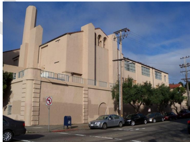
Figure 7. East façade of Richardson Hall, 2012 Source: Chris VerPlanck
