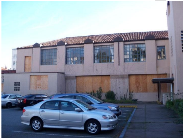
Figure 9. West façade of Richardson Hall, 2012 Source: Christopher VerPlanck
