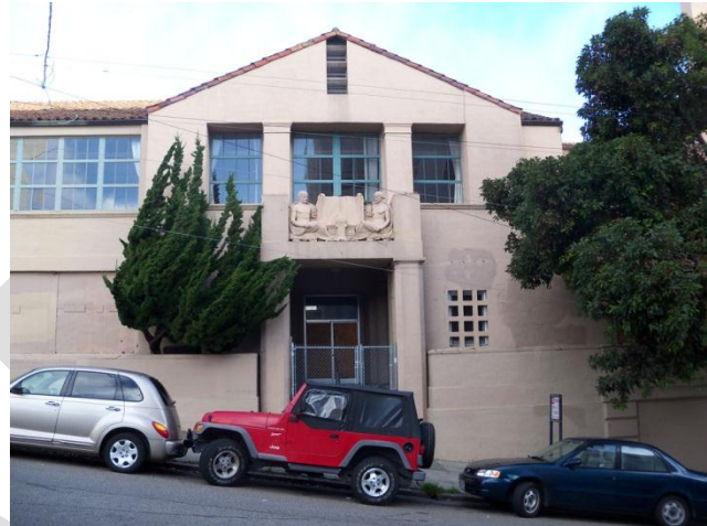
Figure 6. Primary entrance to Richardson Hall, 2012 Source: Christopher VerPlanck
