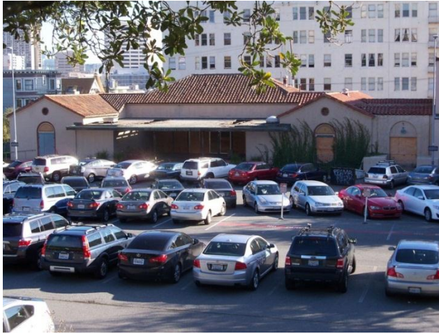
Figure 11. West façade of Richardson Hall Annex, 2012
