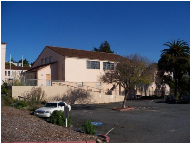
Figure 13. Oblique view of Middle Hall from southwest
