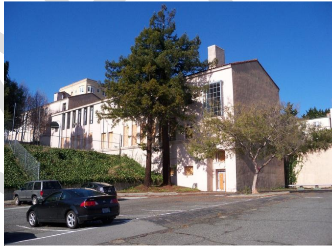
Figure 23. South and east façades of Woods Hall Annex, 2012 Source: Christopher VerPlanck
