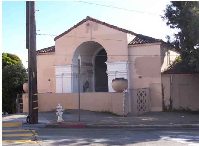
Figure 16. Entry pavilion of Woods Hall, 2012 Source: Christopher VerPlanck
