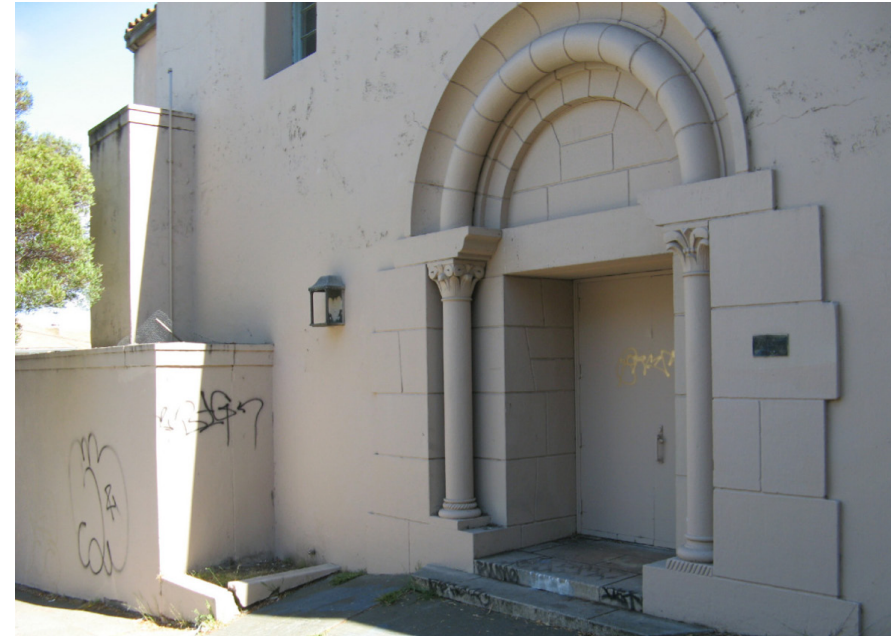
Main entrance along Buchanan Street
