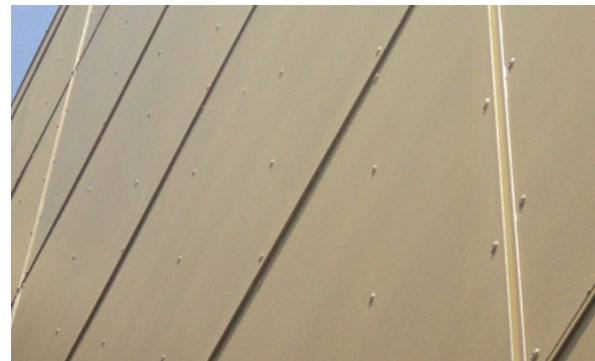
Coated fiber cement panels at bay window spandrel
