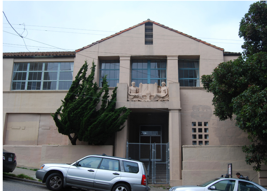
Main entrance at Hermann Street
