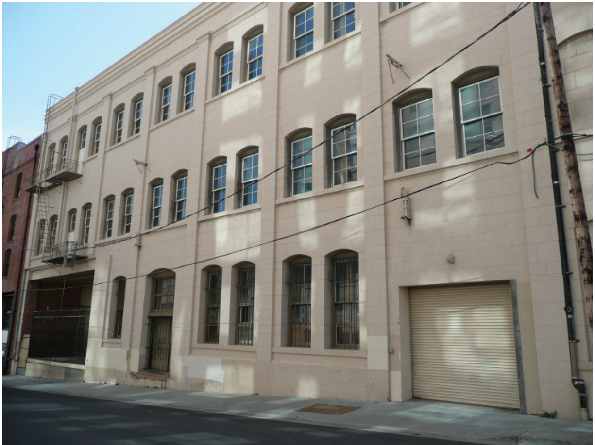
Figure A7. View of bays 3-9 on the Colin P. Kelly Street side (Architectural Resources Group, October 2011).
