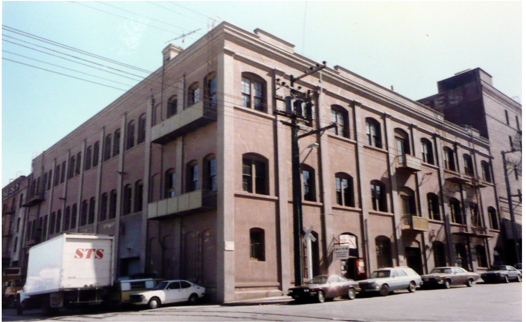
Figure B9. Mid-1980s photograph of 275 Brannan Street. Note the chimney above the filled-in column of window openings along Colin P. Kelly Street ("275 Brannan Street" file, San Francisco Planning Department).
