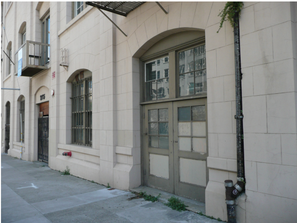
Figure A4. View of entry at seventh bay of main façade (Architectural Resources Group, October 2011).
