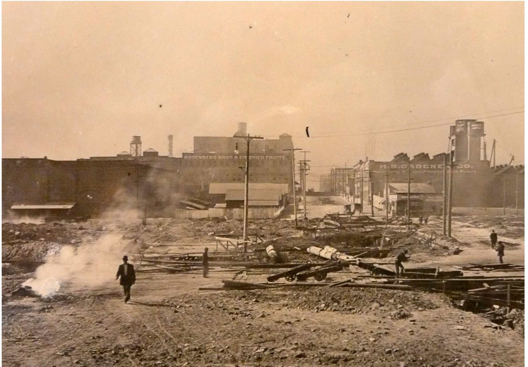
Figure B4. 1912 view looking west along Brannan Street. The Oriental Warehouse (now 650 Delancey Street) is in the left foreground, with the three-story Rosenberg Bros. warehouse behind (San Francisco History Center, San Francisco Public Library).
