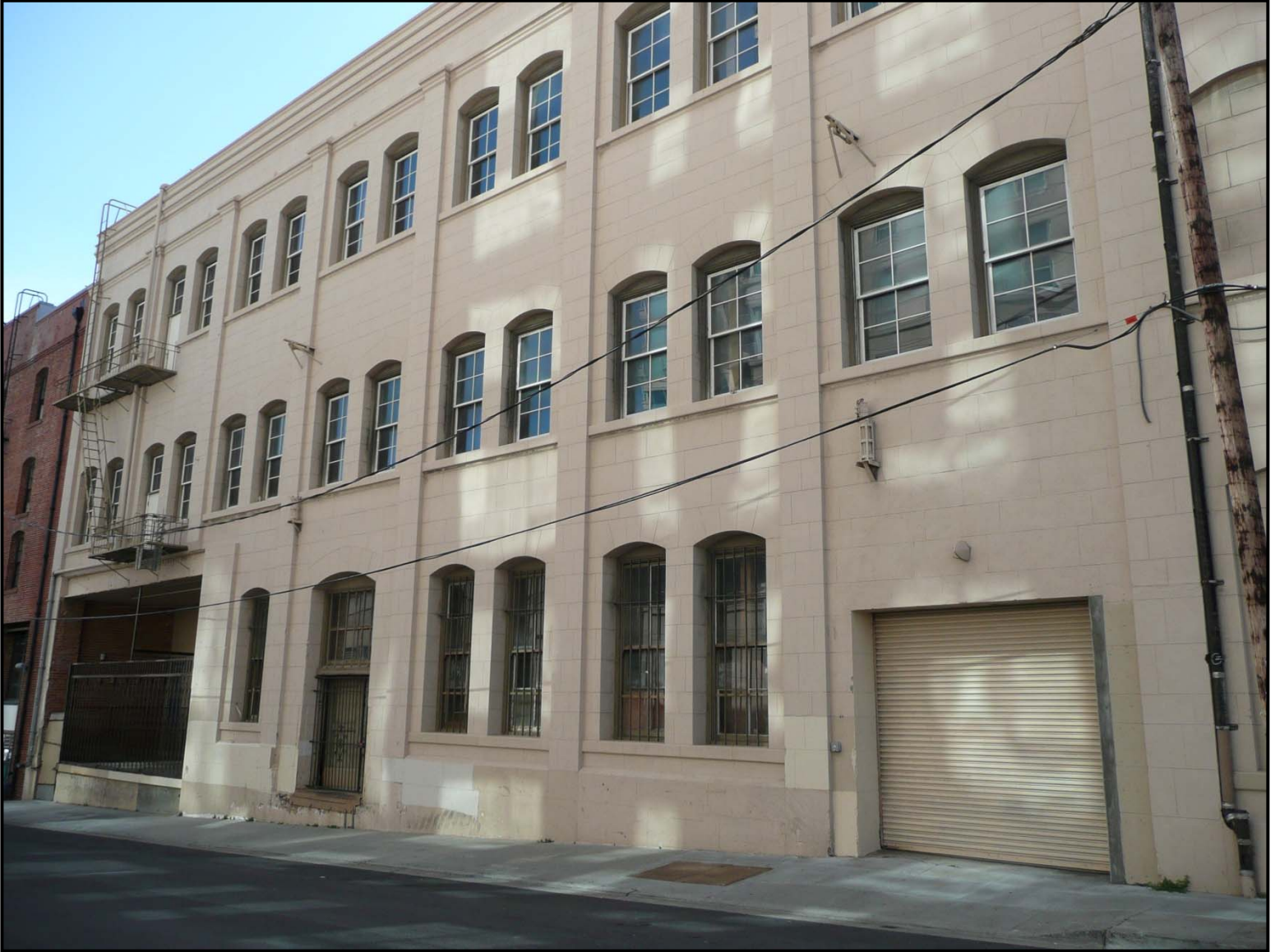
275 Brannan St, View of Colin P. Kelly Street Facade
