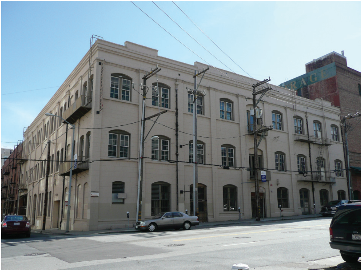
Figure A1. View of east and north elevations (Architectural Resources Group, October 2011).
