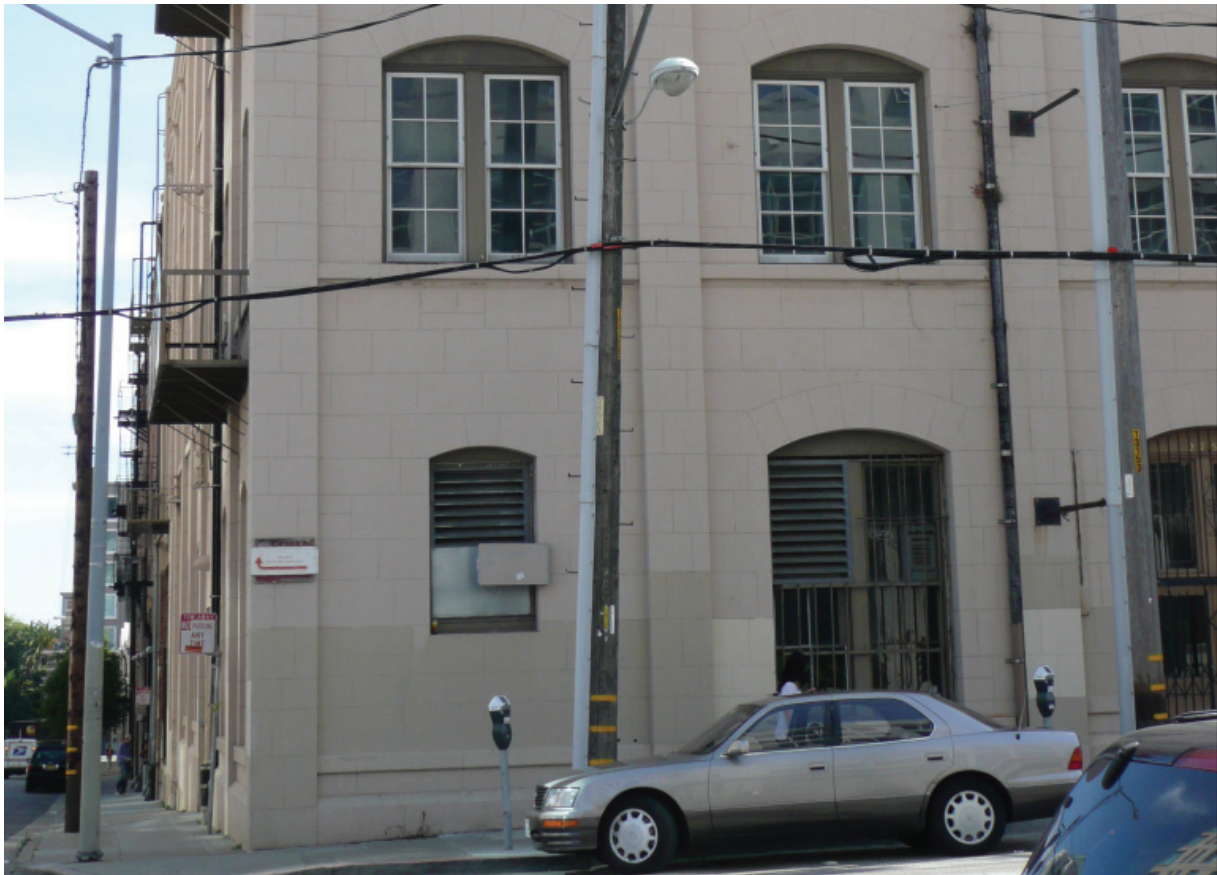
Figure A5. A smaller, single window opening marks the ground floor's first bay, corresponding to the original boiler room (Architectural Resources Group, October 2011).
