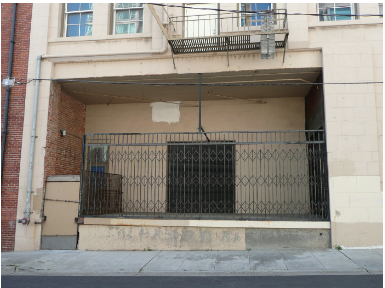
Figure A8. View of the loading dock, Colin P. Kelly Street side (Architectural Resources Group, October 2011).
