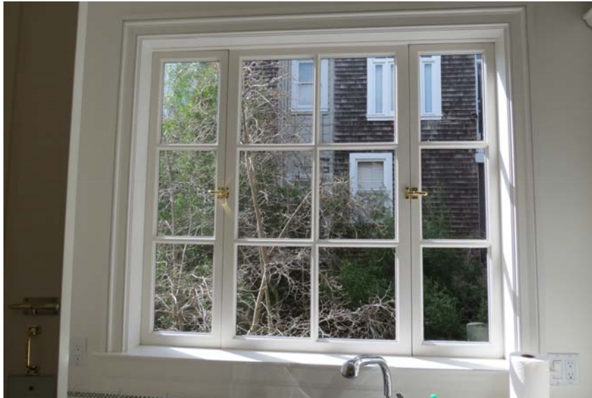
Figure 5. Window 211 – Multi-lite Fixed with Casement.
