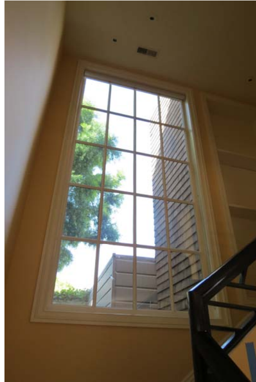
Figure 4. Window 306 – Multi-lite fixed.
