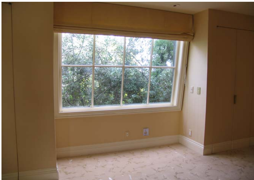
Figure 6. Window 306 – Multi-lite fixed installed at a slant.
