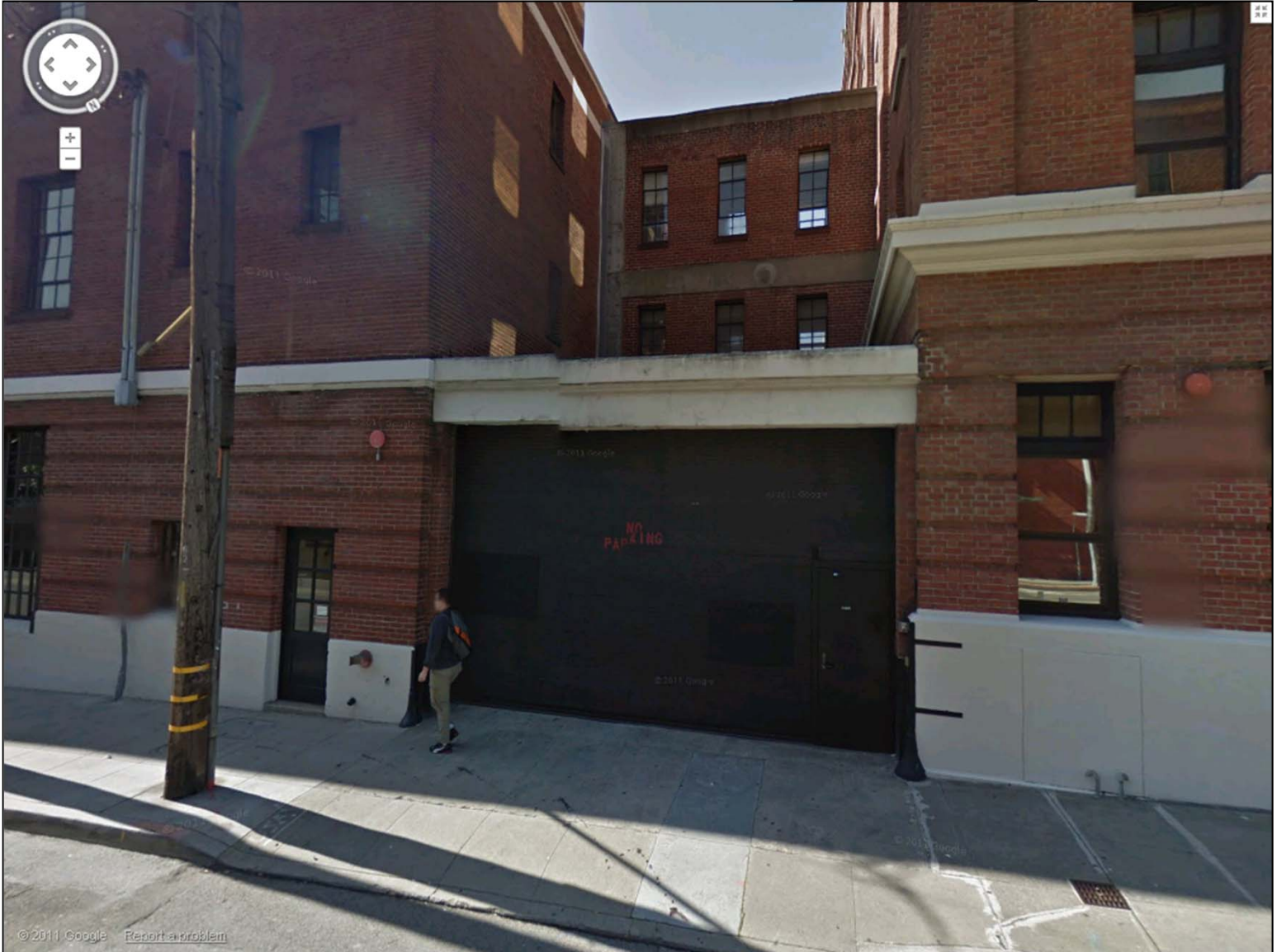
301 Brannan Street, View of private alley from 2 nd Street
