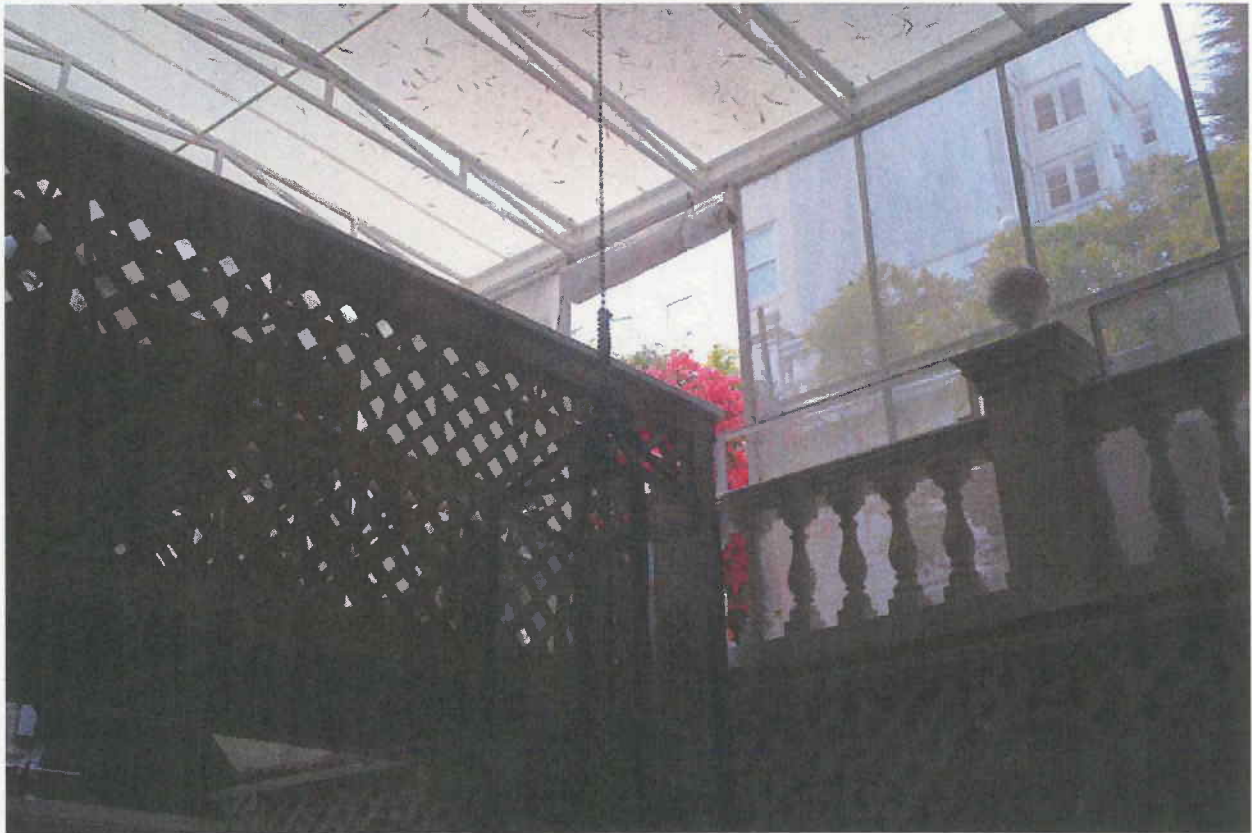
Existing Roof Enclosure - Facing North
