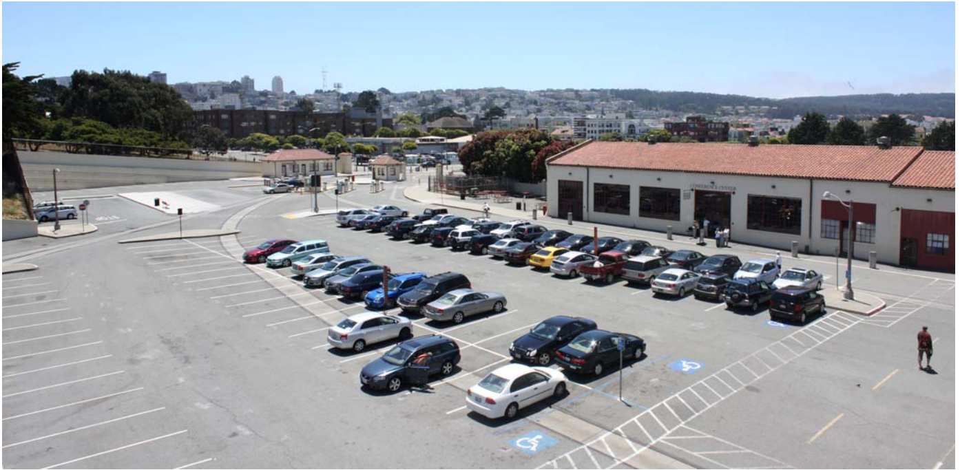
Existing view - Fort Mason Building C stairway looking south
