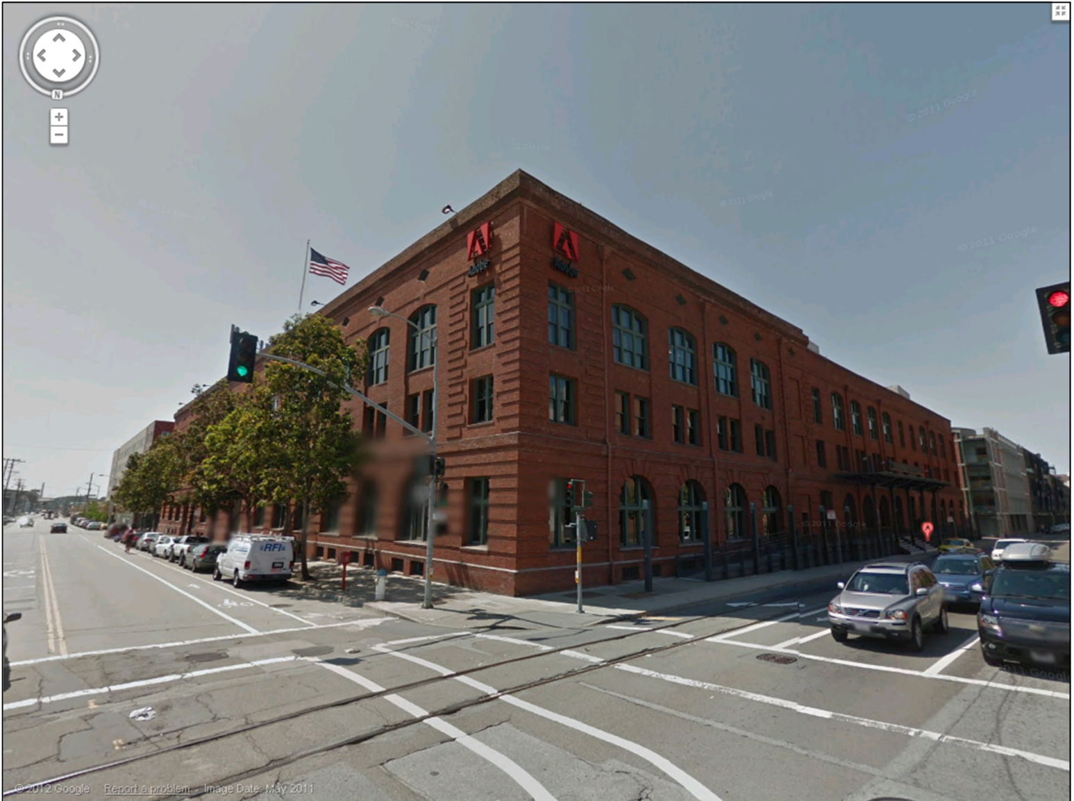
601 Townsend Street, View of Townsend and 7 th Streets
