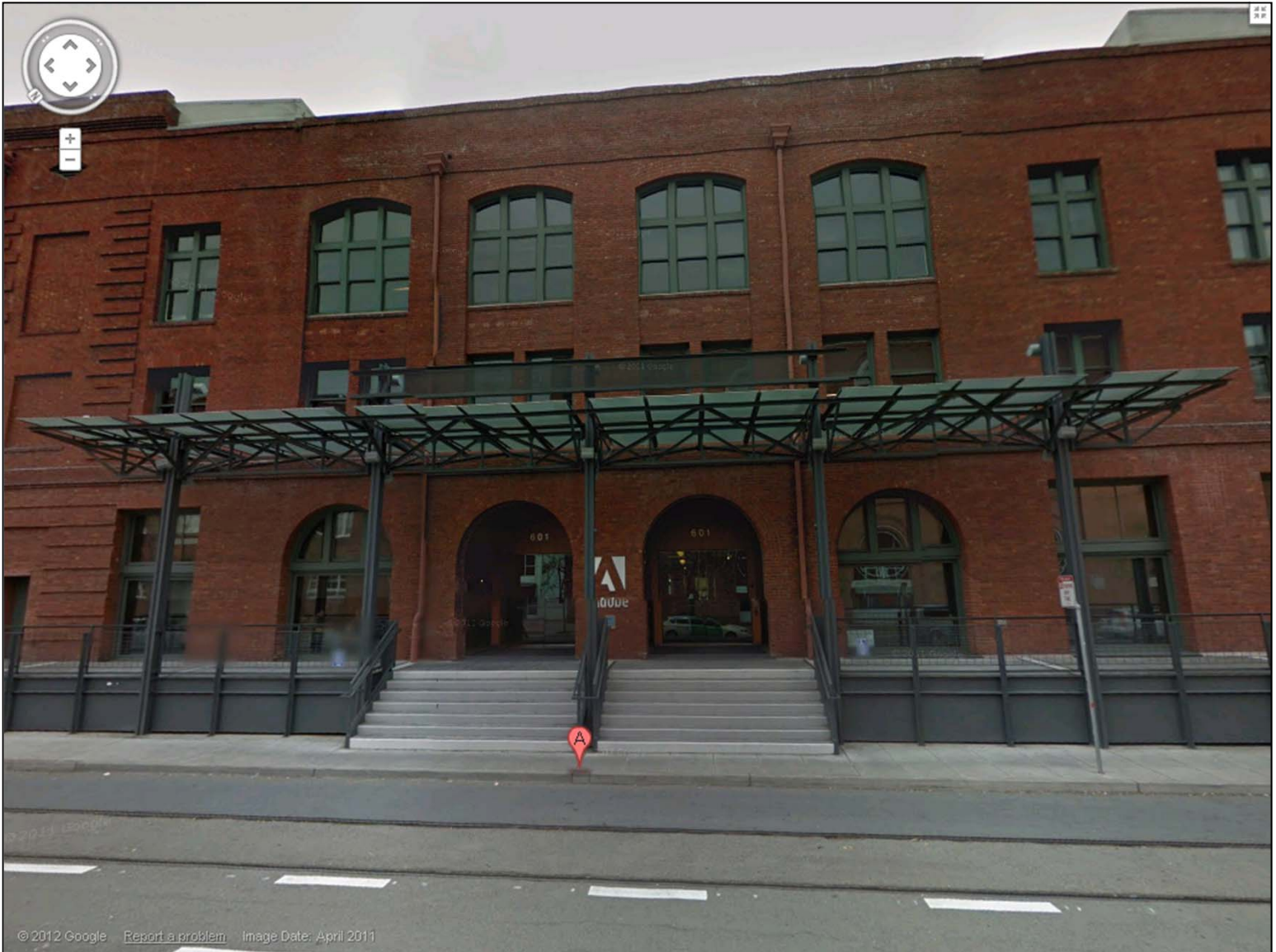
601 Townsend Street, Main Entrance along Townsend Street
