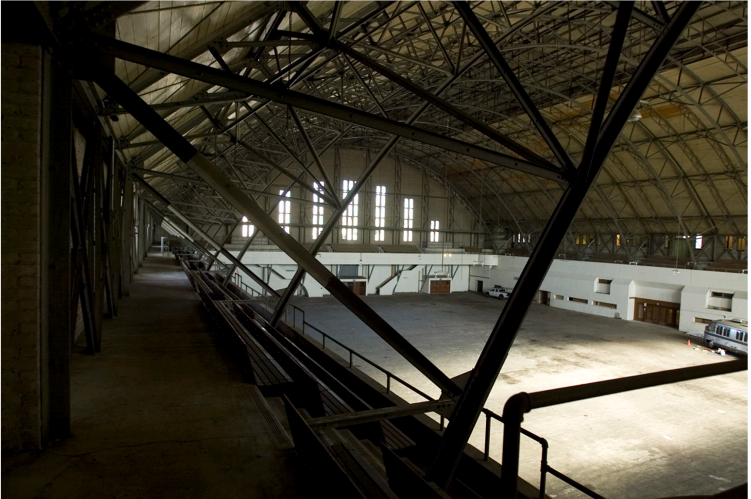
State Armory and Arsenal, Interior, Drill Court, View of Mezzanine Level
