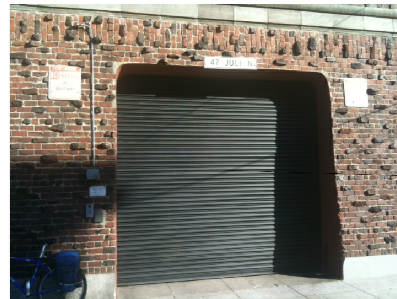
SOUTHWEST CORNER OF DRILLCOURT AT JULIAN AVENUE SERVICE DOOR
