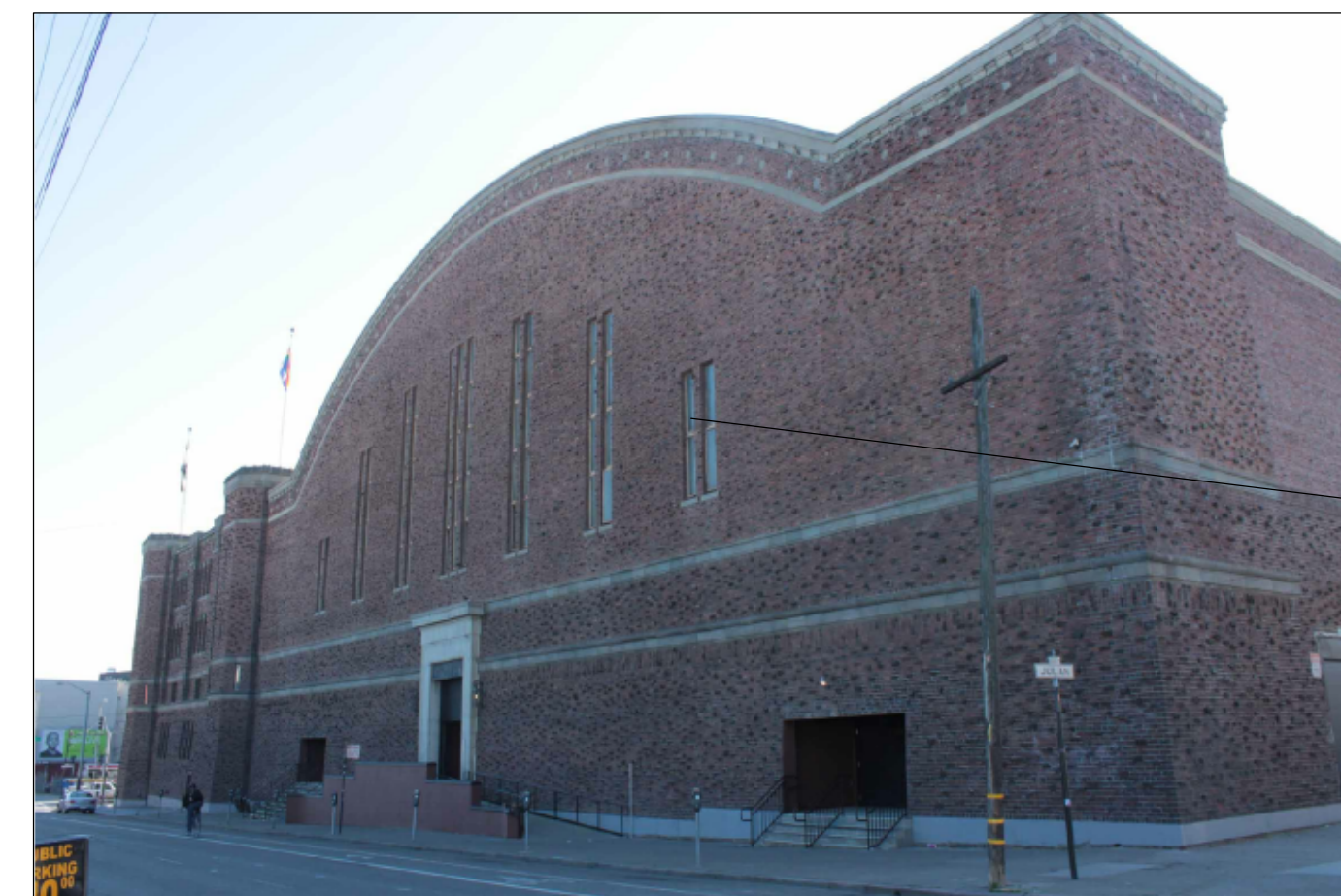
VIEW FROM NORTHWEST CORNER - ALL DRILL COURT WINDOWS TO BE WORKED UPON: NORTH, WEST AND SOUTH ELEVATIONS
