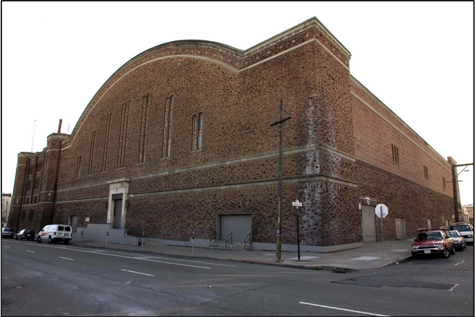
State Armory and Arsenal, View along 14 th Street
