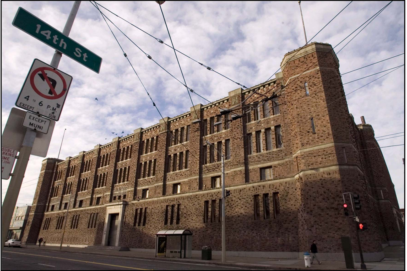
State Armory and Arsenal, View along Mission Street
