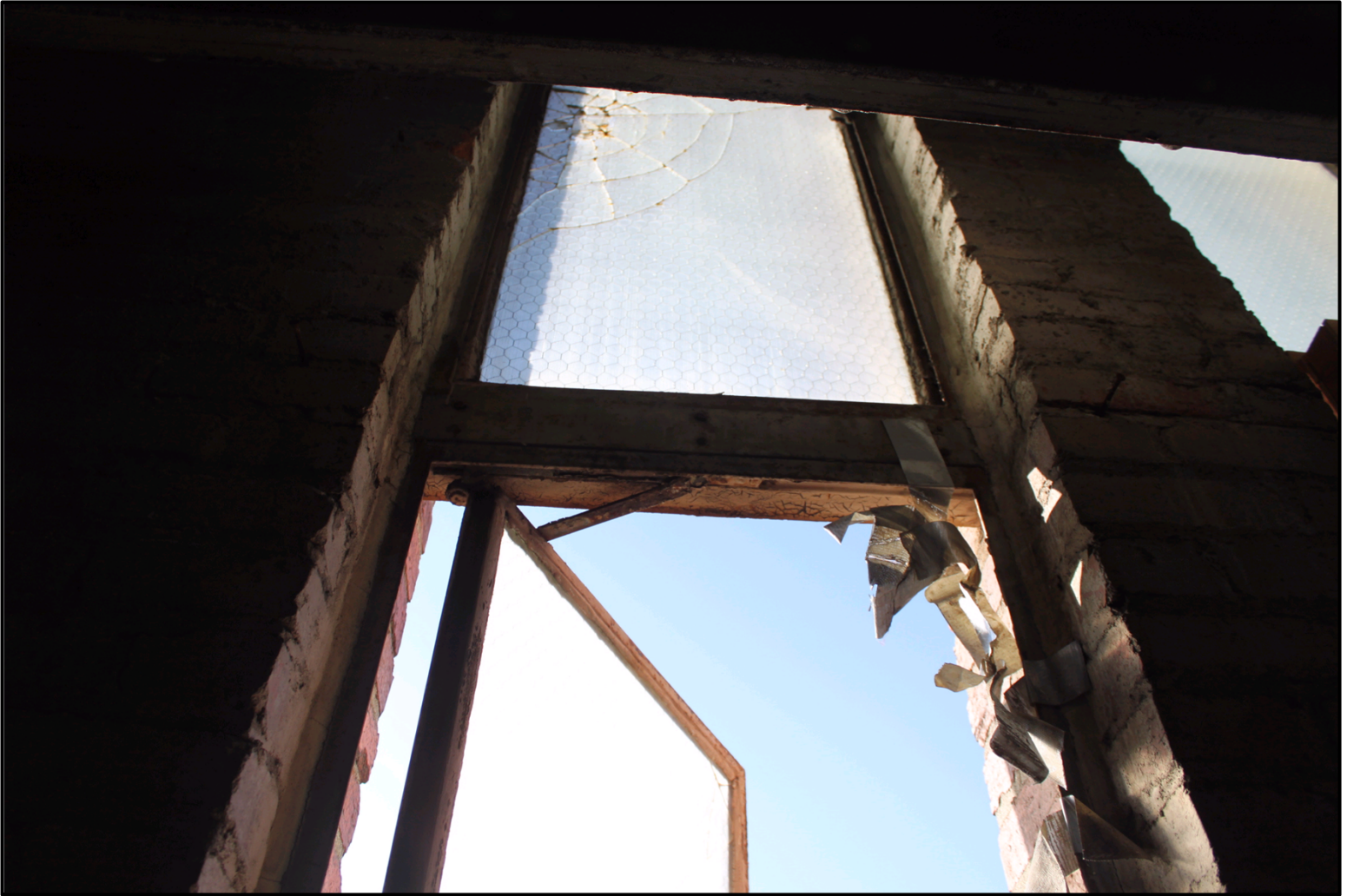
State Armory and Arsenal, Interior, Drill Court, View of Windows
