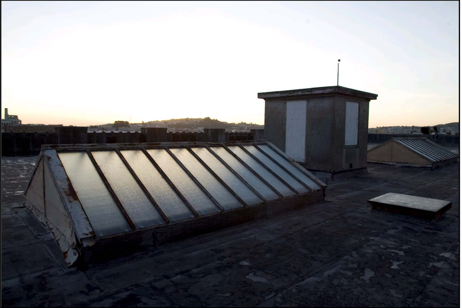
State Armory and Arsenal, View of Administration Building Roof
