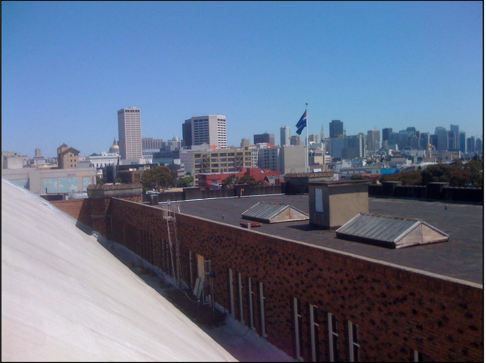
State Armory and Arsenal, View of Roof
