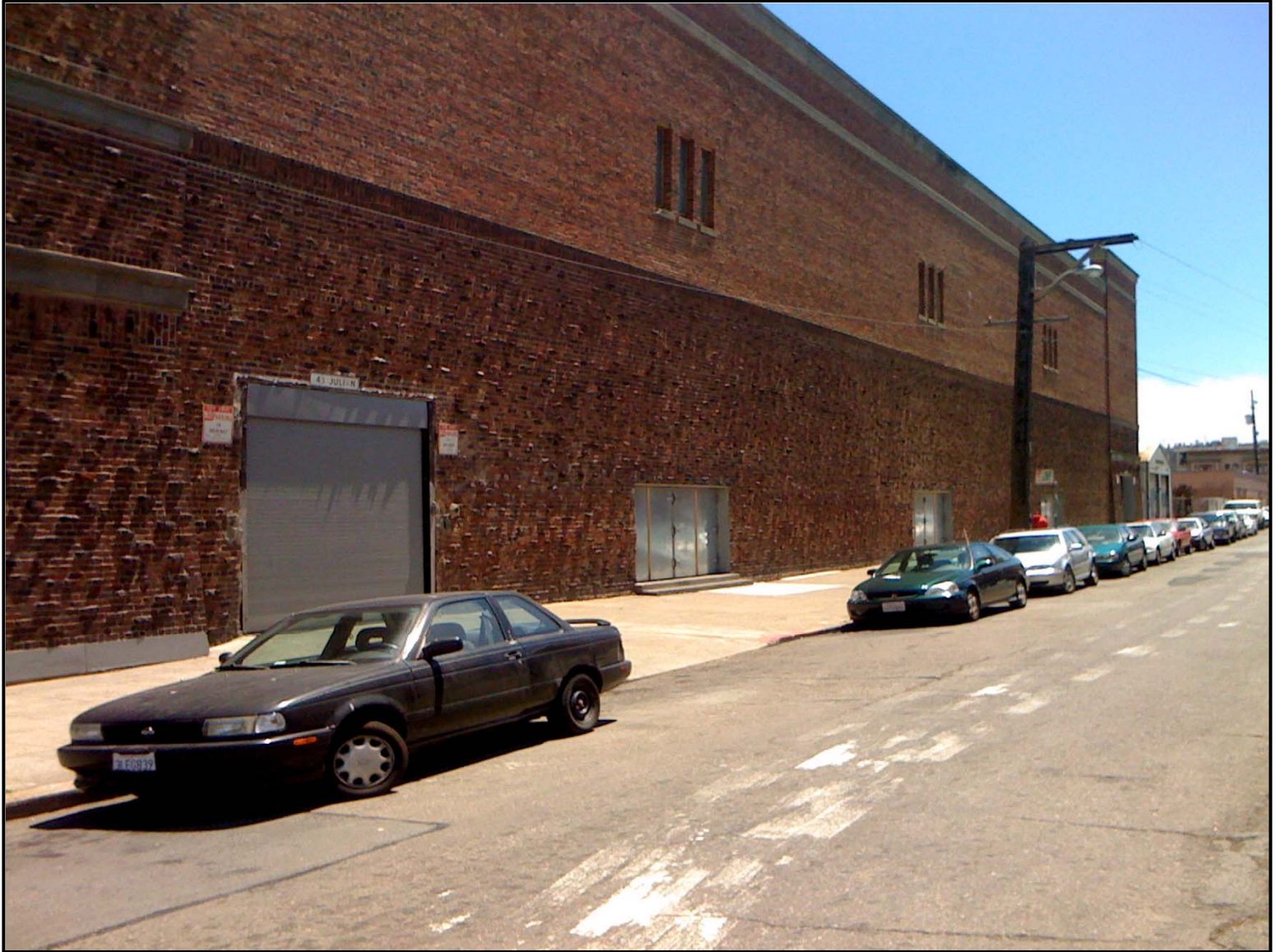
State Armory and Arsenal, View along Julian Avenue
