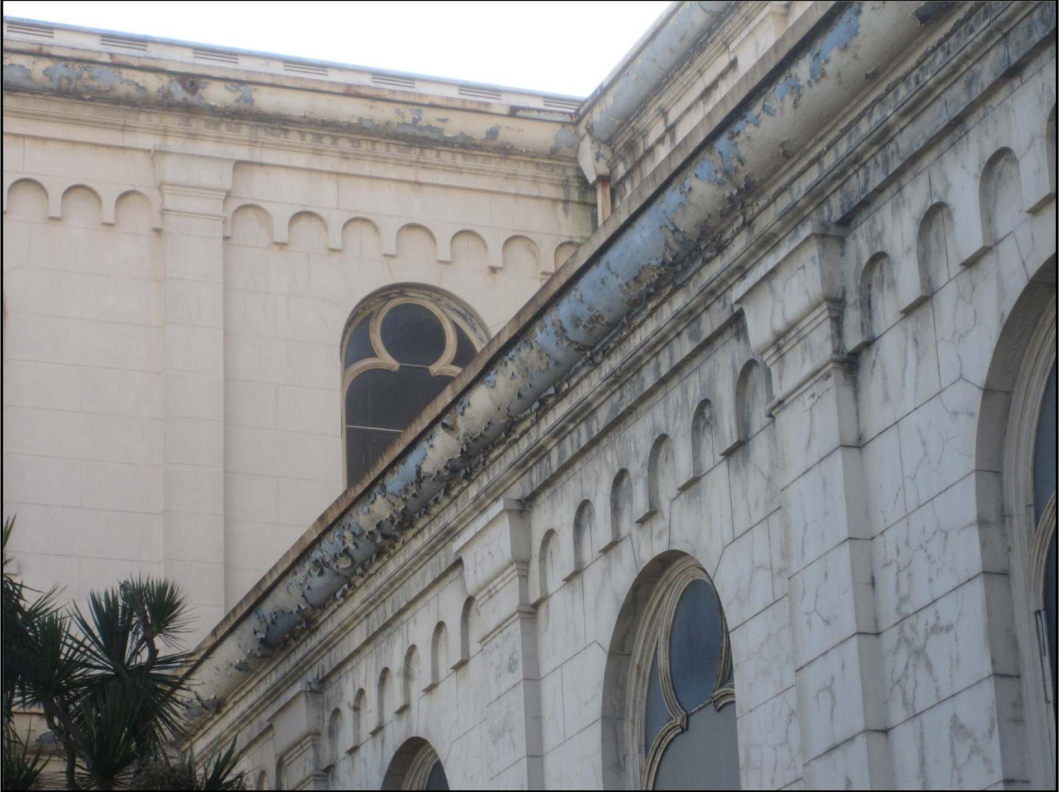
1401 Howard Street, Detail View of Sheet Metal Cornice along East Facade
