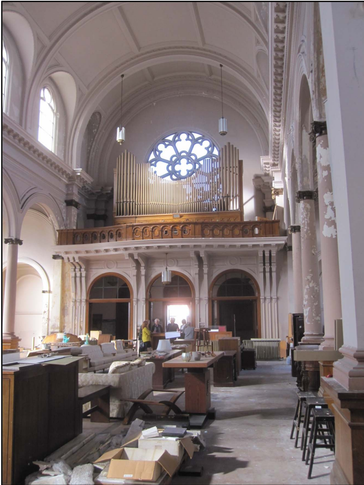
1401 Howard Street, View of Nave and Organ Loft
