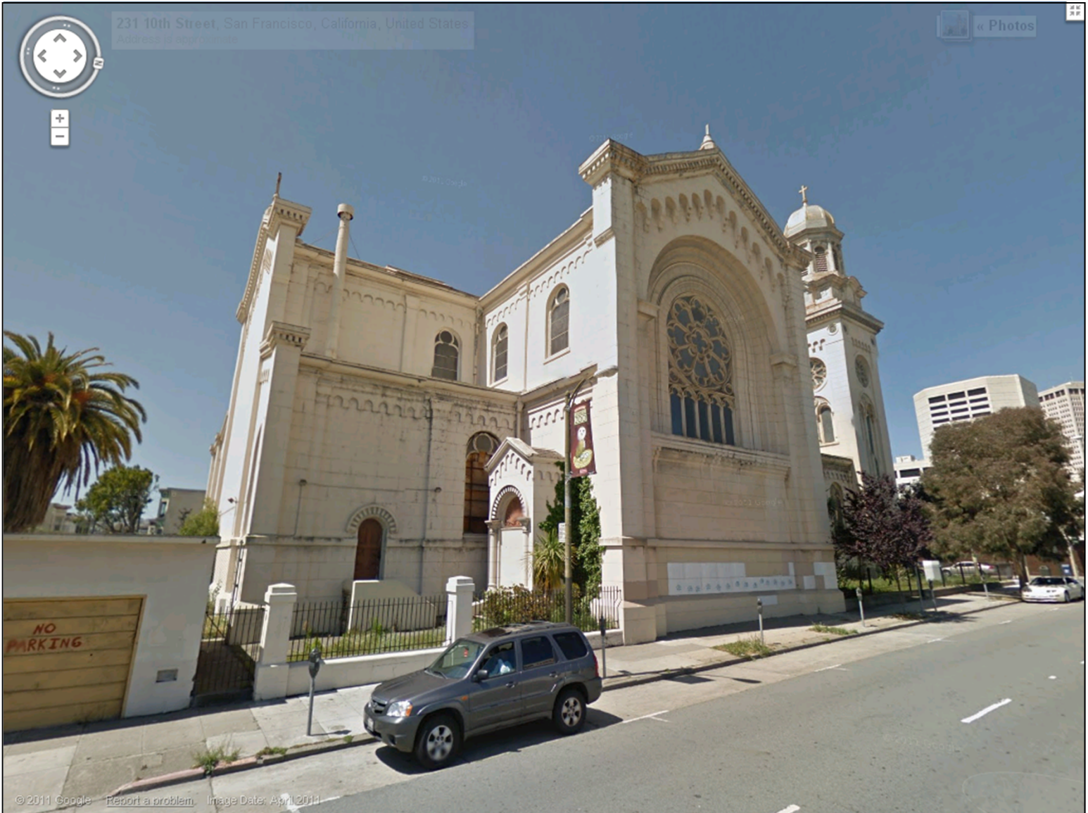
1401 Howard Street, View along 10 th Street looking north
