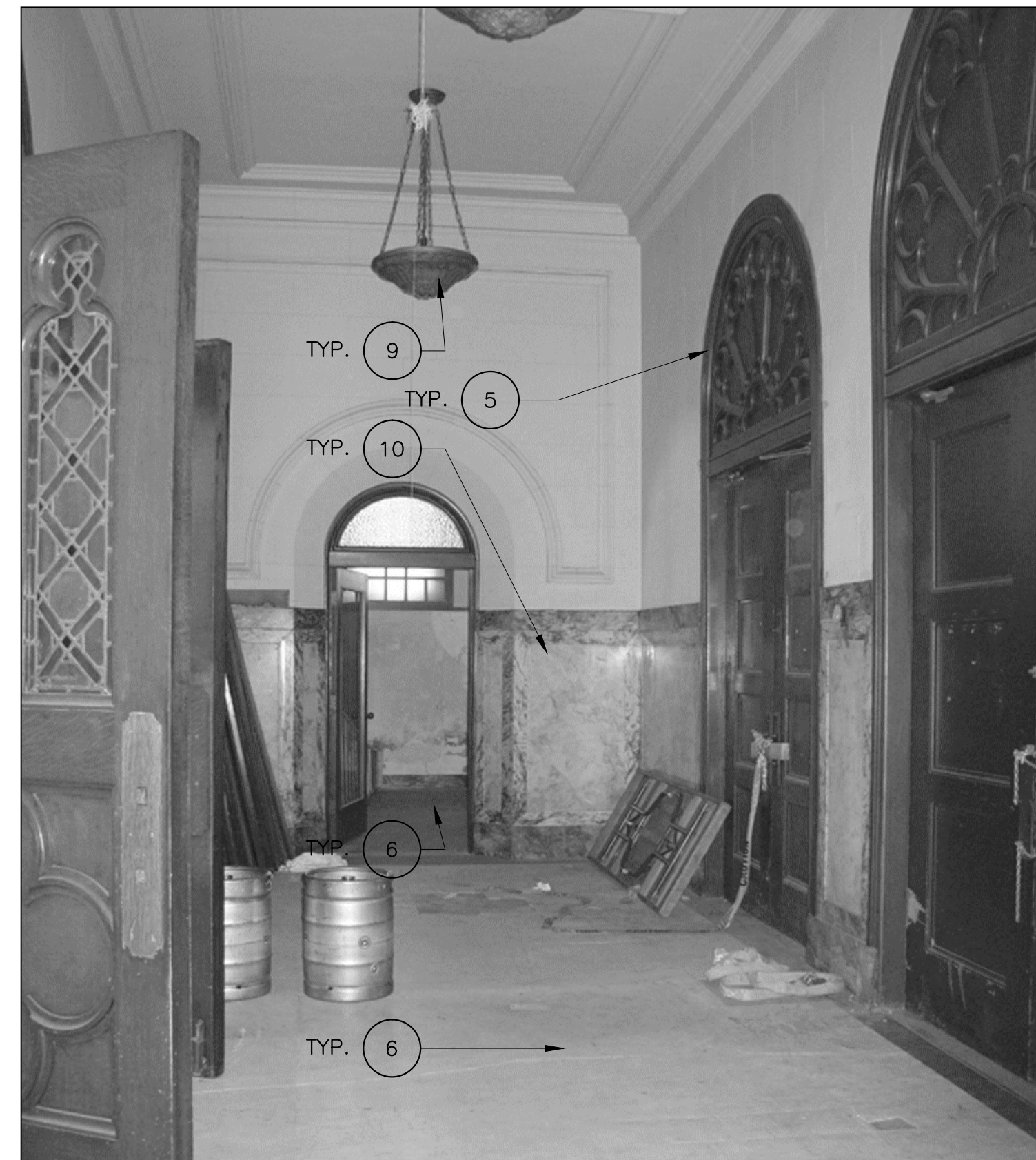
IMAGE F - ENTRY VESTIBULE LOOKING WEST
