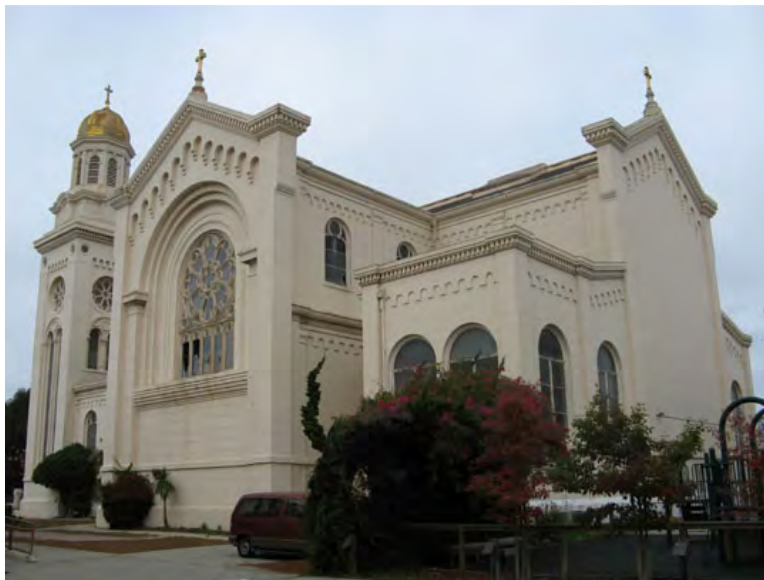
Figure 5. St. Joseph's Church, south and west façades. View north from courtyard. Source: Page & Turnbull, November 2007.
