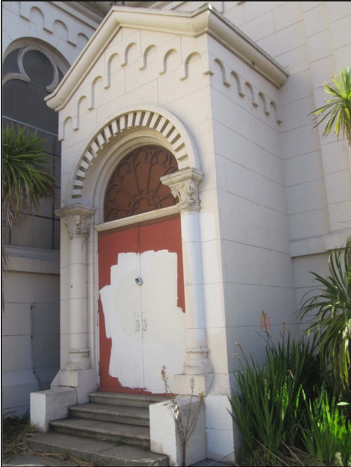
1401 Howard Street, View of Secondary Entrance along West Facade
