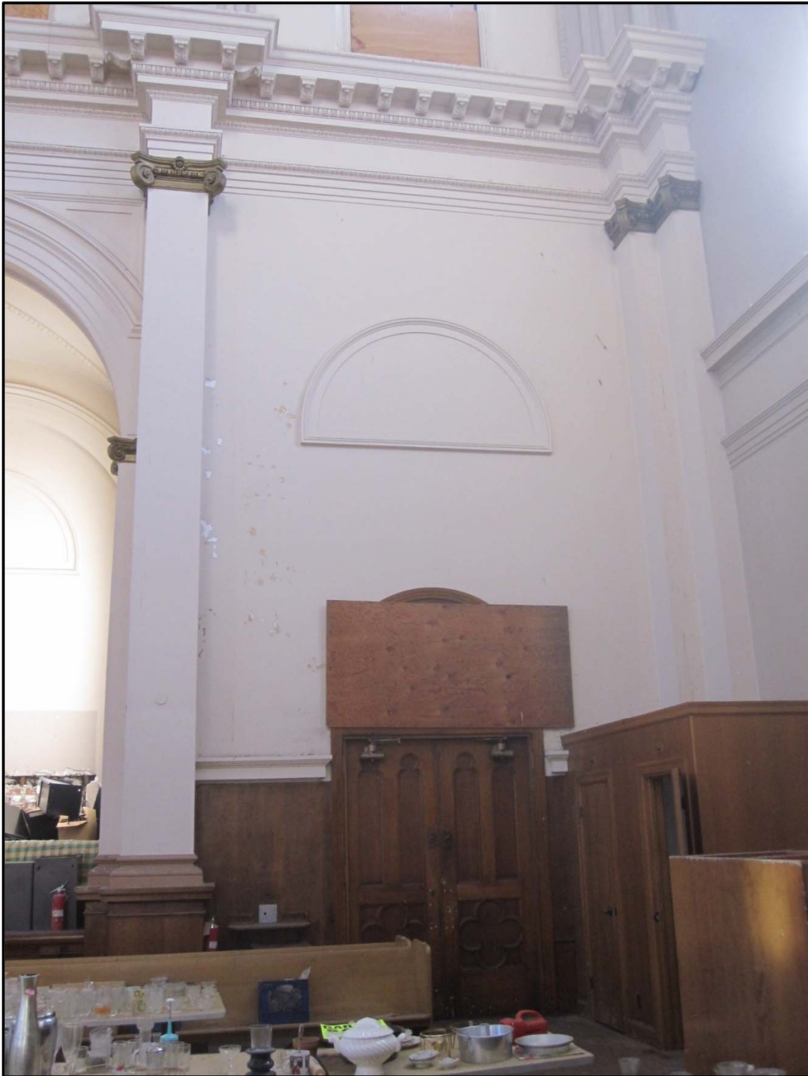
1401 Howard Street, View of Transept Side Wall
