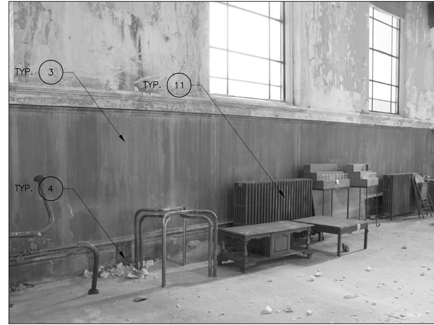
IMAGE E - EAST WALL OF EAST AISLE
