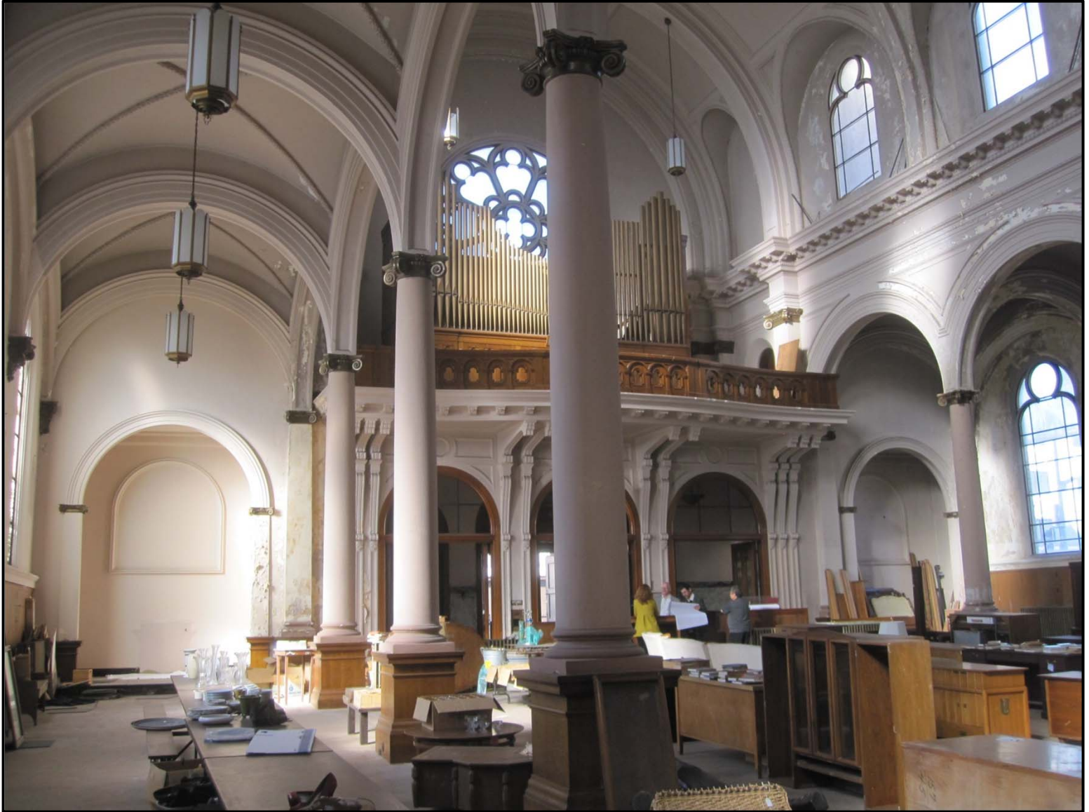
1401 Howard Street, View of Side Aisle looking towards Organ Loft
