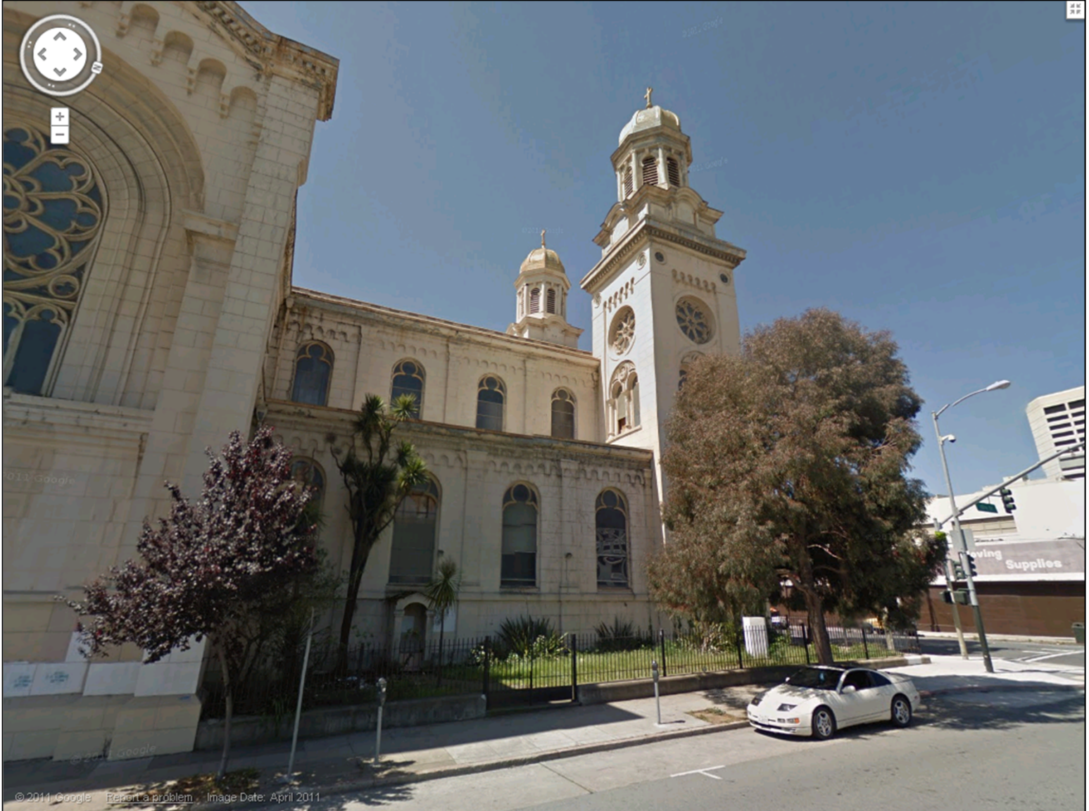
1401 Howard Street, East Façade, View along 10 th Street
