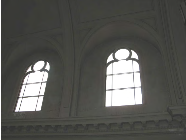
St. Joseph's Church interior. Detail of clerestory windows. Source: Page & Turnbull, November 2007.
