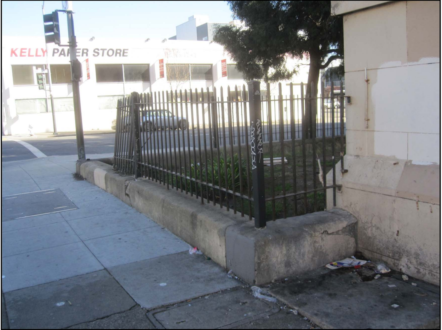
1401 Howard Street, View of fence at corner of 10 th and Howard Streets
