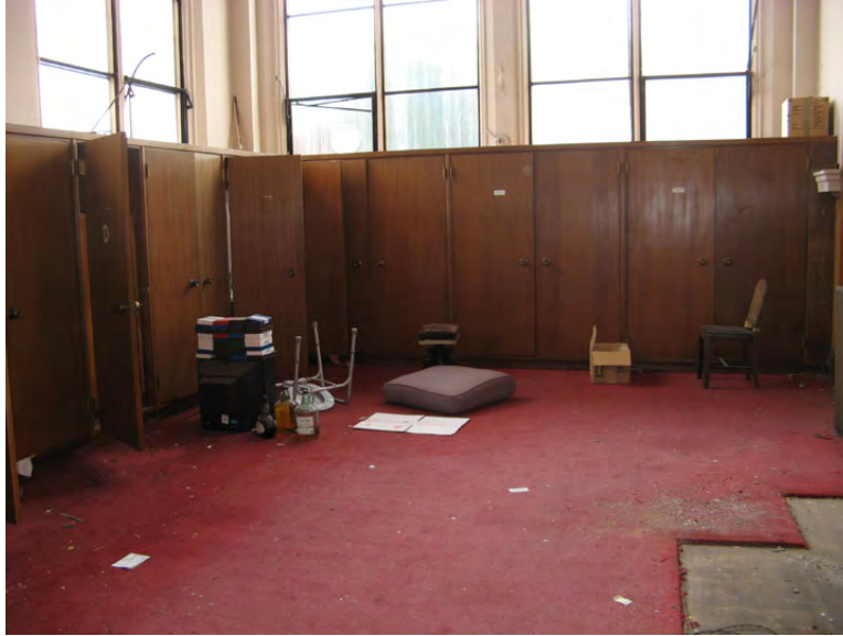
St. Joseph's Church interior. Detail of cabinets in office at southwest corner of church. Source: Page & Turnbull, November 2007.
